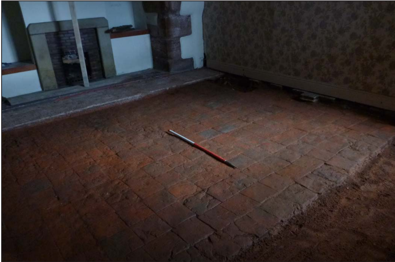
Plate 02: Dining Room showing tiled floor, from the southwest. Scale 1.0m.
