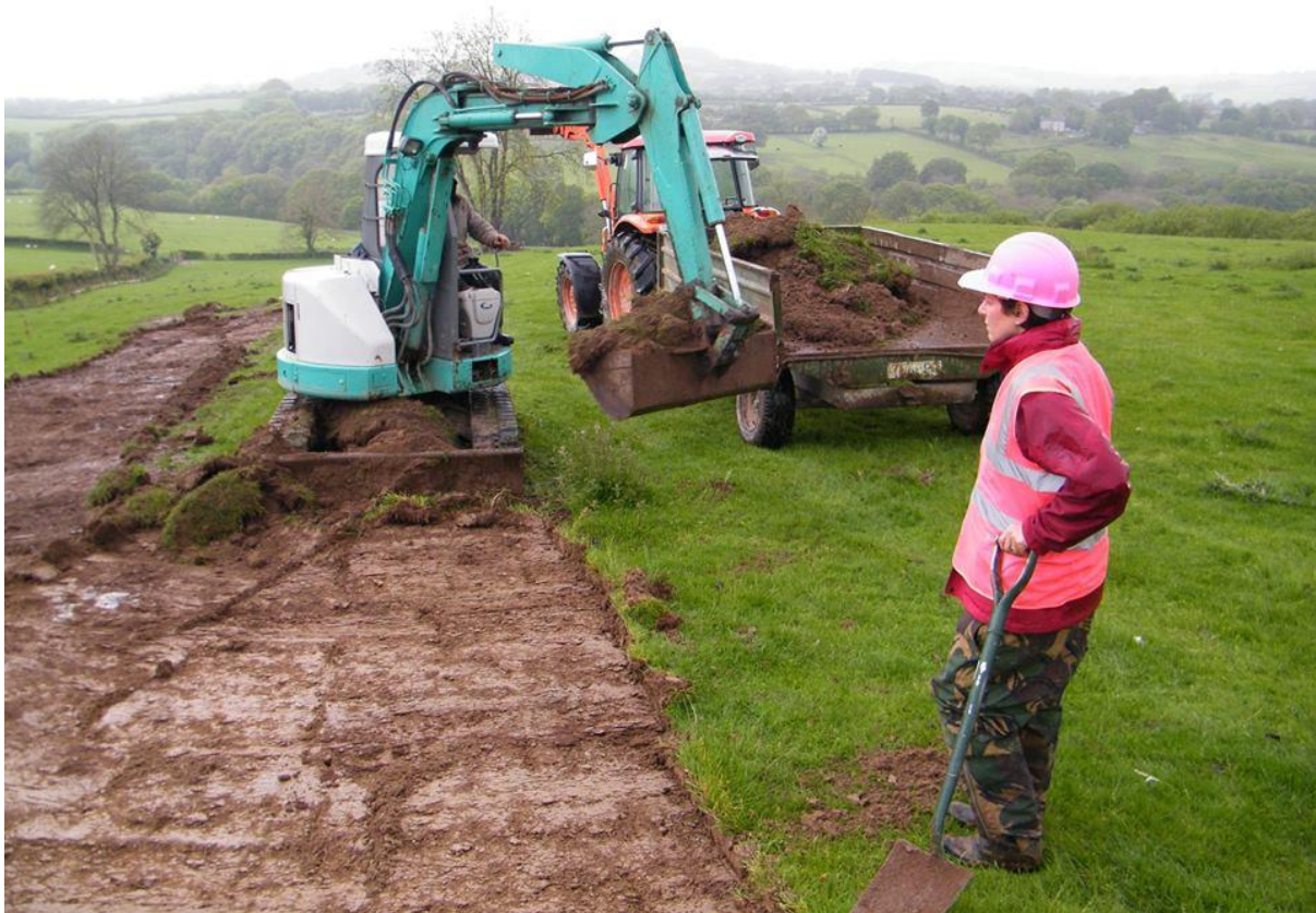
Figure 7: Removing the topsoil.
