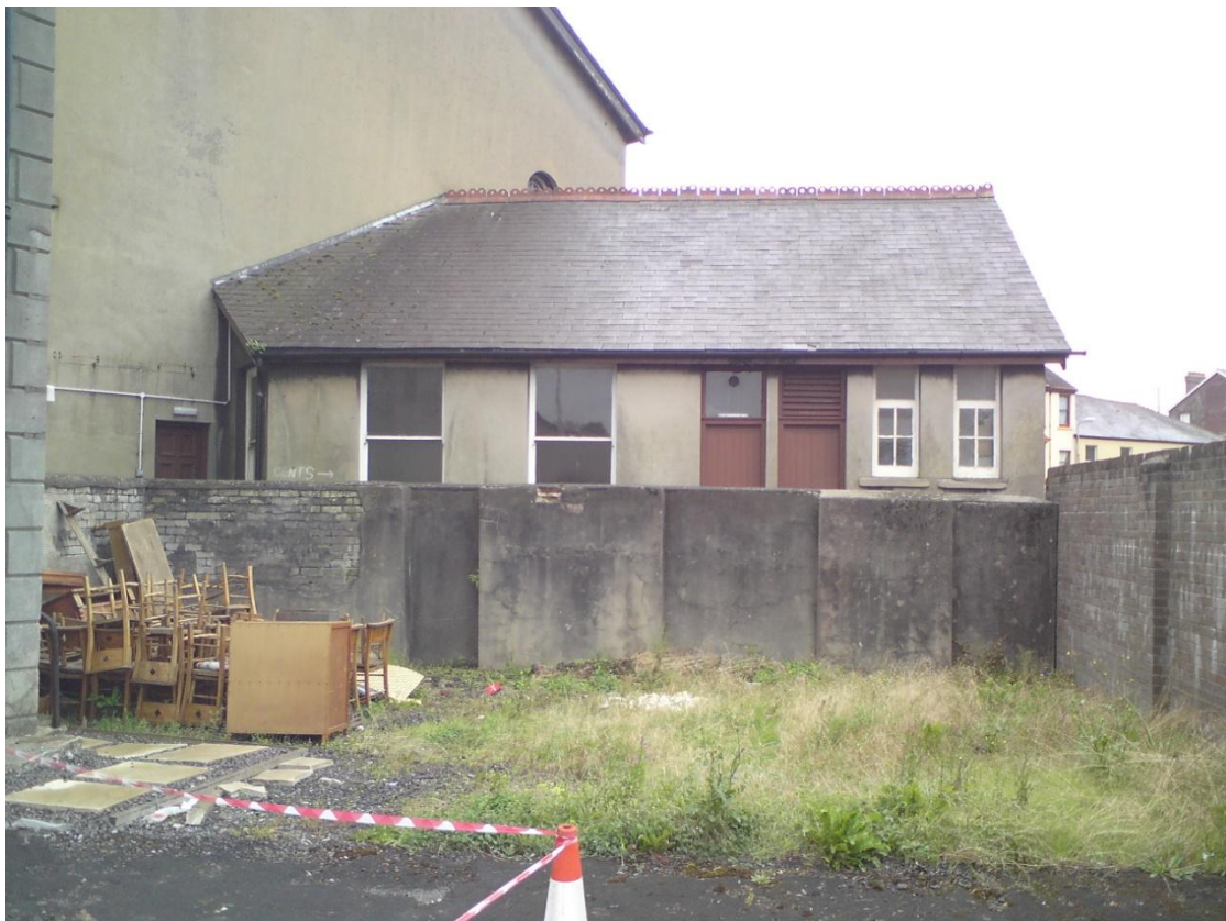
3. Classroom annex, from northeast (rear service yard)
