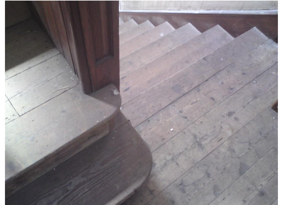
Gallery stair detail, School building
