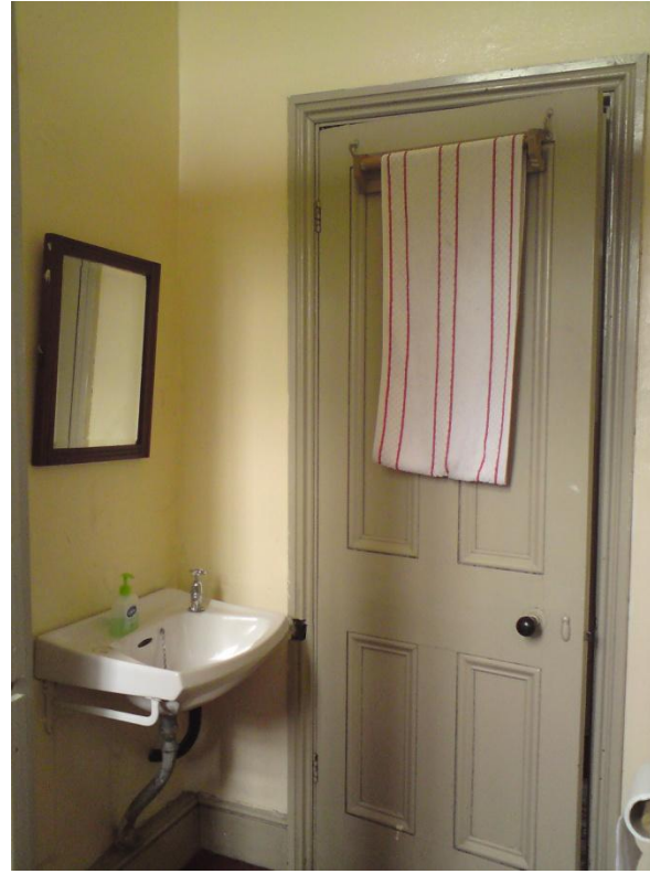
WCs, Classroom annex
