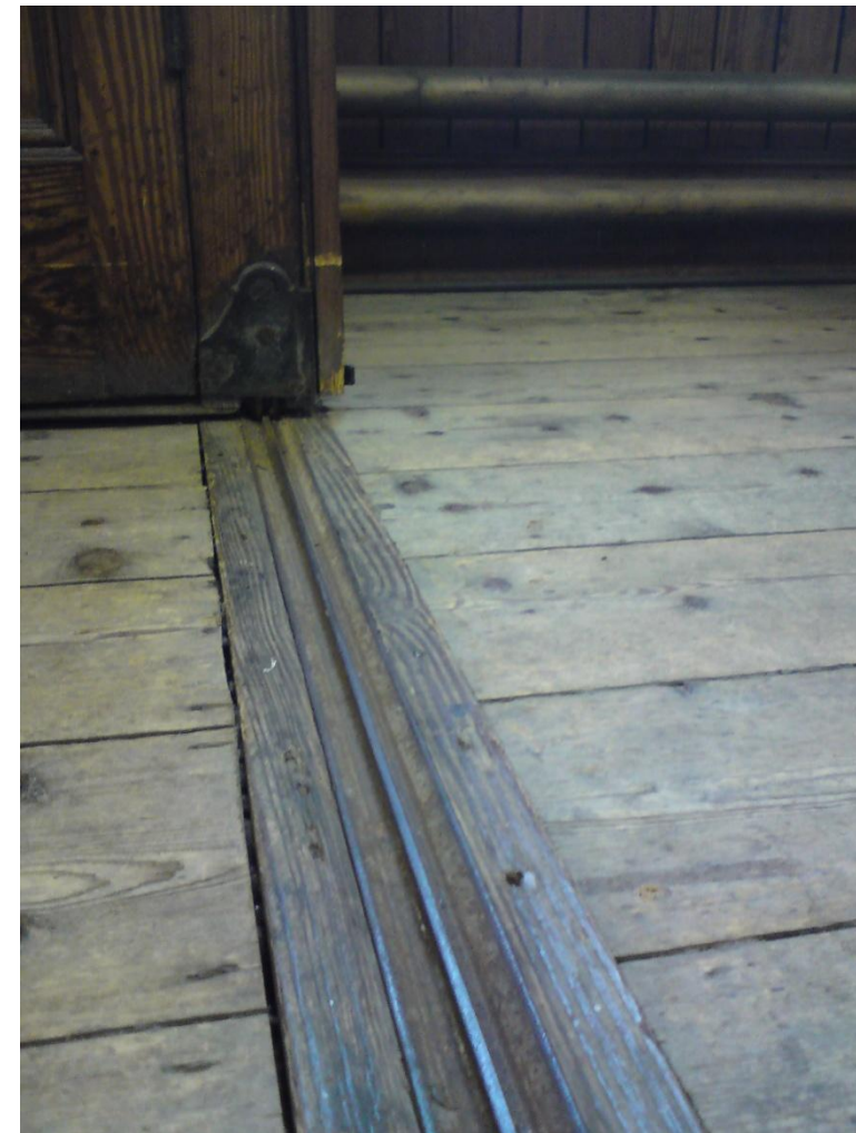
Original Partition Floor Track, Worship Space
