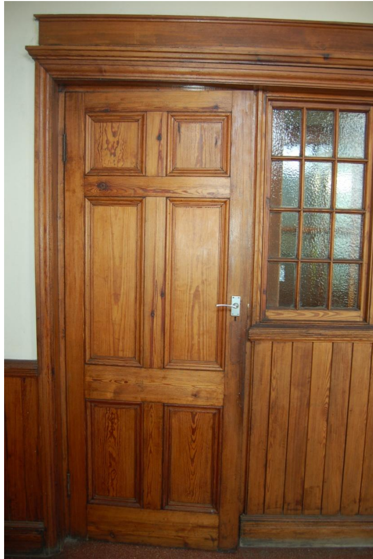
Timber door, School Entrance Lobby
