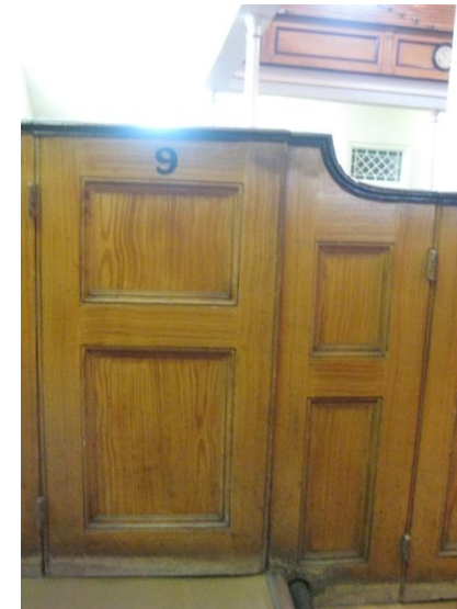
Pew doors, Zion Chapel
