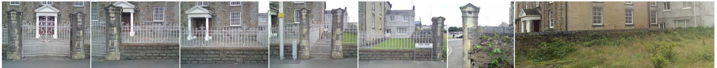
3. Listed perimeter stone wall & iron railings, eastern-most element (Zion Row, beyond), circa 1913
