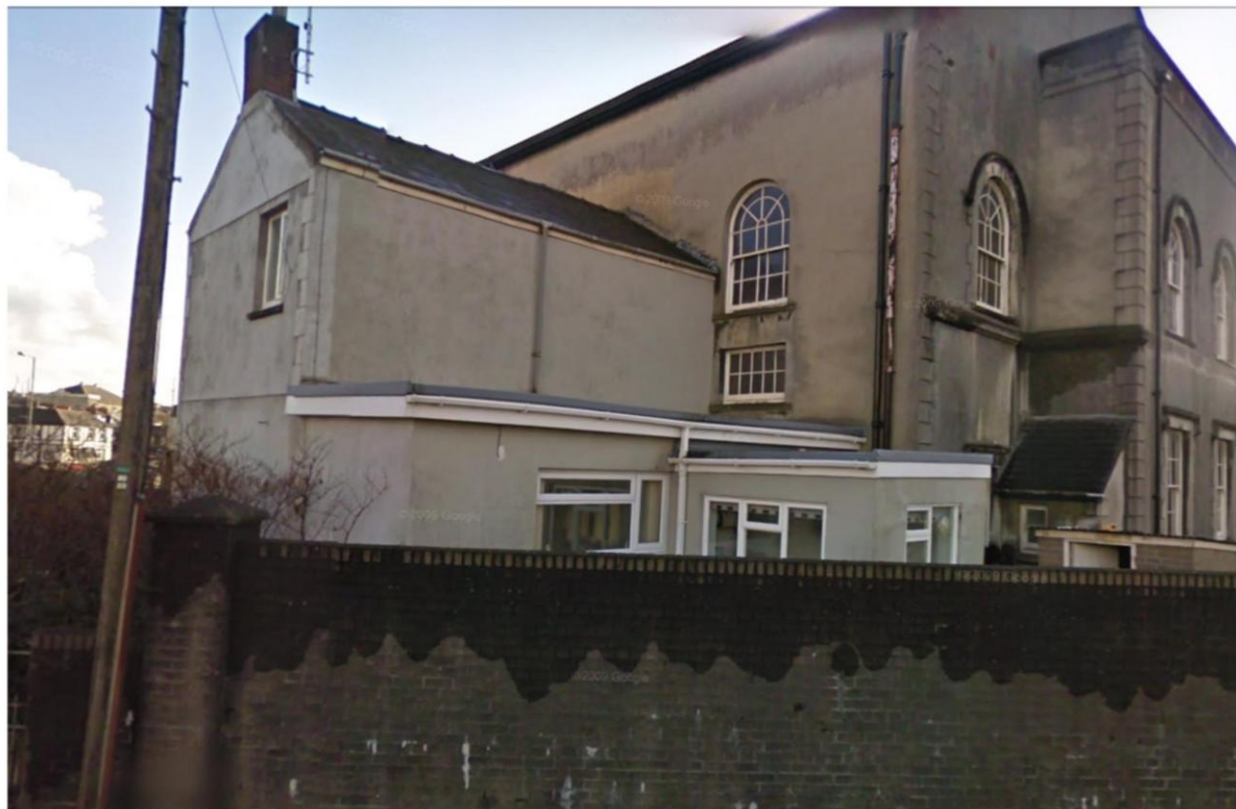
Zion Chapel & Caretaker's House from northeast
