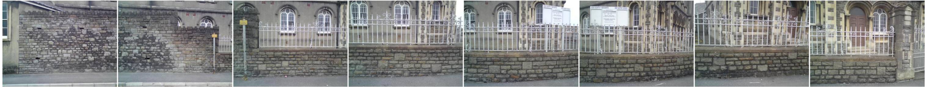
1. Listed perimeter stone wall & iron railings, south-western element (Water Street), circa 1913
