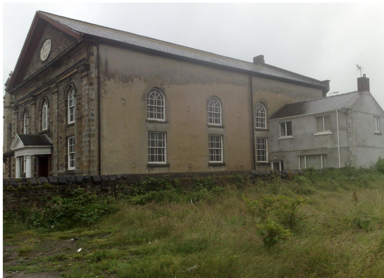
Zion Chapel & Caretaker's House from southeast
