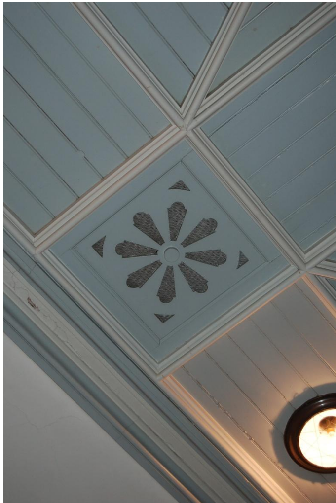
Ceiling plaster/joinery detail, Zion Chapel
