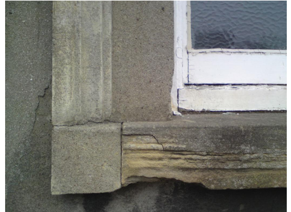
1c. Stucco window detail, Classroom annex
