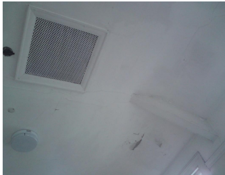
Classroom ceiling, Classroom annex
