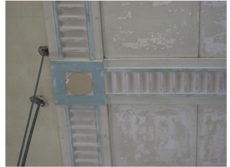
Original plaster ceiling detail, School building
