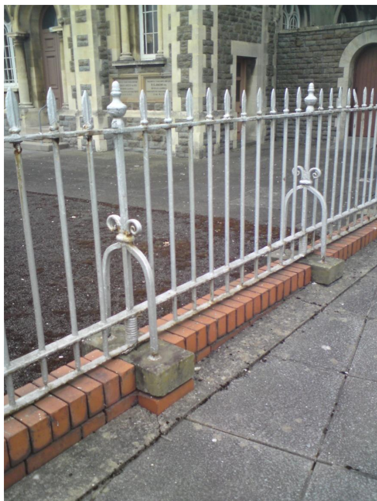
Wrought iron railings between Chapel & School
