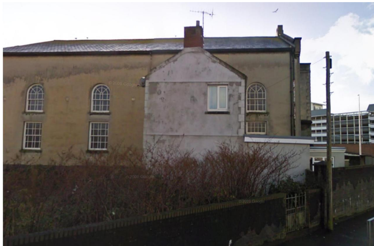
Zion Chapel & Caretaker's House from east
