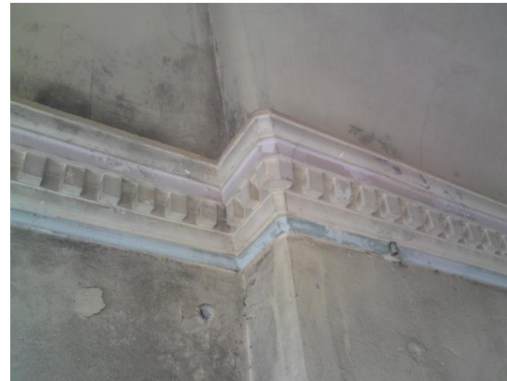
Gallery level wall plaster mouldings, School building
