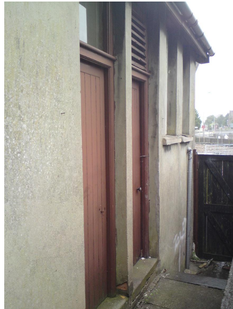
2b. Corridor & WC doors, Classroom annex
