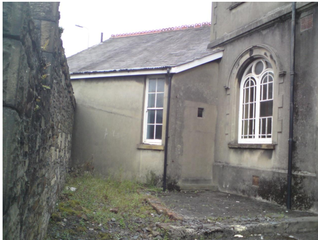
4. Classroom annex, from south (Water Street/entrance forecourt)
