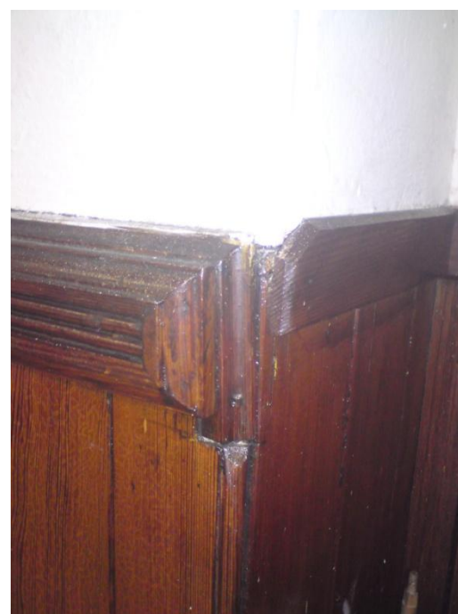
Typical partition recess/dado joinery
