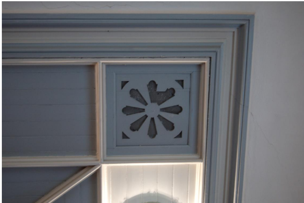
Ceiling plaster/joinery detail with small vent, Zion Chapel
