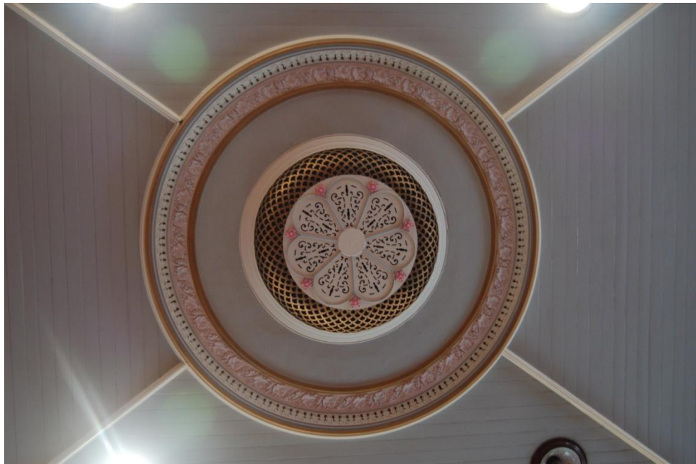
Central plaster/timber/brass roof vent, Zion Chapel
