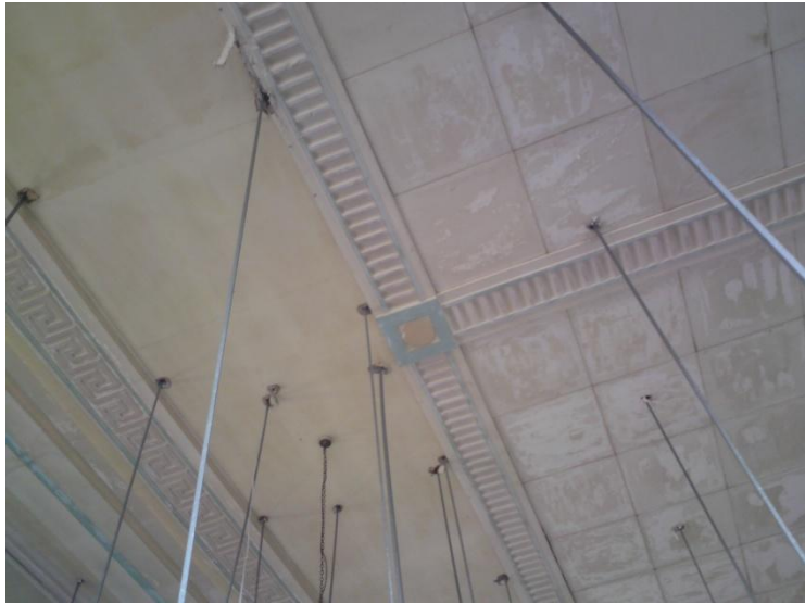
Original plaster ceiling, School building
