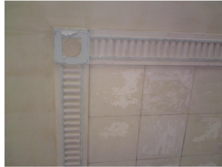
Original plaster ceiling detail, School building
