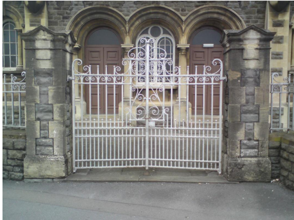
1. Gates & gate piers to Zion Baptist School
