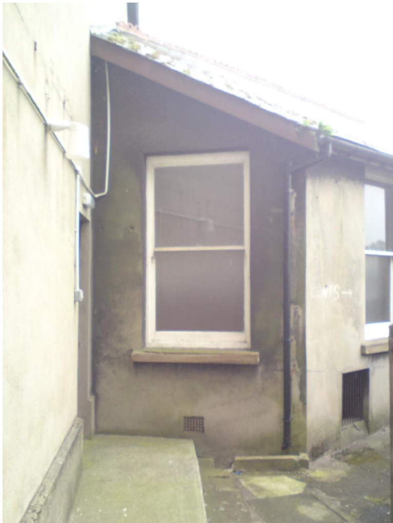
2a. Classroom sash window, Classroom annex
