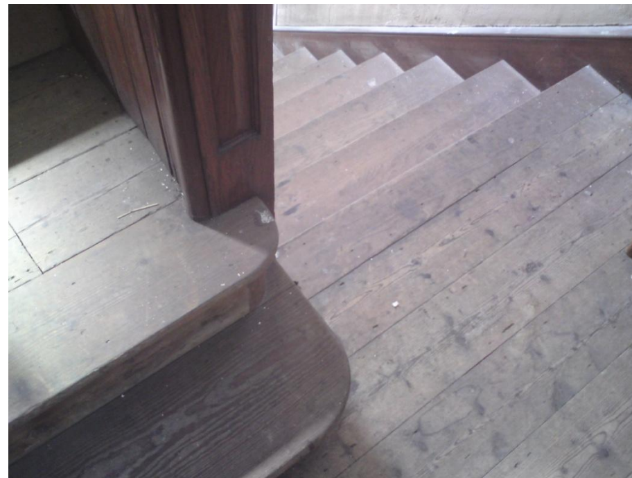
Gallery joinery detail, School building
