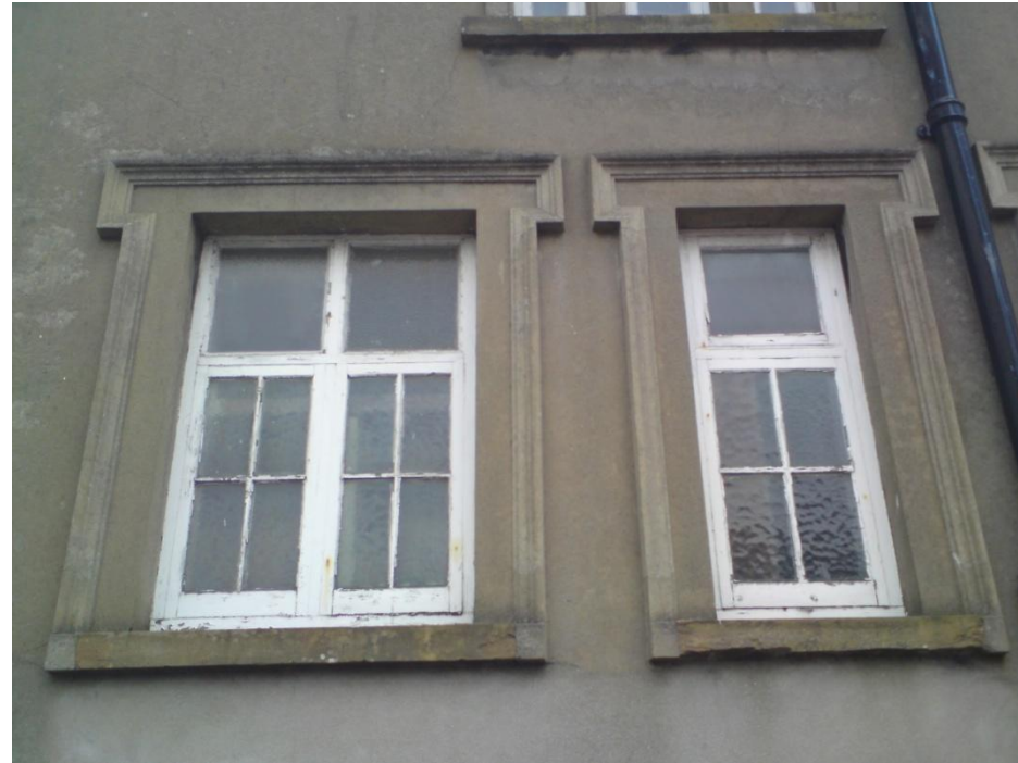
1b. Kitchen/WC stucco feature windows, Classroom annex
