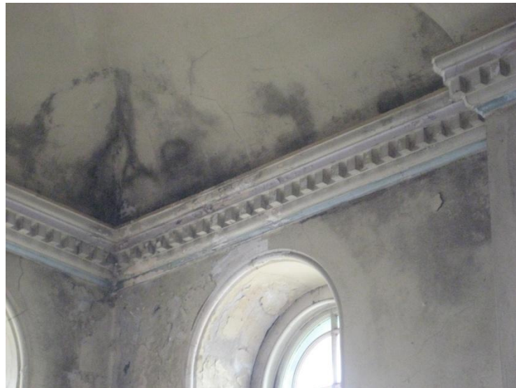
Gallery level wall plaster mouldings, School building
