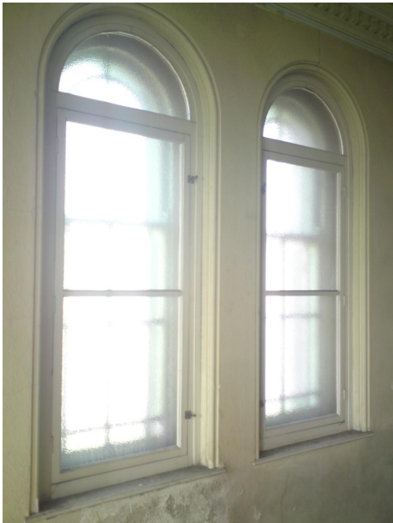
Secondary Glazing (west), School building
