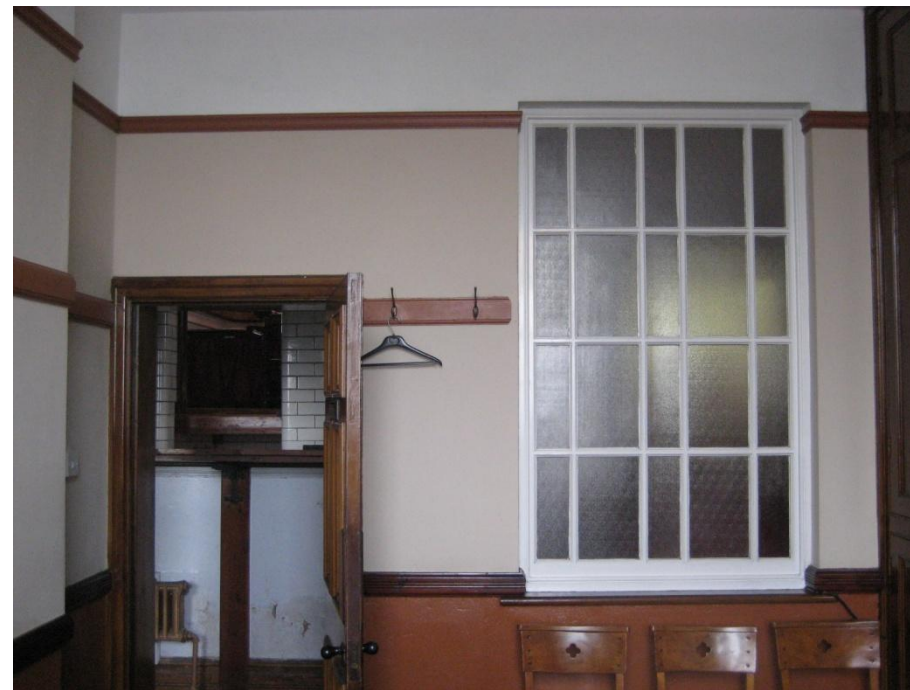
Deacons' Room interior (south), Zion Chapel
