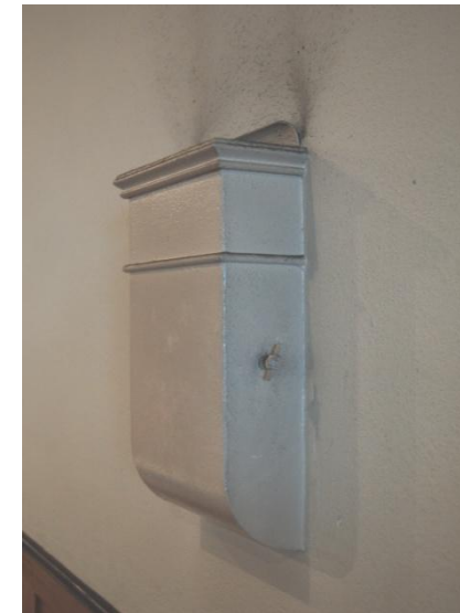
Wall vent, Zion Chapel
