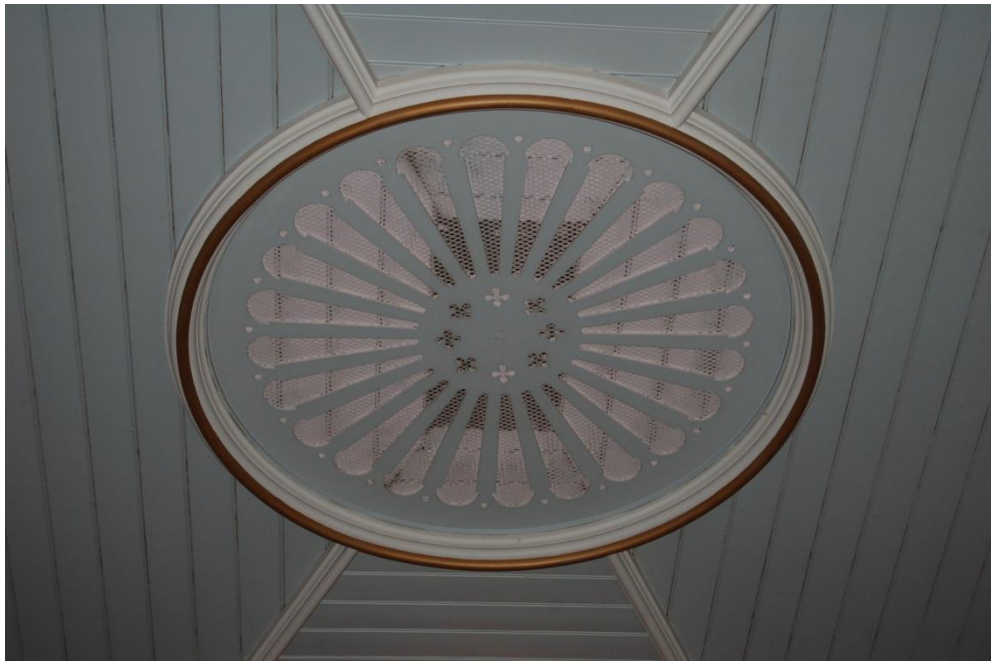
Plaster/timber roof vent, Zion Chapel
