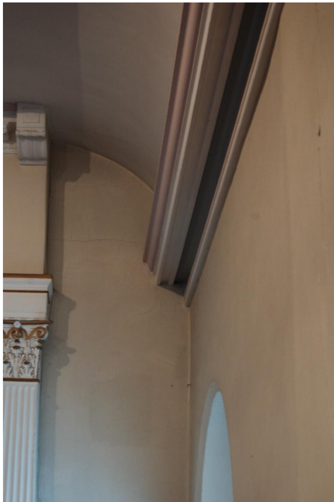
Ceiling level plaster details, Zion Chapel
