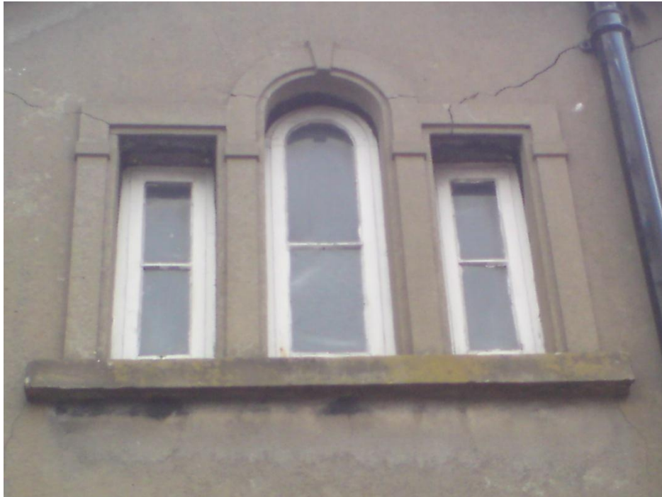
1a. Loft level stucco feature window, Classroom annex
