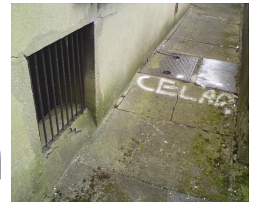
2d. Cellar access, annex
