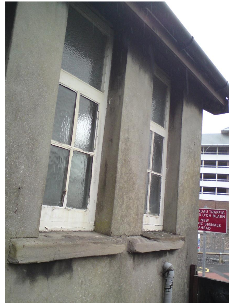
2c. WC Windows, Classroom annex
