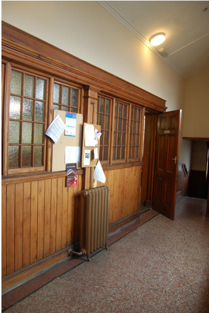
Timber/glazed screen, School Entrance Lobby
