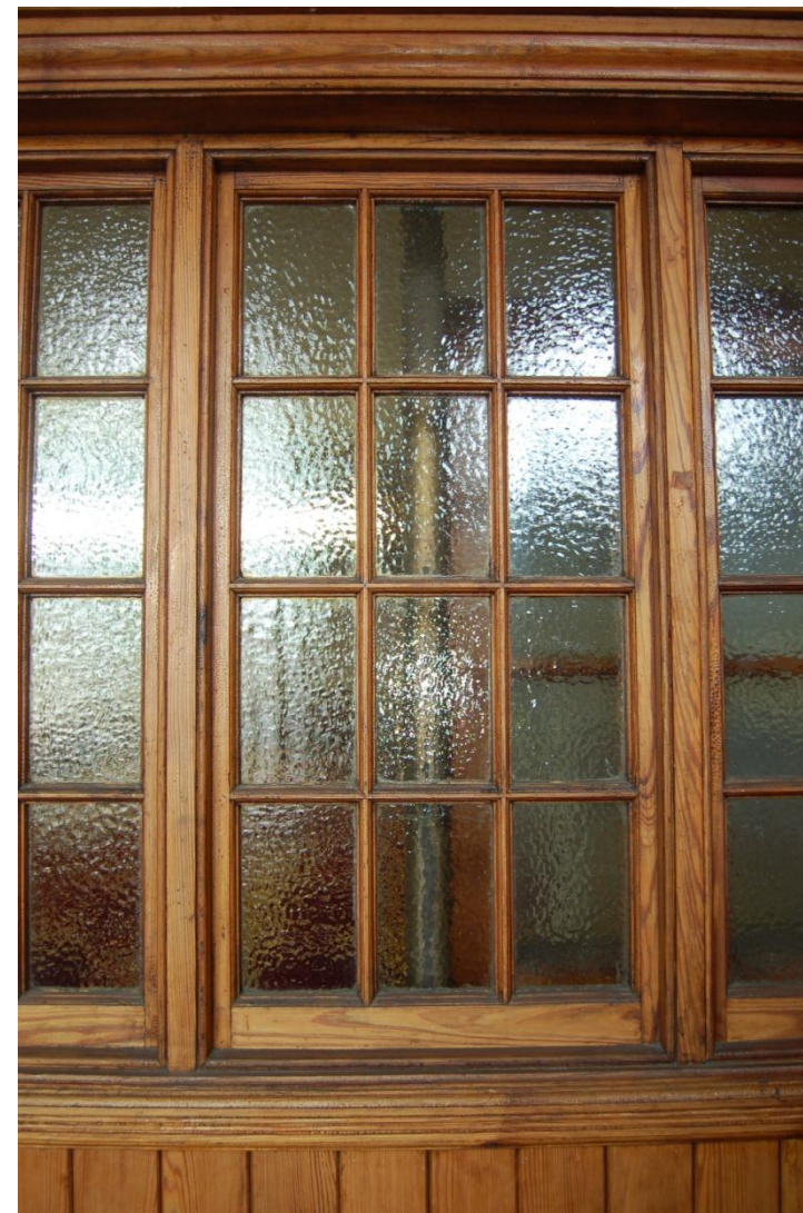
Glazed panel, School Entrance Lobby
