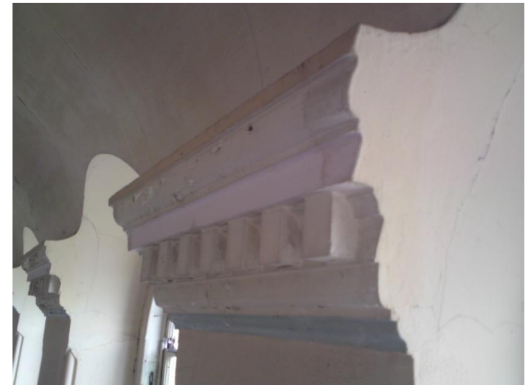
Gallery level wall plaster mouldings, School building
