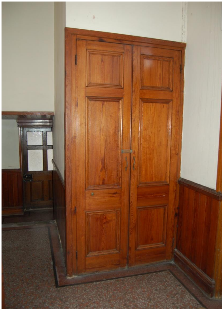
Gallery stair lobby doors (east), School building
