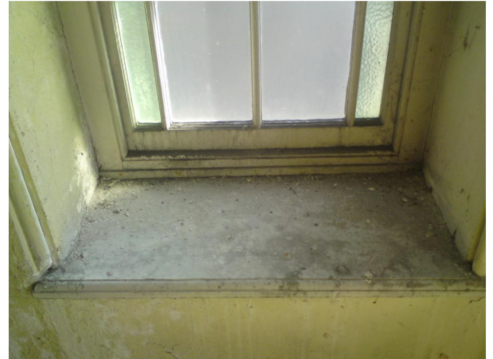
Gallery level window sill detail, School building
