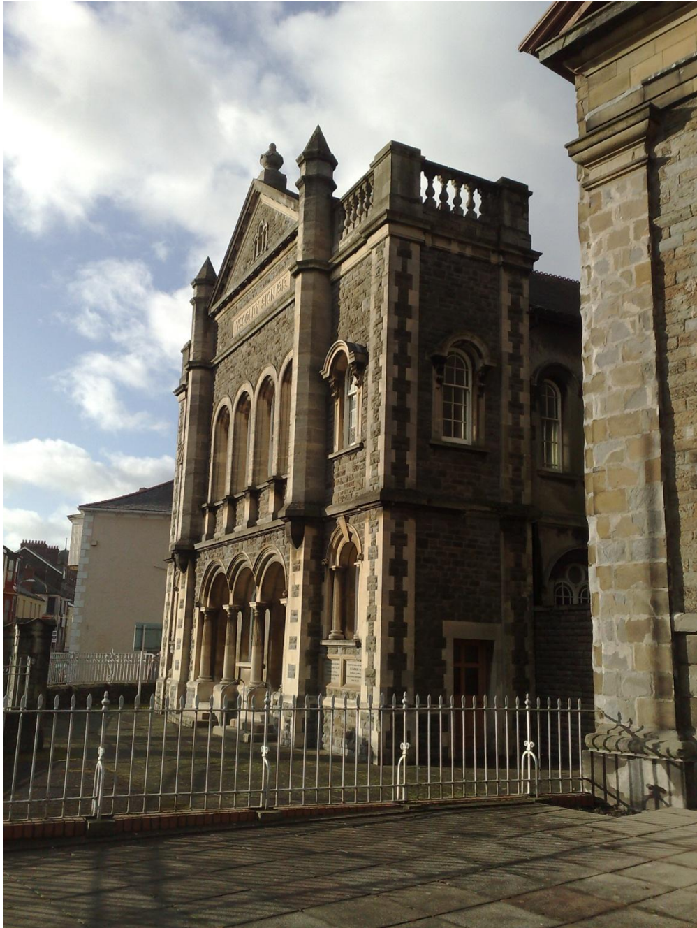
1. Southern (entrance) facade of School Building (1913)
