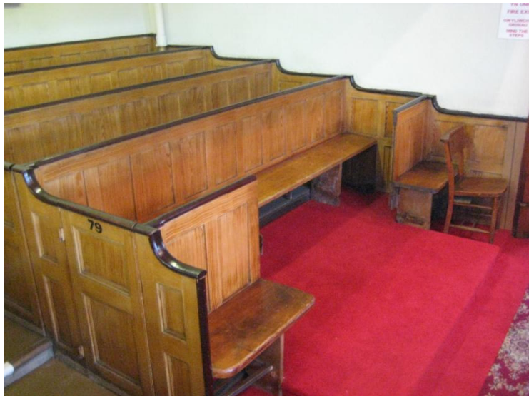
Ground level pew alteration, Zion Chapel
