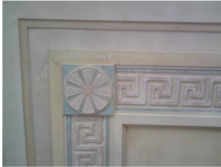
Original plaster ceiling detail, School building
