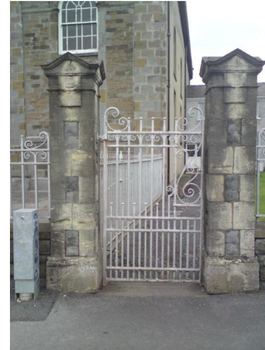
3. Gates & gate piers to Caretakers' House
