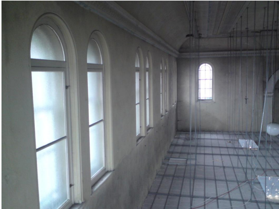
Gallery level window vista, School building
