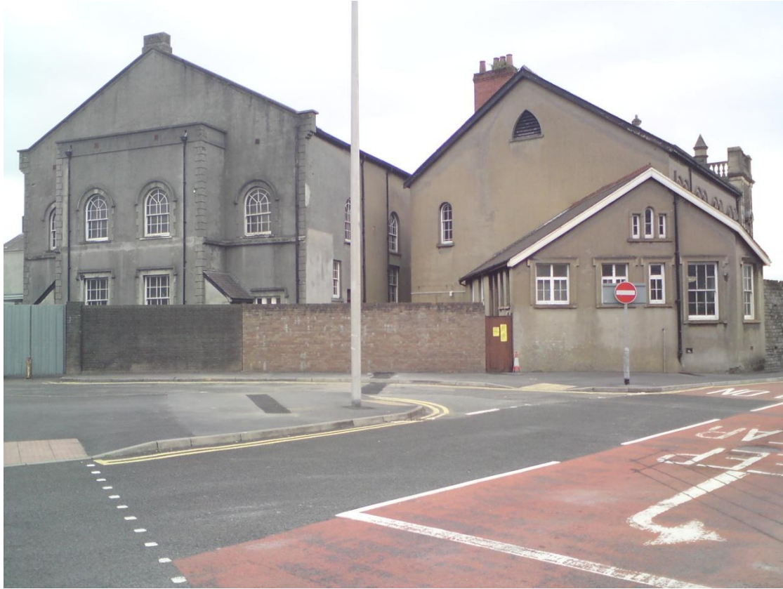
1. Zion Chapel, School and Classroom annex, from northwest (A484)
