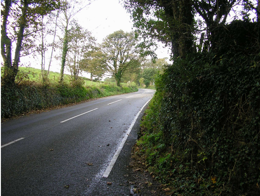
Plate C – Visibility in Leading Direction from Existing Site Access
