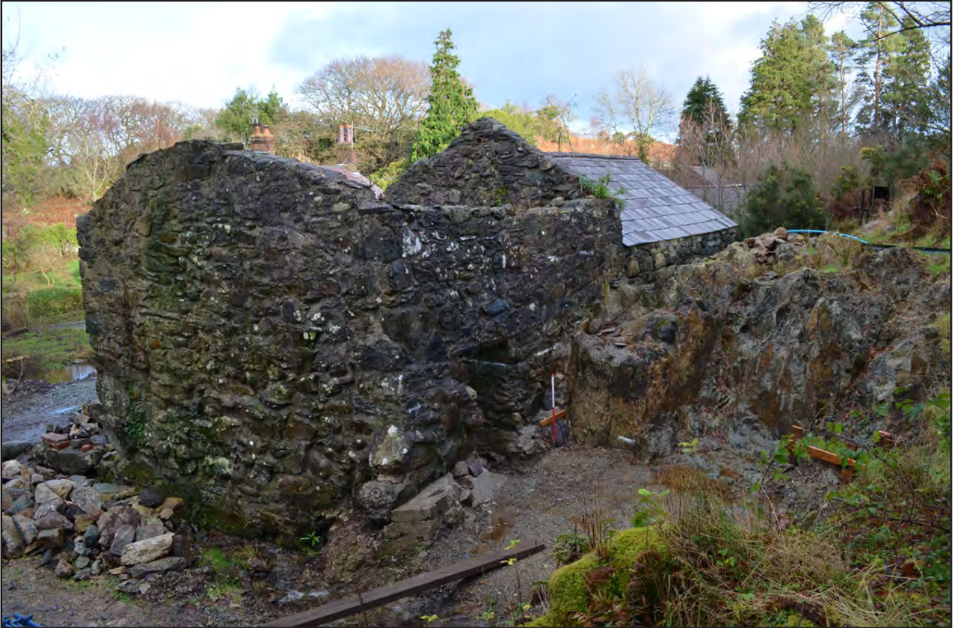
Plate 09: General view from the south (Scale: 1 x 1.0m)
