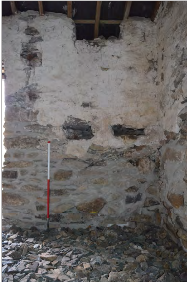
Plate 14: Northeast room - southeast-facing internal elevation (Scale: 1 x 1.0m)
