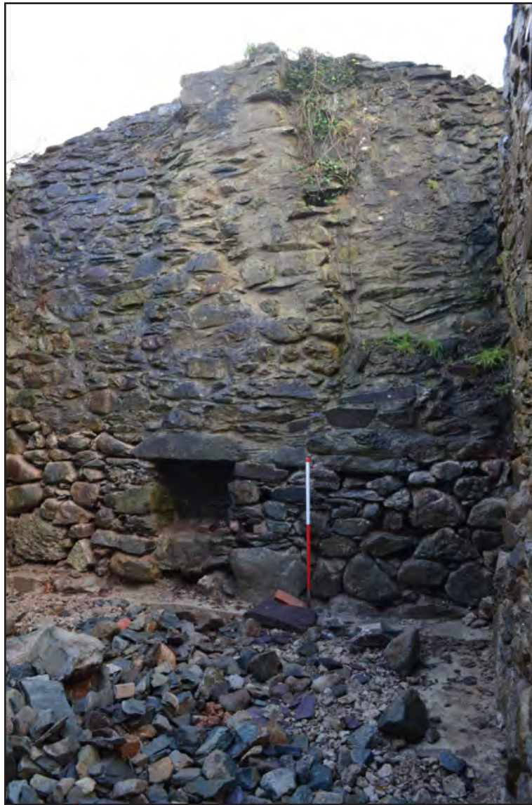
Plate 15: Southwest room - internal elevation: fireplace in the gable wall (Scale: 1 x 1.0m)
