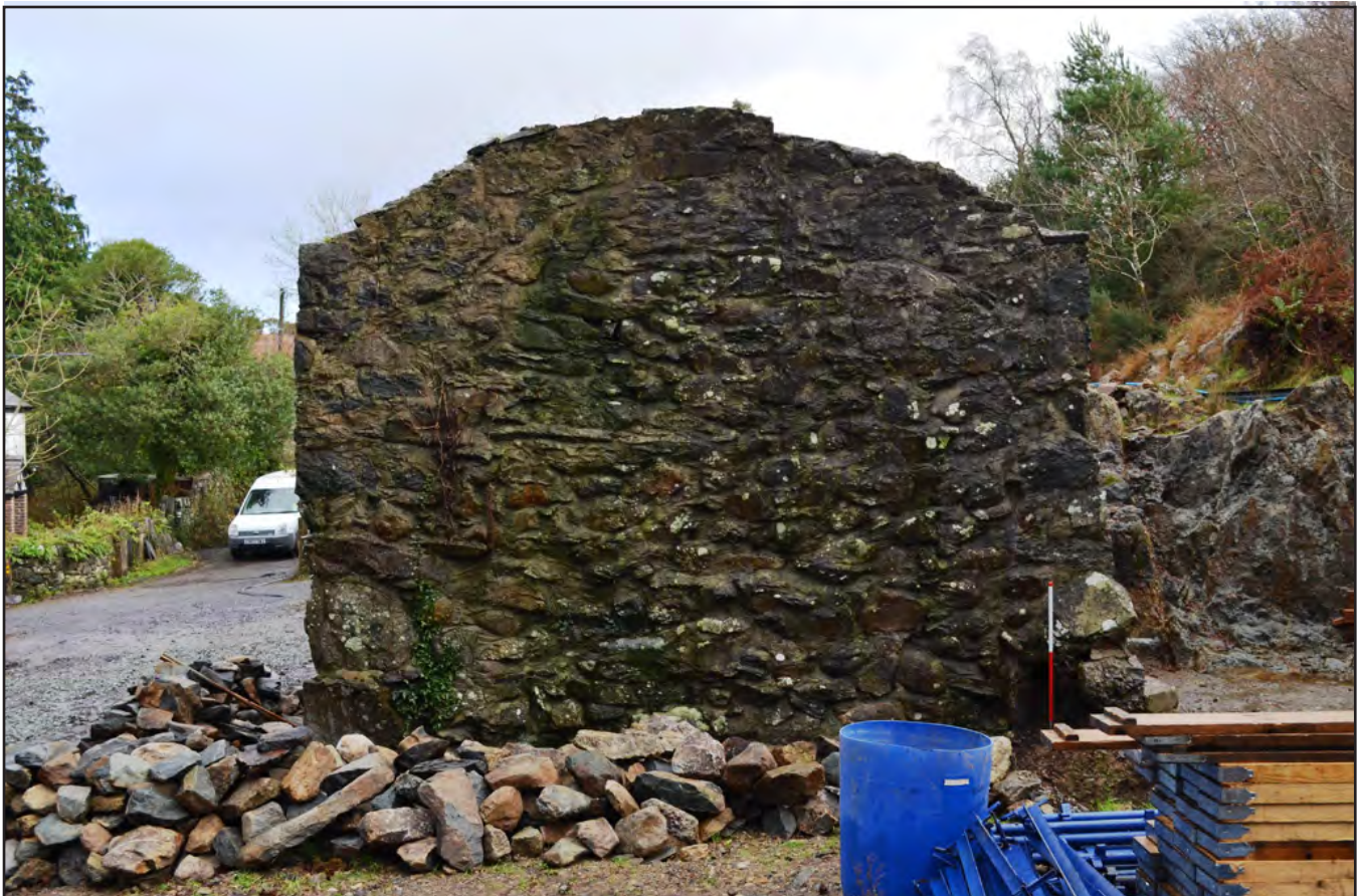
Plate 10: Southwest elevation (Scale: 1 x 1.0m)
