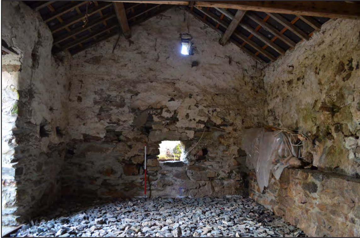
Plate 13: Northeast room – southwest-facing internal elevation (Scale: 1 x 1.0m)
