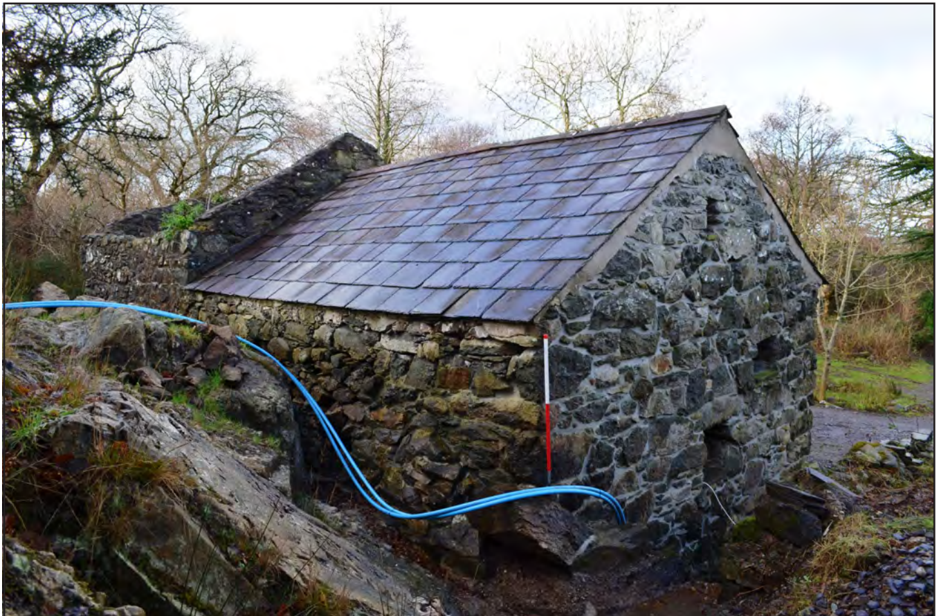
Plate 04: Oblique view of northeast gable (Scale: 1 x 1.0m)
