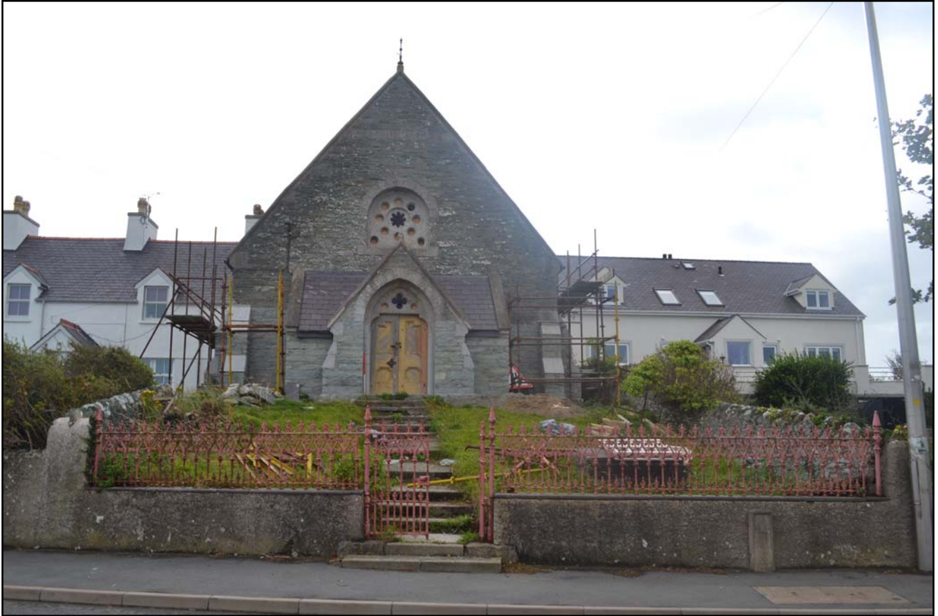
Plate 01: Capel Horeb external northwest elevation. Photograph taken from the northwest.
