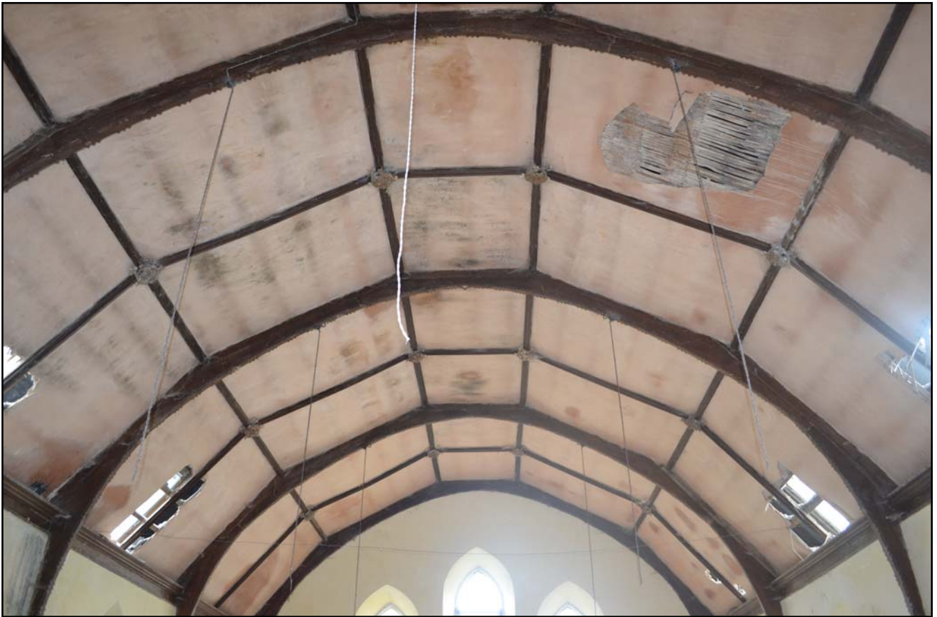
Plate 09: Capel Horeb plaster wagon ceiling. Photograph taken from the northwest.
