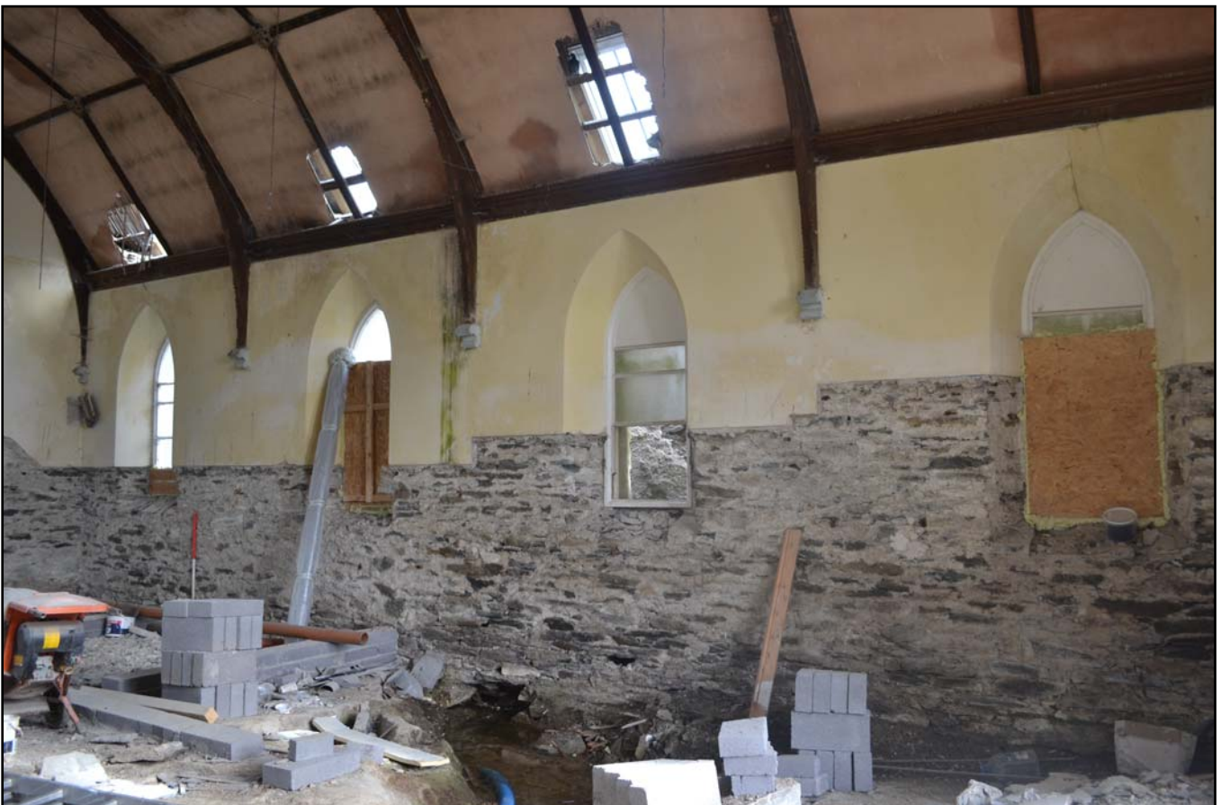
Plate 08: Capel Horeb internal northeast elevation. Photograph taken from the south.
