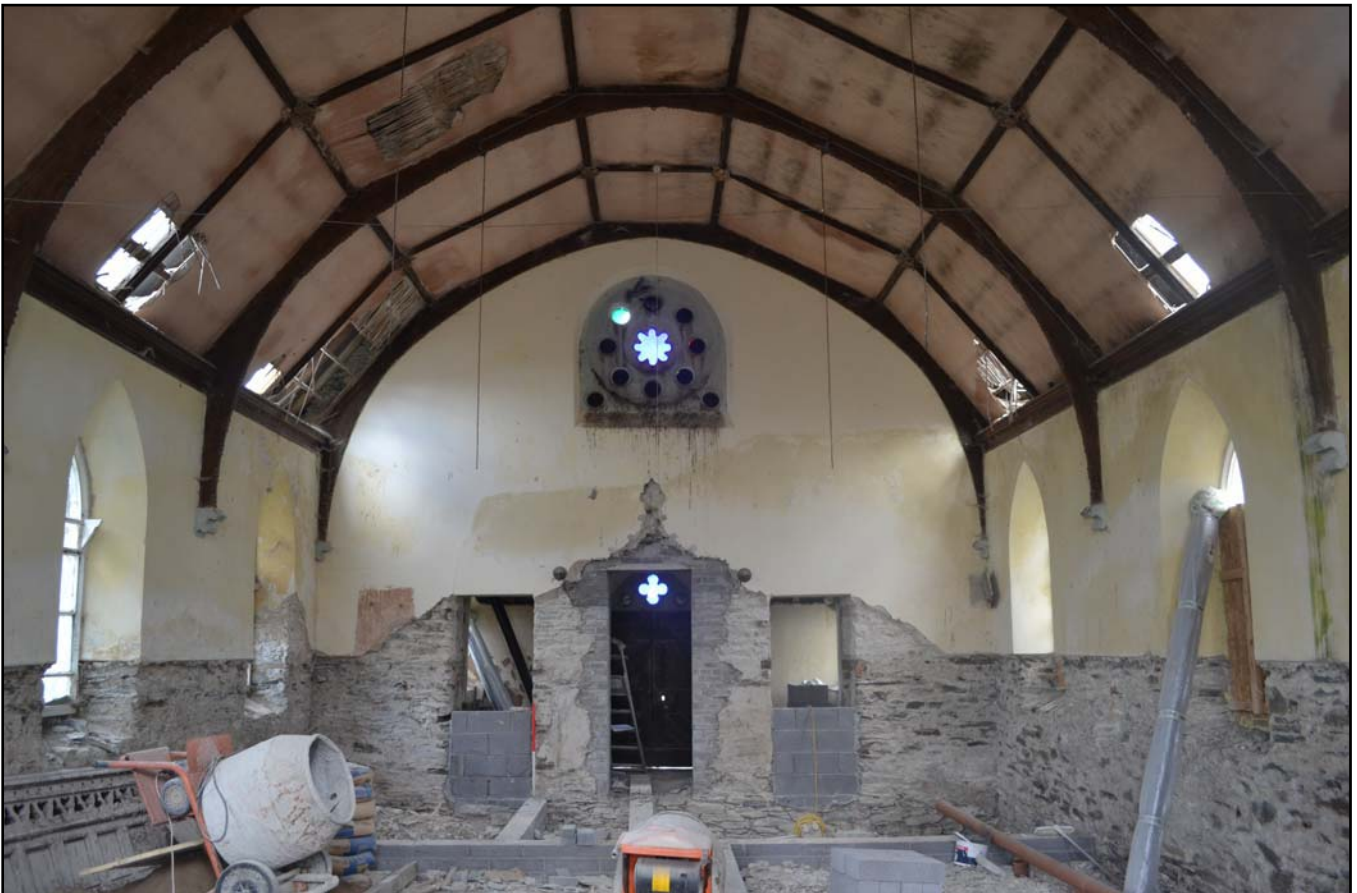
Plate 06: Capel Horeb internal northwest elevation. Photograph taken from the southeast.
