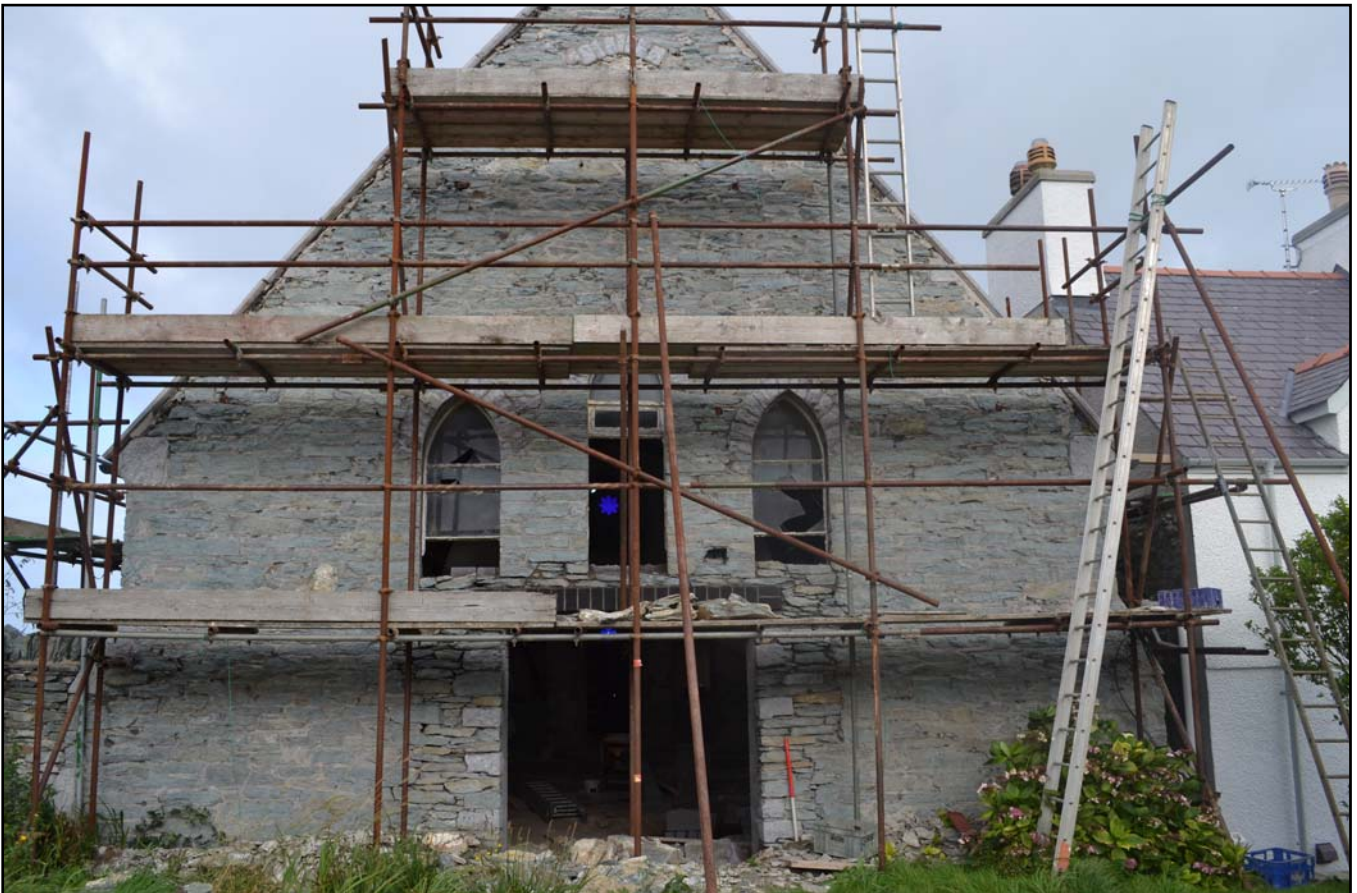
Plate 04: Capel Horeb external southeast elevation. Photograph taken from the southeast.
