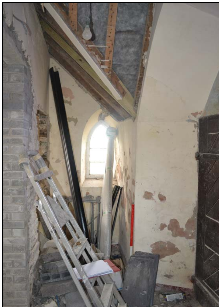
Plate 12: Capel Horeb narthex internal southwest elevation. Photograph taken from the northeast.
