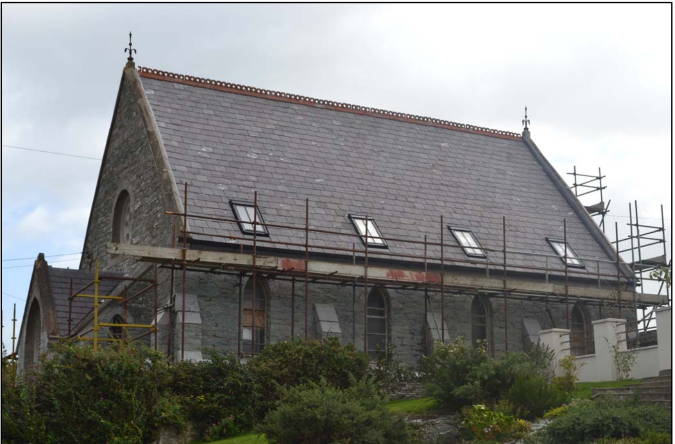
Plate 02: Capel Horeb external southwest elevation. Photograph taken from the west.
