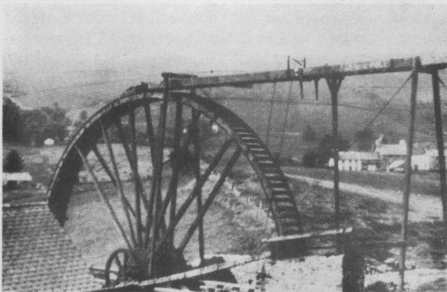
Figure 2. A close up view of the 50 foot waterwheel taken by Mr D.L. Dixon in 1932. In the launder, the trap door to discharge the water is visible with control wires still affixed but the chute below the launder, into the shaft, has rotted away. The large gear fixed to the axle, engaged onto a pinion on the 16 HP. steam engine housed on the first floor, above the boiler. The sweep rod is also particularly apparent. This was connected to a bogie which ran on rails fixed to the masonry pier, now demolished as it was in danger of falling into the cafn shaft which was located behind it. The hamlet of Llywernog is visible in the background.
