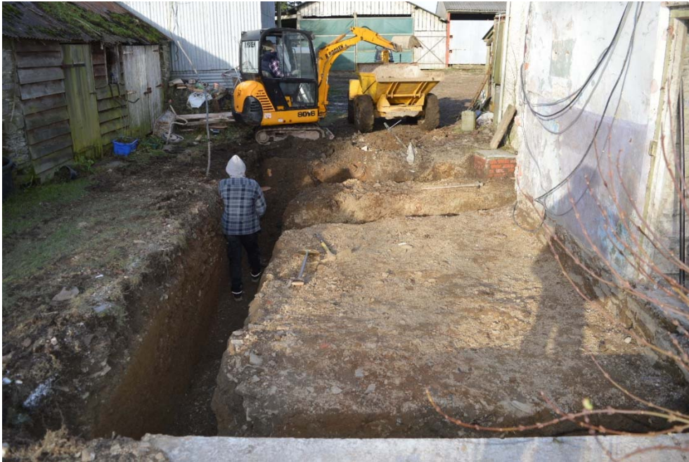
Fig. 5 General view of the foundation trenches. Photo CPAT 4287-0002
