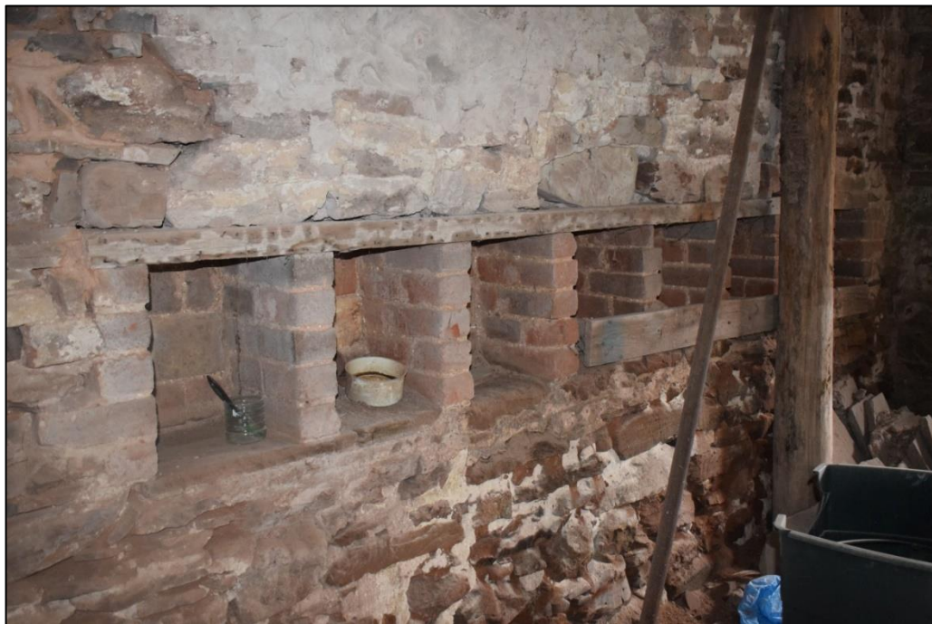
Fig. 12 Bee boles in the north-east elevation Photo CPAT 4691-28
