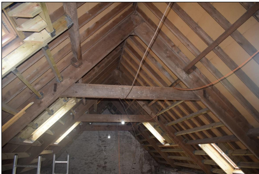
Fig. 14 Roof frame viewed from the south-west Photo CPAT 4691-57
