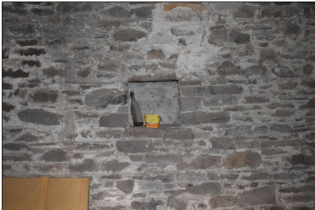
Fig. 10 Niche in north-west elevation Photo CPAT 4691-29
