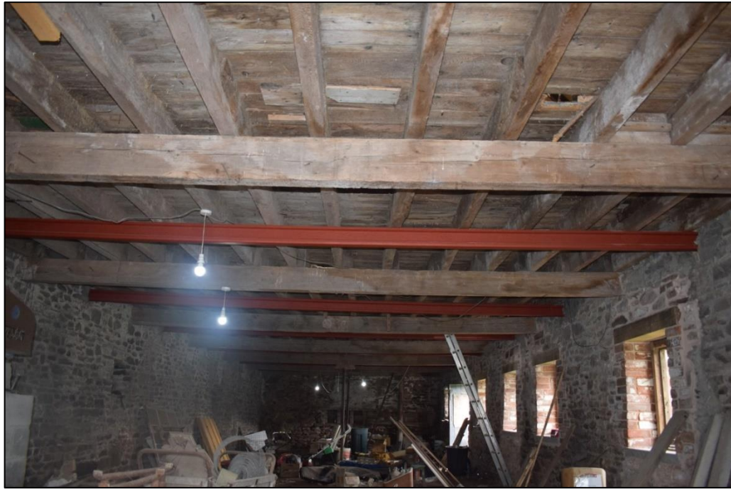
Fig. 9 Ground floor of the granary, viewed from the south-west Photo CPAT 4691-38
