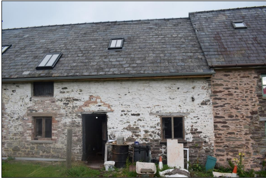
Fig. 7 Original doorway and mullion window in the south-east elevation Photo CPAT 4691-13
