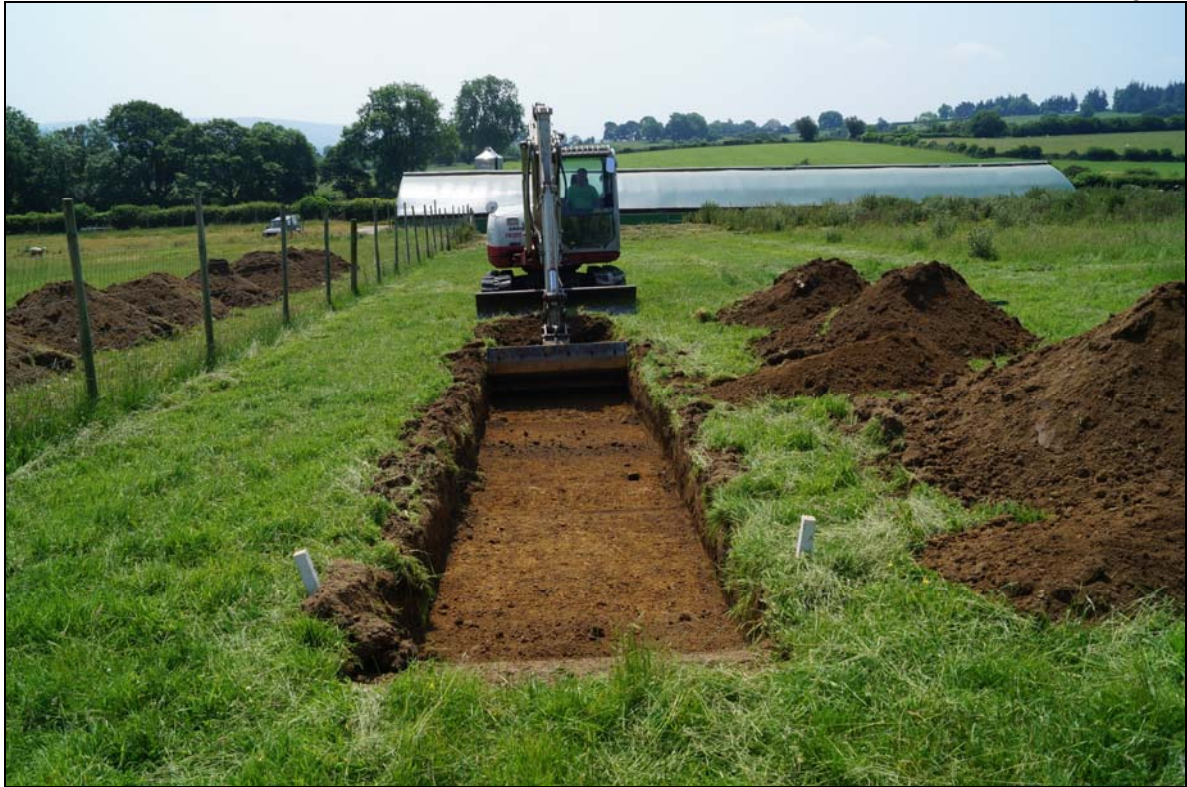
Plate 11: BCF2017_210. Trench E, looking south-southeast
