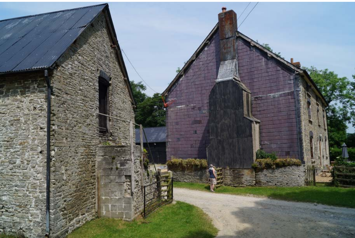
Plate 8: The view east-northeast towards Bache farmhouse, showing the slate-clad western gable wall. The southern end of the western farmyard range is seen in the foreground to the left.
