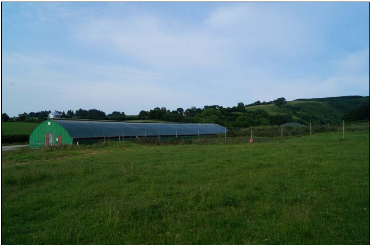
Plate 2: BCF2017_201. View of existing mobile poultry sheds, looking southwest.
