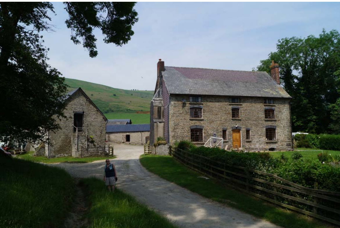
Plate 14: A view looking north at the front of Bache farmhouse and the entrance into the farmyard.
