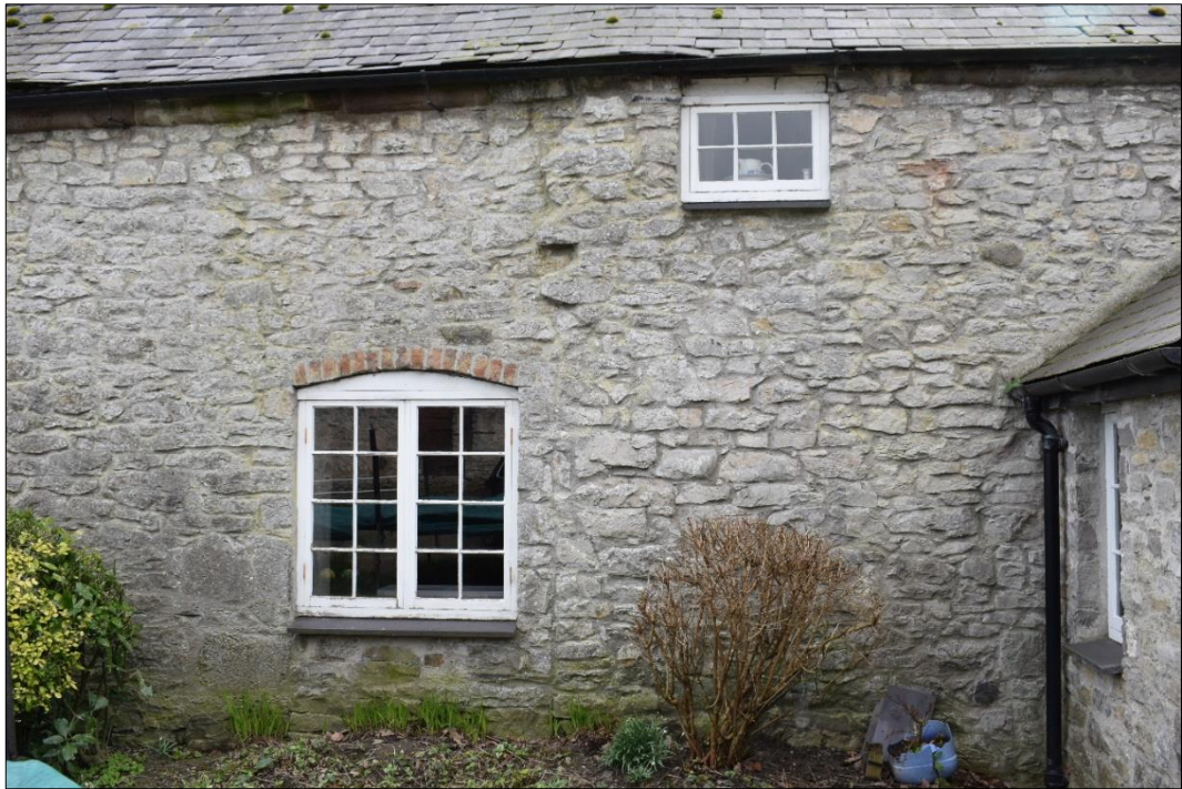
Fig. 13 The possible earlier doorway and obvious masonry joint. Photo CPAT 4335-0061
