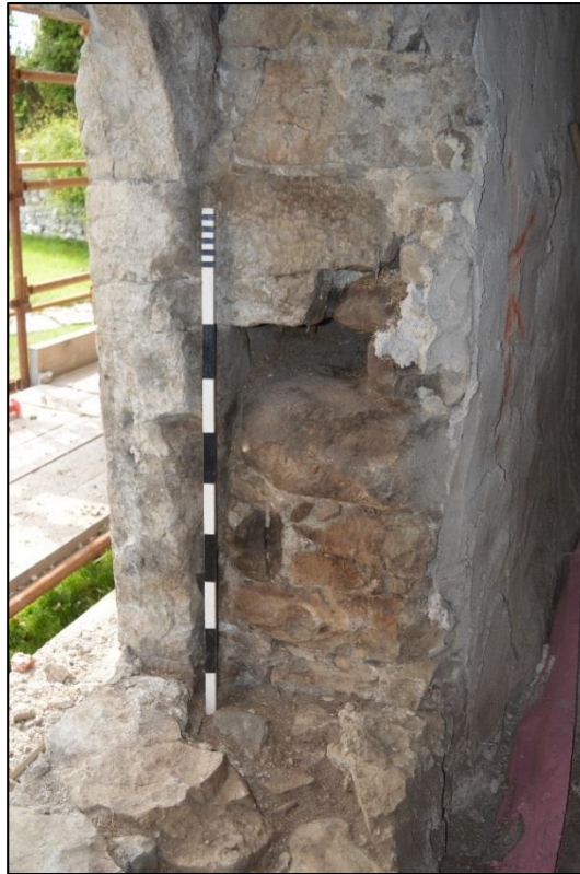
Fig. 20: The south-west side of the cyclopean doorway, note the slot for a wooden drawbar. Photo CPAT 4335-0139
