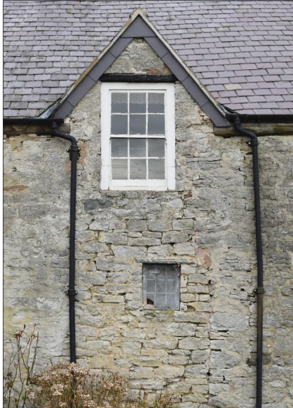
Fig. 7 The blocked doorway and inserted dormer window in the south-east elevation. Photo 4335-0009/11
