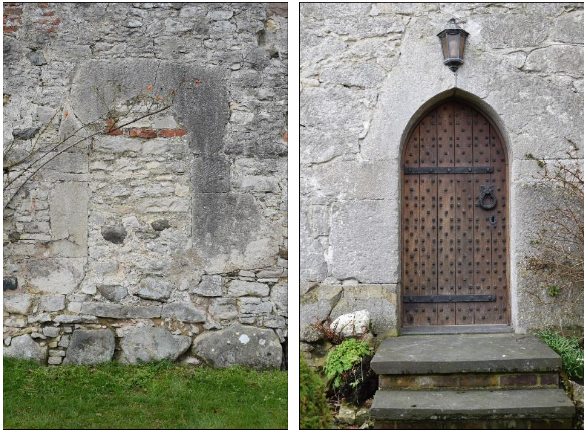
Fig. 6 The blocked pointed-arched cyclopean entrance and the matching entrance into the lodgings range. Photos CPAT 4335-0031 and 4335-0040
