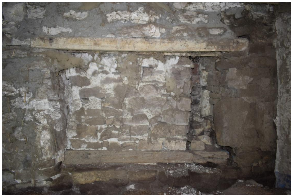
Fig. 10 Interior of the blocked first-floor window showing sandstone moulding and blocked ventilation slit on the left. Photo CPAT 4335-0068
