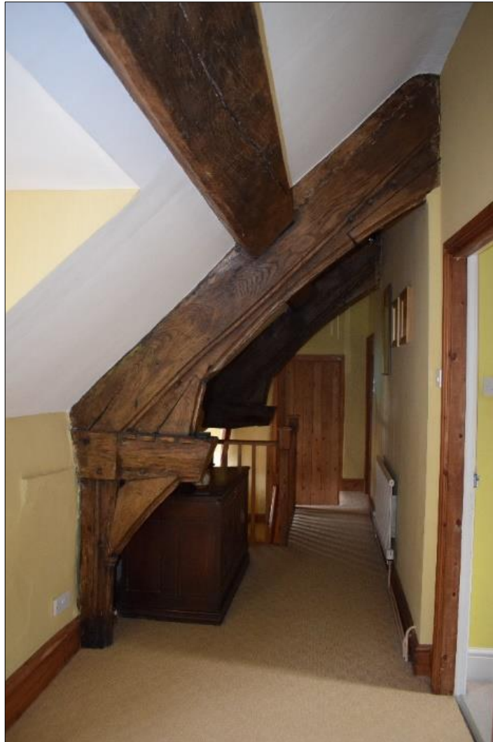
Fig. 4 Two of the hammerbeam principals associated with the original open hall (Trusses T4 and T5). Photo CPAT 4335-0005
