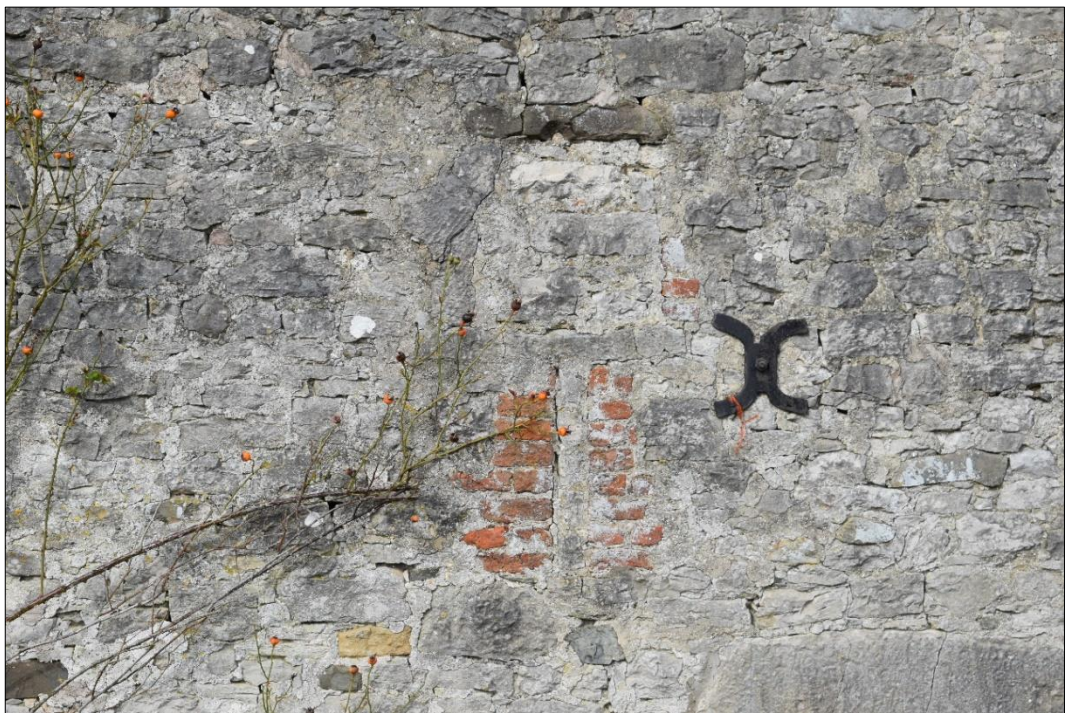
Fig. 8 The blocked first-floor window and later, infilled, ventilation slit above and to the left of the cylcopen doorway. Photo CPAT 4335-0039
