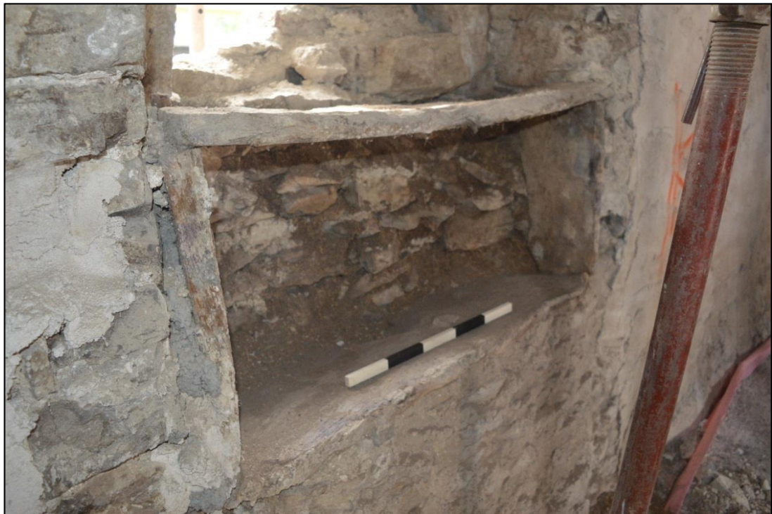
Fig. 18: The wooden frame within the blocking material of the cyclopean doorway. Photo CPAT 4335-0137
