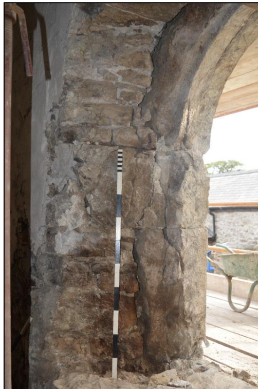
Fig. 21: The north-east side of the cyclopean doorway, note the iron hinge to the right of the top of the scale. Photo CPAT 4335-0140
