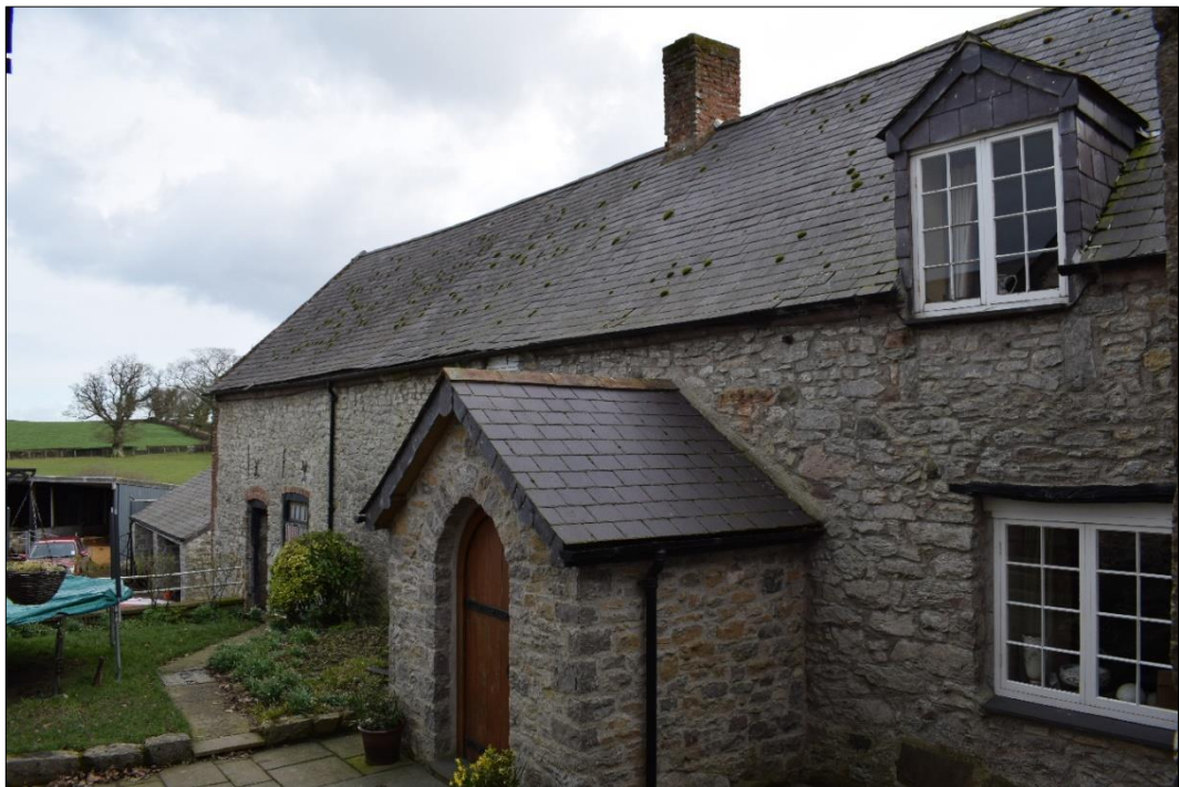
Fig. 14 The modern porch with adjacent windows with evidence for earlier openings. Photo CPAT 4335-0058
