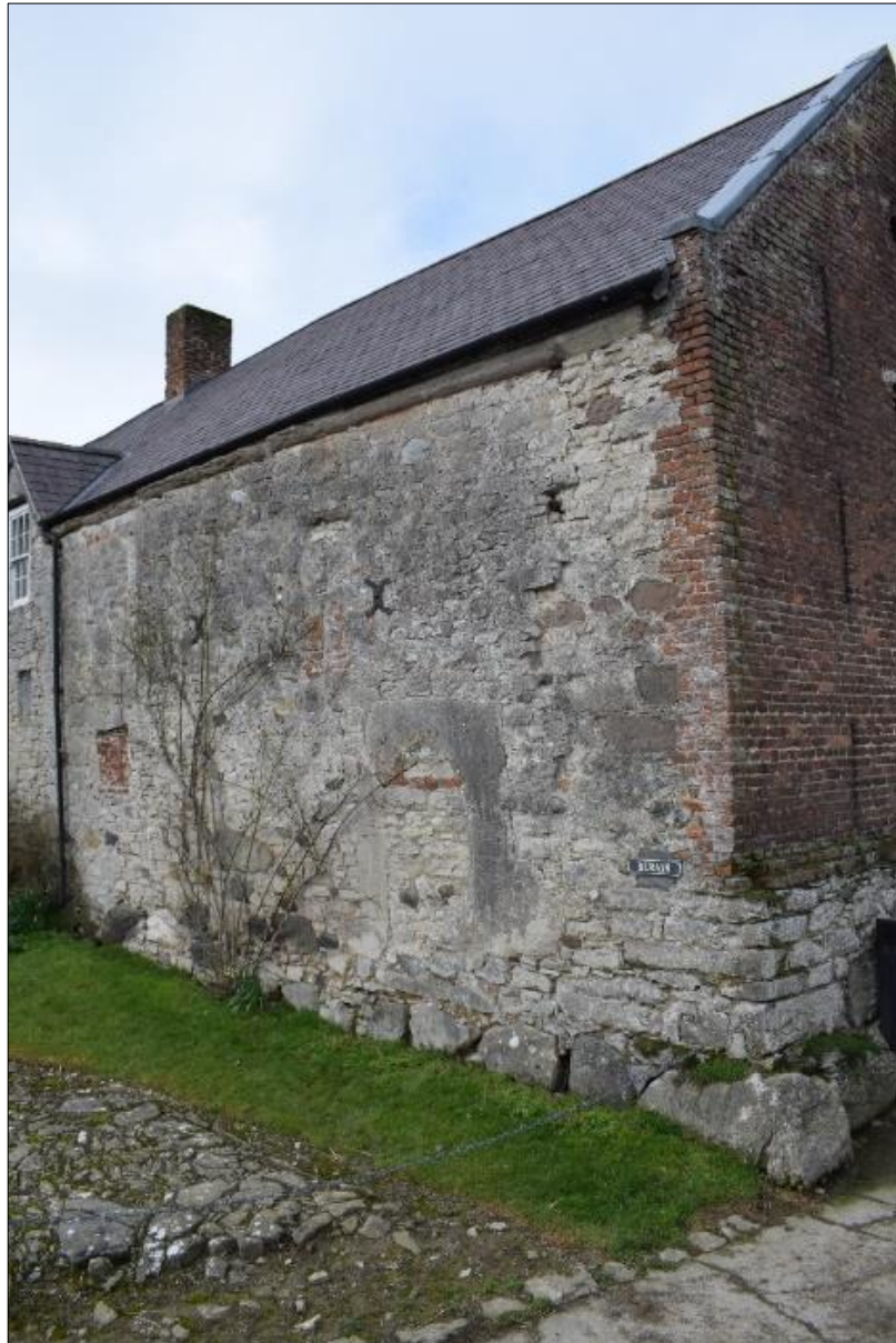
Fig. 11 The eastern corner of the south-east elevation, showing the two-tier plinth, changes in the masonry and the brick gable. Photo CPAT 4335-0049
