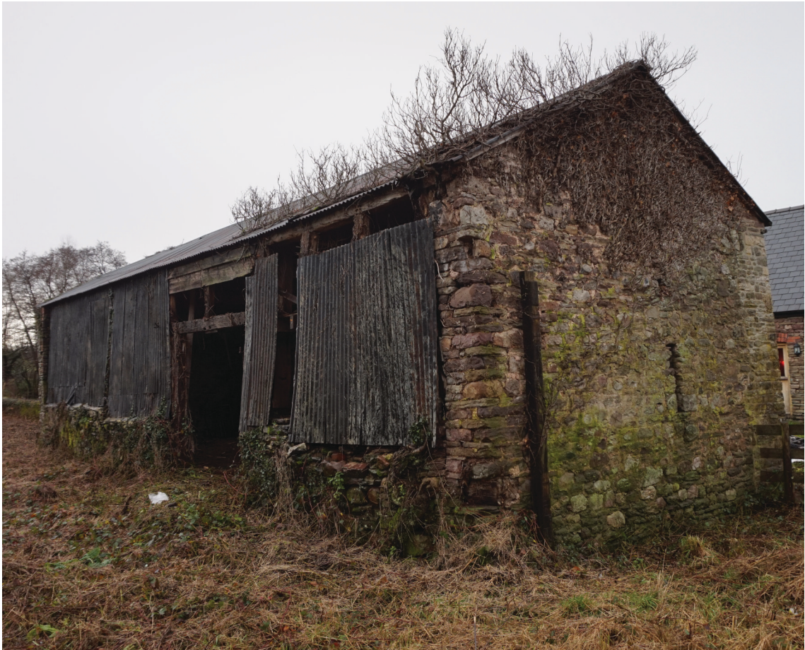
View of the barn from the South East
