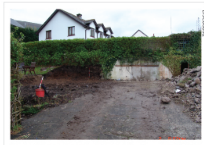
Plate 04: South boundary, retaining wall.
