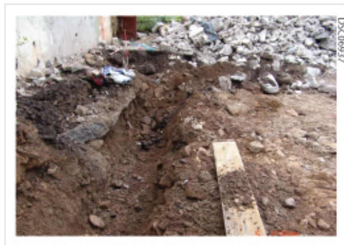
Plate 13: Concrete floor, connected to retaining wall, south trench.
