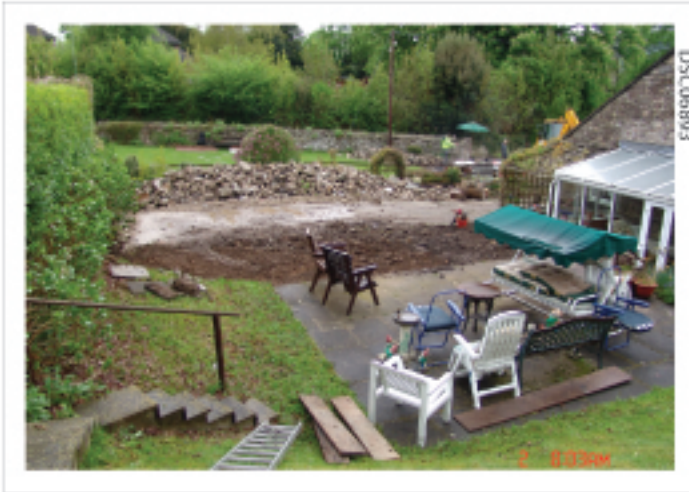
Plate 05: Remaining raised patio after ground reduction.
