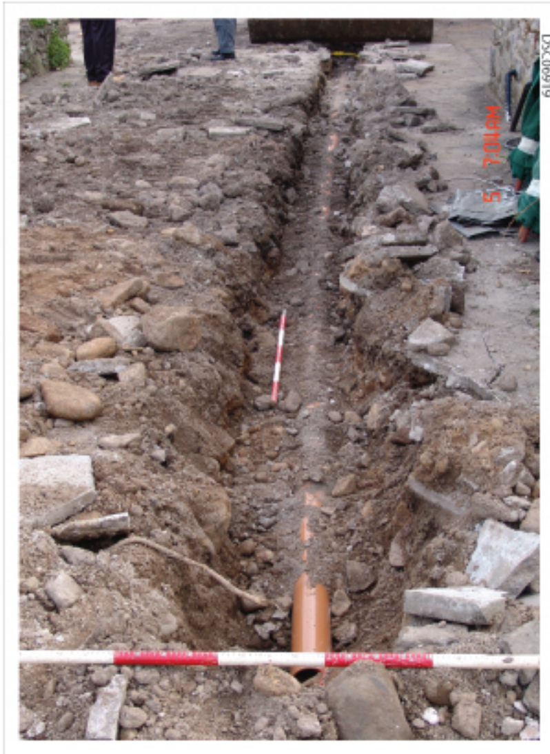
Plate 08: Service pipe replacement along western drive area
