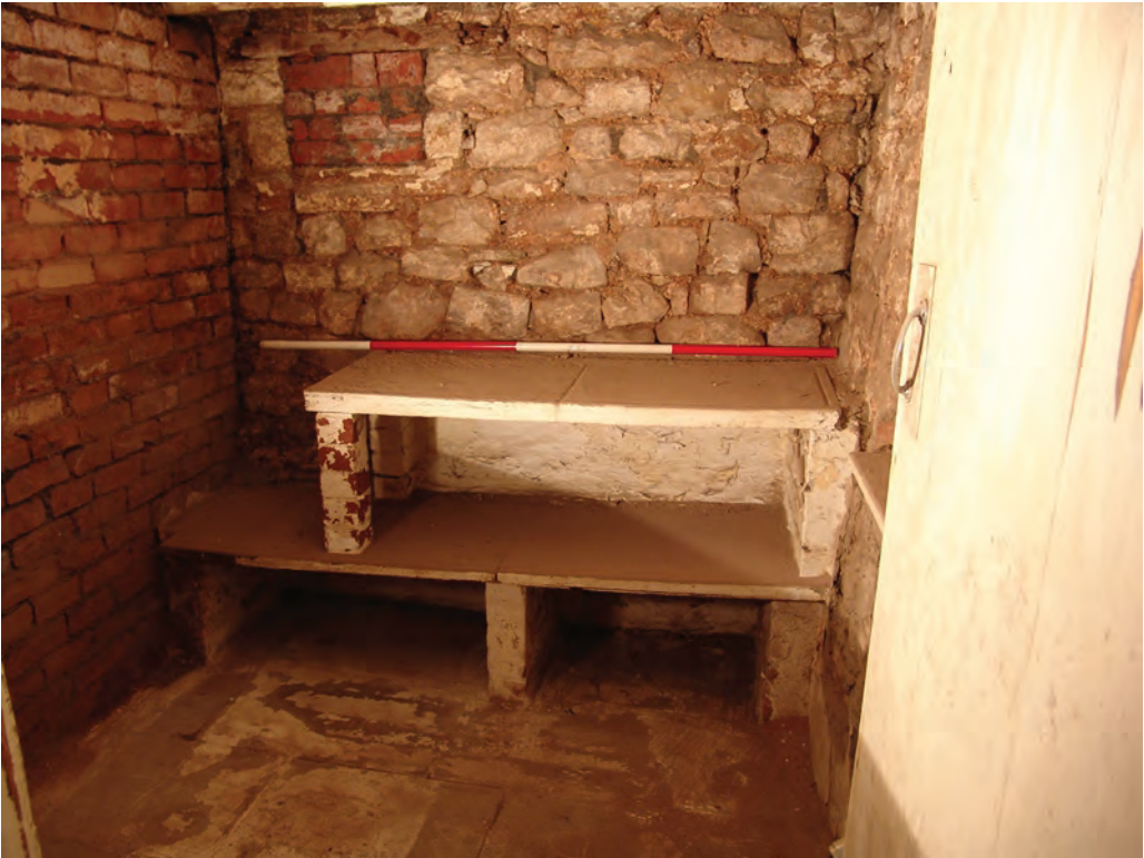
Reason for image Cold slab shelving, Flag floor. Blocked external window and new brick partition
