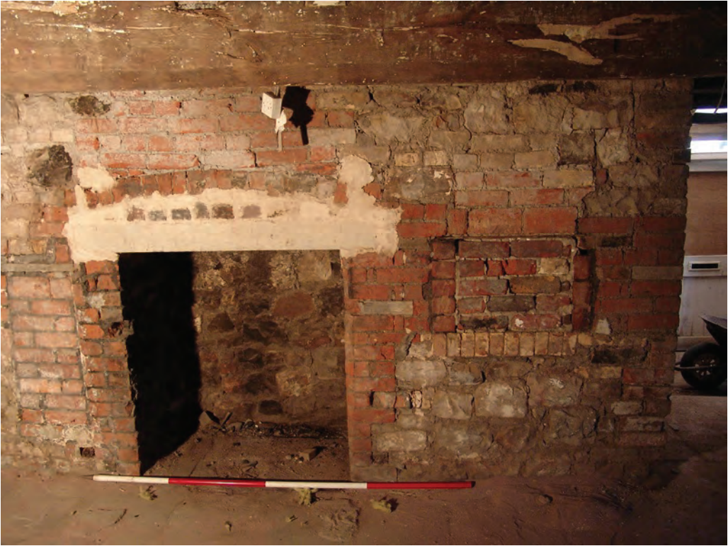
Reason for image Multiphase fireplace and later warm shelf? to right
