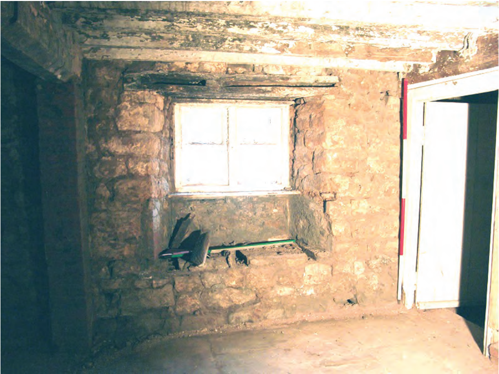
Reason for image South window setting, Re used window lintel
