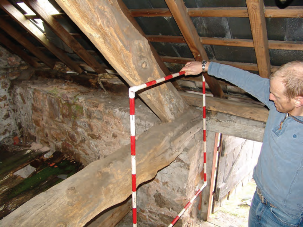
Reason for image Overview Oak truss and tie beam. (closed truss) oak plate added B1s
