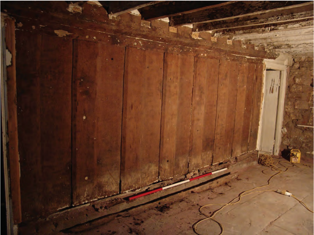
Reason for image Plank Partition, chamfered side.
