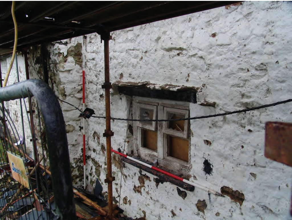
Reason for image Detail of dripstone above NE window of 1 living room and stairwell
