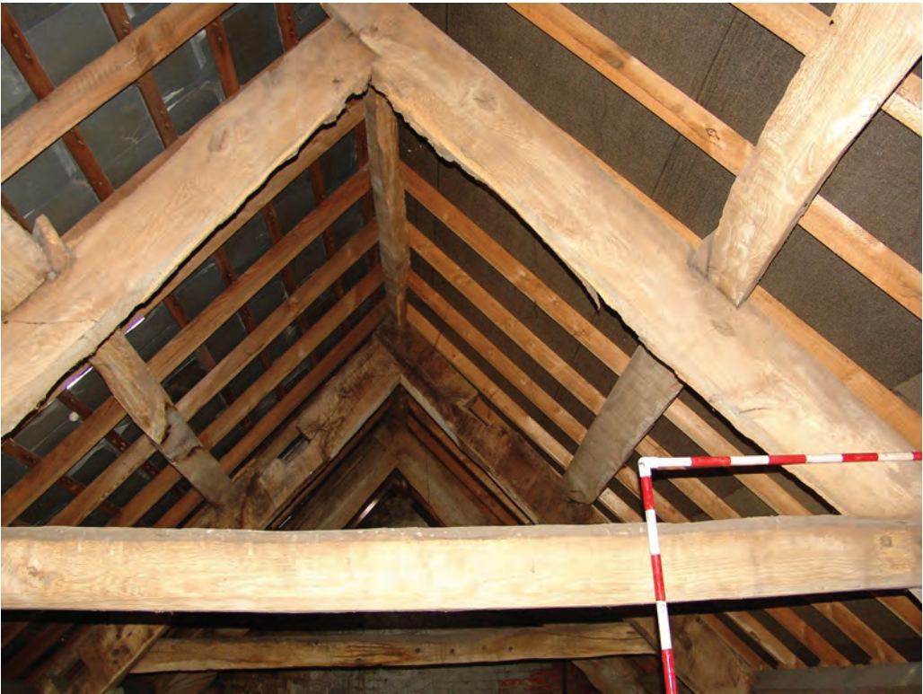
Reason for image Overview Oak truss (closed truss) and collar. Wooden peg joints. B1
