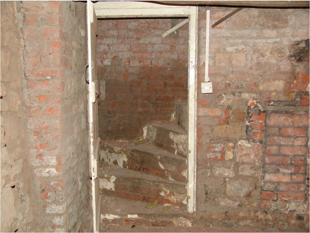
Reason for image Later phase brick N wall liner, stairwell and fireplace
