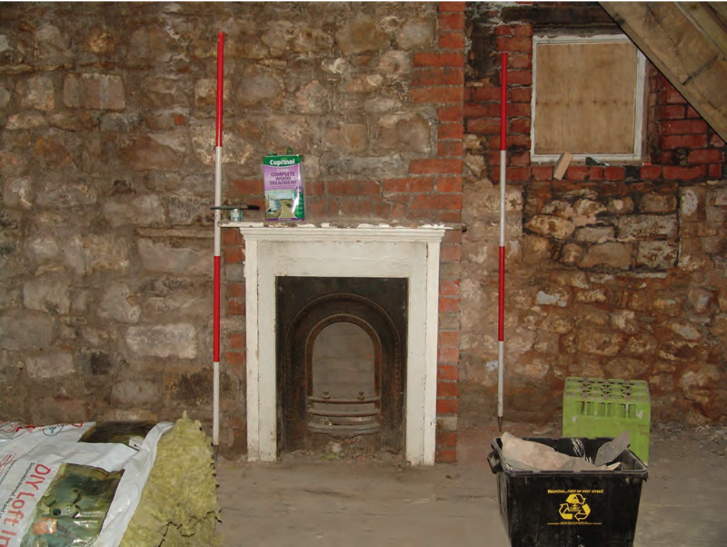
Reason for image East wall, chimney brest and two phase windows
