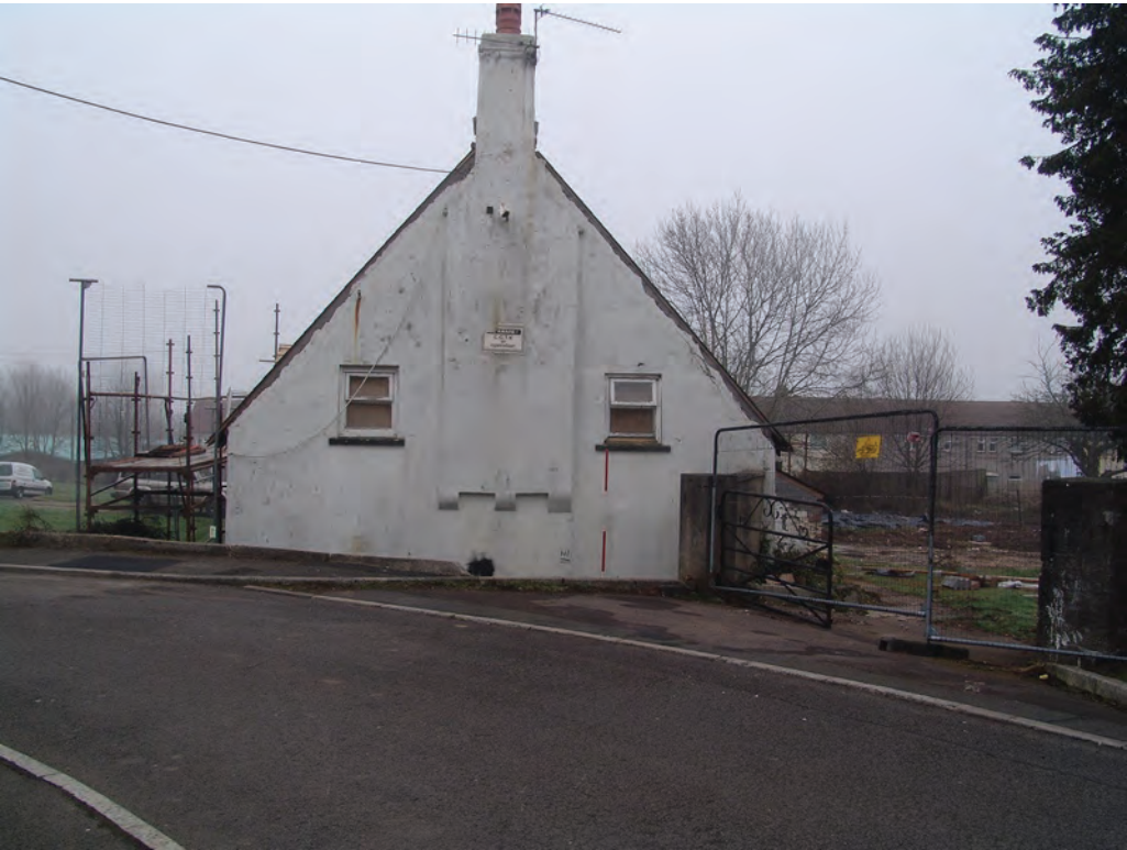
Reason for image Detail of W gable showing corbelled chimney breast
