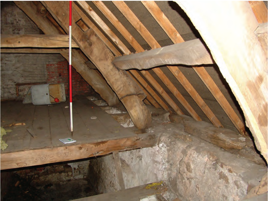
Reason for image Overview Oak upper cruck truss, collar an tie beam. B2n
