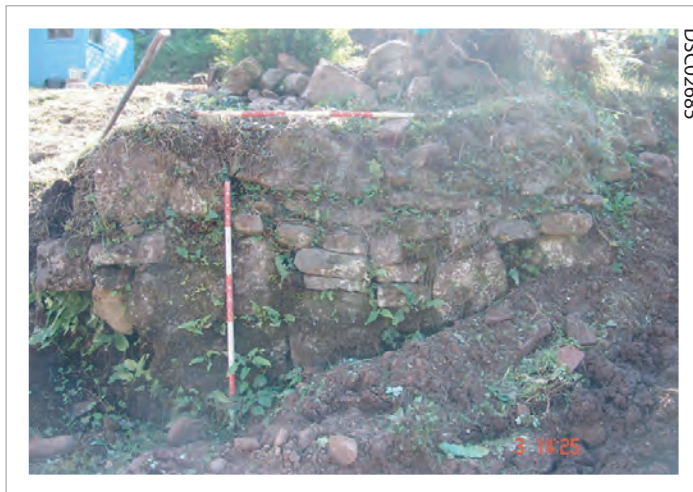
Plate 07: Section of structure, significantly different from the terrace revetment wall and at different alignment
