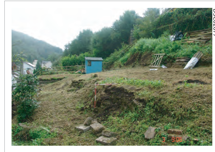
Plate 02: Upper terrace where the cabin foundation is to be placed
