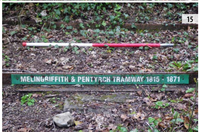
ILLUS 9 Post-1875 sluice gates at western end of feeder channel (east elevation) ILLUS 10 Cobblestone wall forming southern side of feeder channel ILLUS 11 East facing view along Mellingriffith feeder channel ILLUS 12 Detail view of iron girders spanning northern end of overflow channel ILLUS 13 General view of northern end of feeder channel ILLUS 14 Southern terminus of overflow culvert ILLUS 15 Detail of Mellingriffith & Pentyrch tramway
