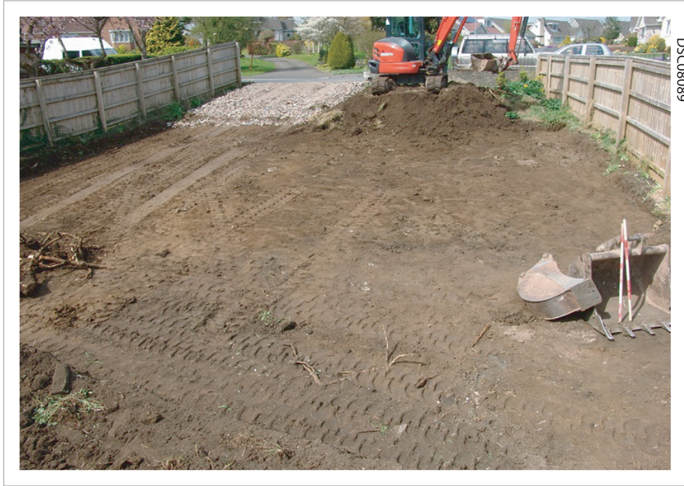
Plate 03: Site stripped of top soils [100], [101], & [102]
