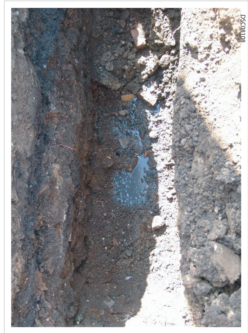
Plate 08: Trench 3 at \leq 3 m back fill [106] active waste pipe broken at 1.2m
