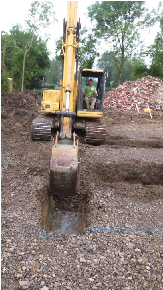
Plate 3: Excavation of foundations, facing southwest
