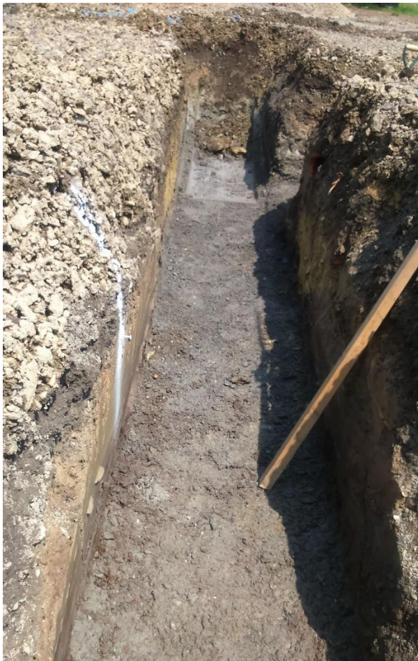
Plate 10: Foundation of front (northwest) side, Trench 1, facing northeast
