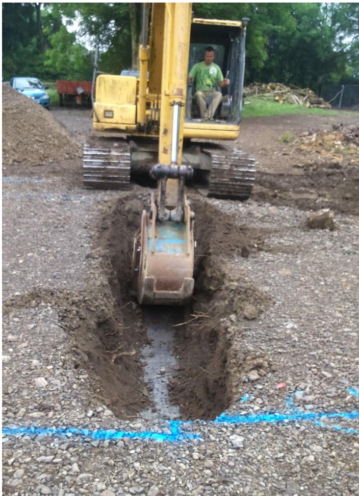
Plate 2: Rhos Common, Llanymynech, foundation trenches, facing northeast
