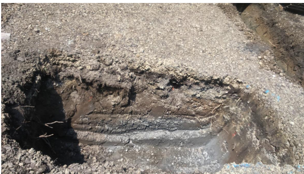
Plate 5: Foundation for master pillar, at the centre of the layout, Trench 2, facing southeast
