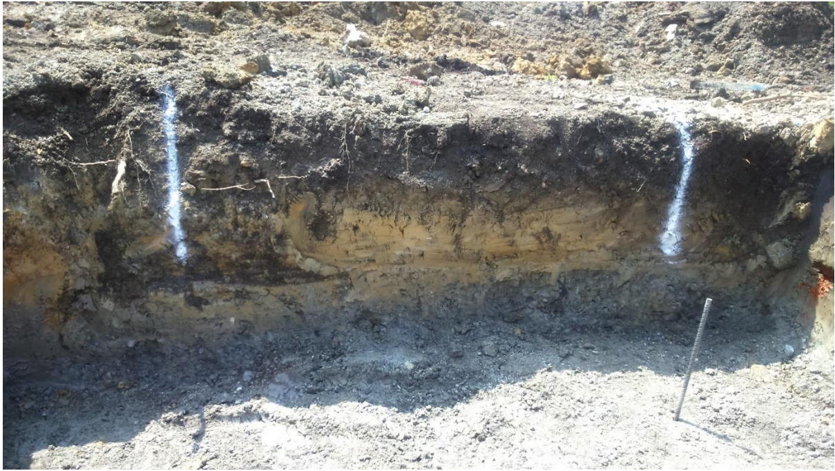
Plate 6: Foundation of southwest side, Trench 3, facing northeast
