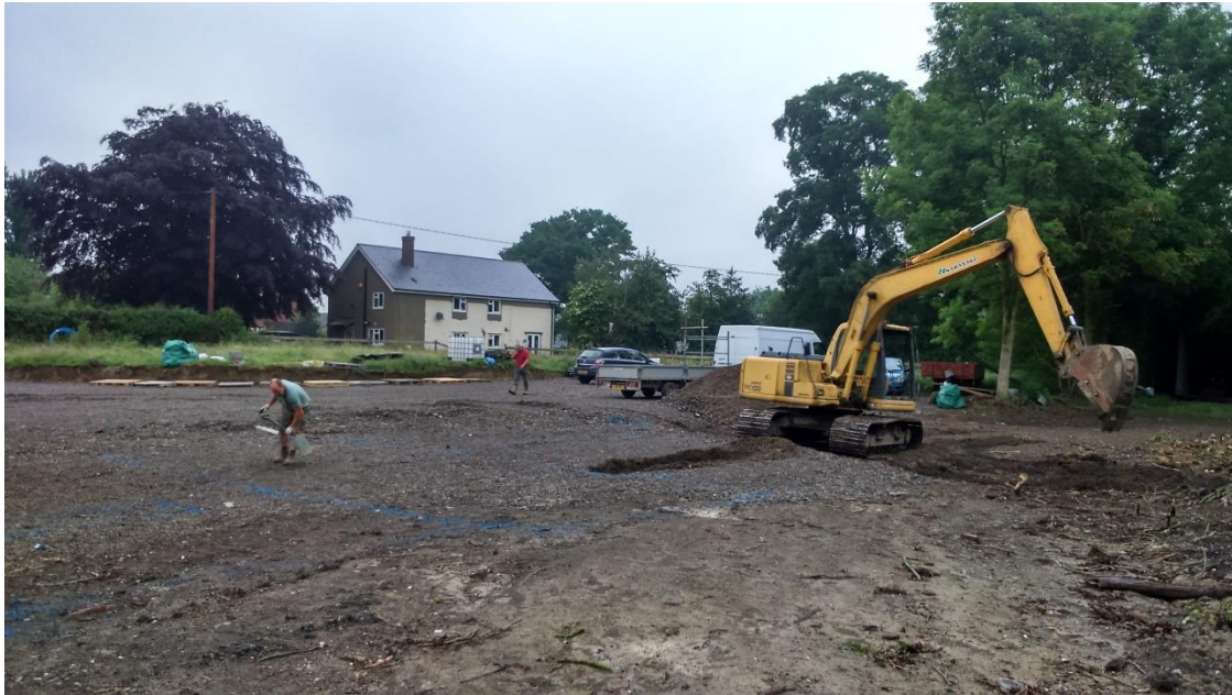
Plate 1: Rhos Common, Llanymynech, layout of foundation trenches, facing northwest
