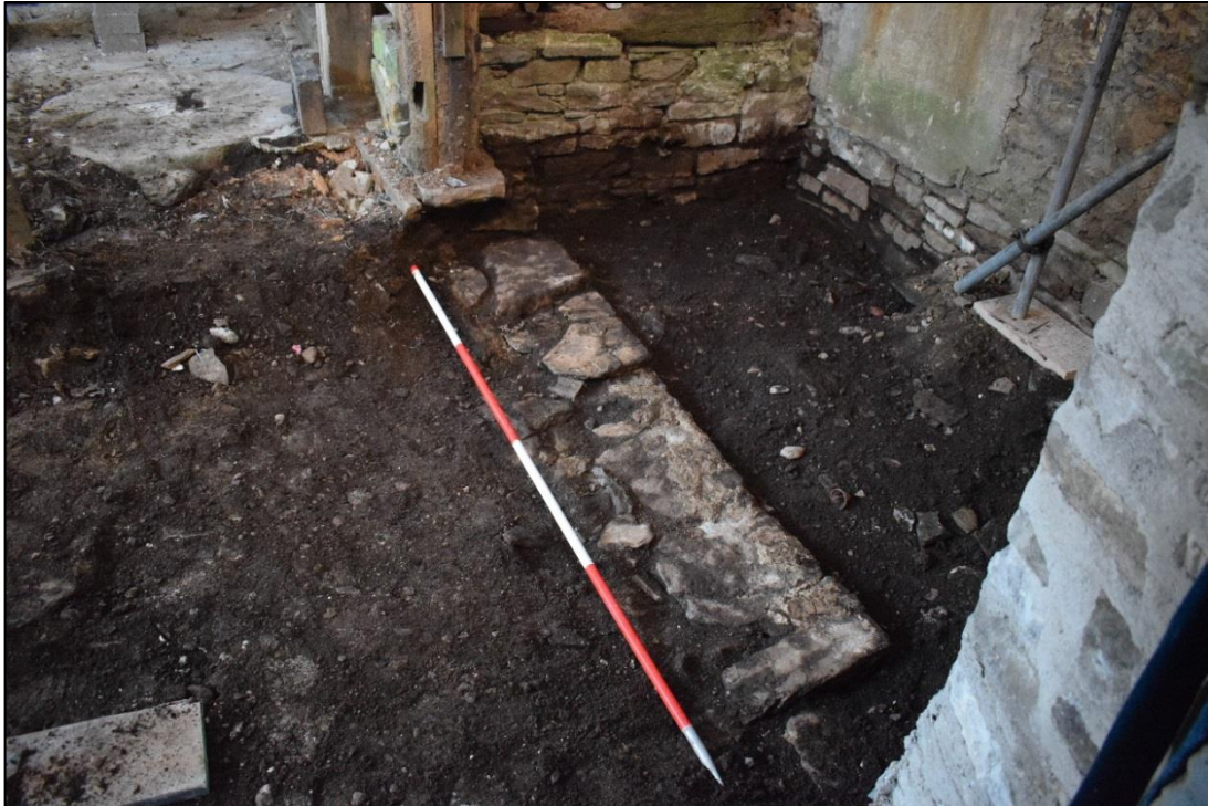
Fig. 9: The section of walling which defined the extension to the gearing pit, from the west. CPAT 4580-0001
