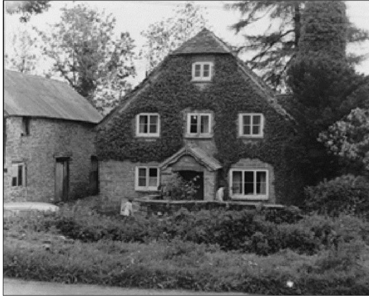
Fig. 6: Photograph taken in the 1950s showing the north-west elevation of the mill and adjoining barn
