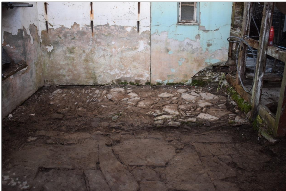
Fig. 10: The cobbled flooring of the dairy, from the south-west. CPAT 4580-0014
