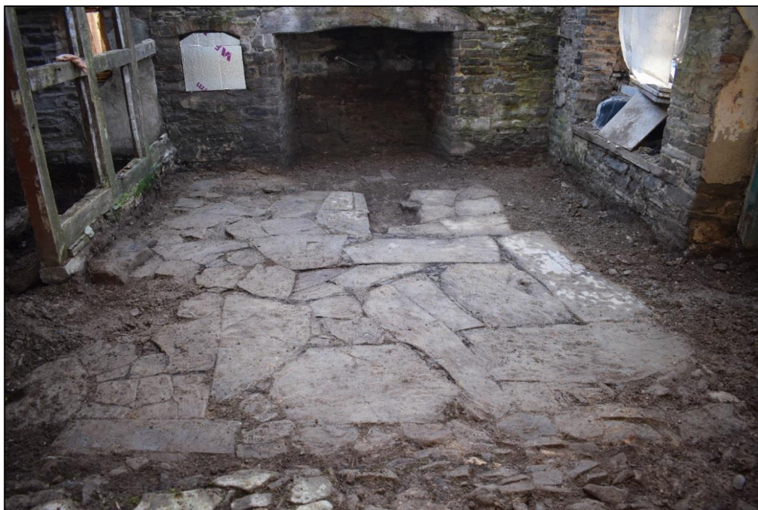
Fig. 11: The stone slab floor in the parlour and main passage leading to the mill, which lies to the left of the image. CPAT 4580-0009.
