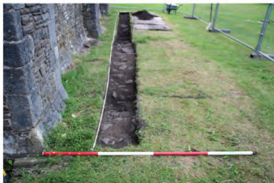
Plate 222. View of drainage trench with top soil removed and stone spread exposed. Looking east.
