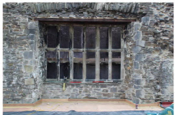
Plate 65: View of square headed late Tudor window in west wall. Looking west.
