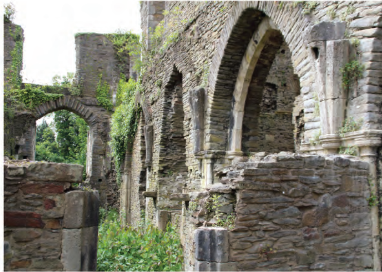
Plate 8: View of southern side of interior of Reredorter. Looking south,
