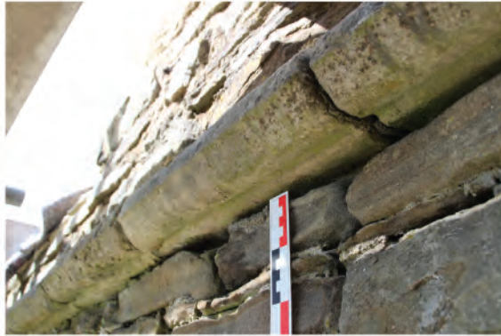
Plate 121. Detail of stringcourse with drip in east wall at far north end (121). Looking southwards.
