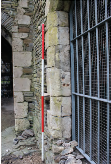
Plate 110. View of side jamb in doorway into Novice Room (136). Looking south.
