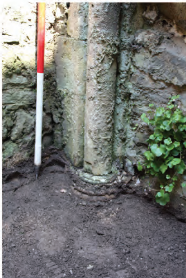
Plate 258. Cleared area around base of arch pier of Reredorter. Looking northeast.
