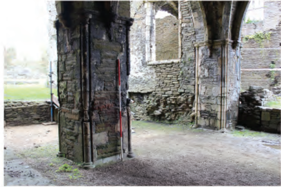
Plate 164. View of central bridge support pier below north side of bridge. Looking northeast.
