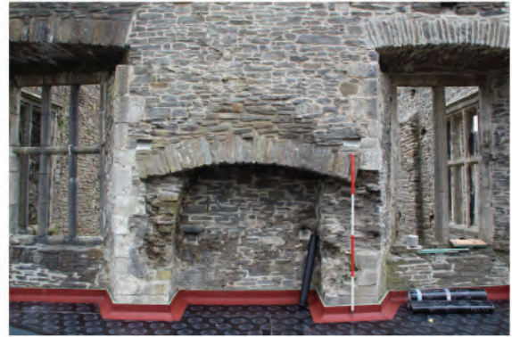
Plate 159. View of 16th century fireplace (169) set between the two square headed windows in the north facing internal elevation of the south wall of the bridge. Looking south.
