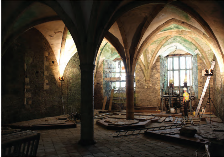
Plate 266. Working shot during timber lintel removal in undercroft. Looking south.
