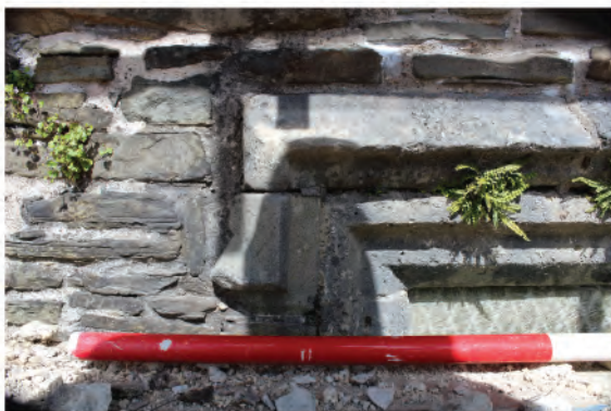
Plate 87. Detail shot of hood moulding in south wall window (62). Looking south.
