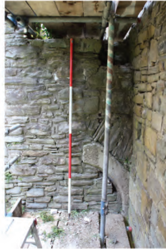
Plate 47: Remains of former late 15th century doorway in lateral cross wall of west wall. Looking north.
