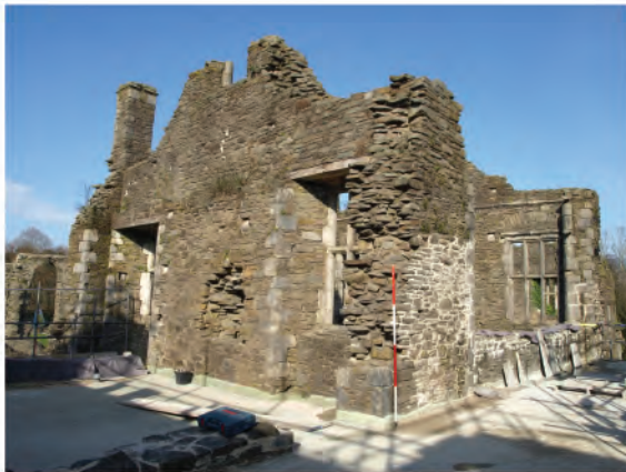
Plate 137. View of northern end of west facing internal elevation of east wall and bridge wall. Looking northeast.
