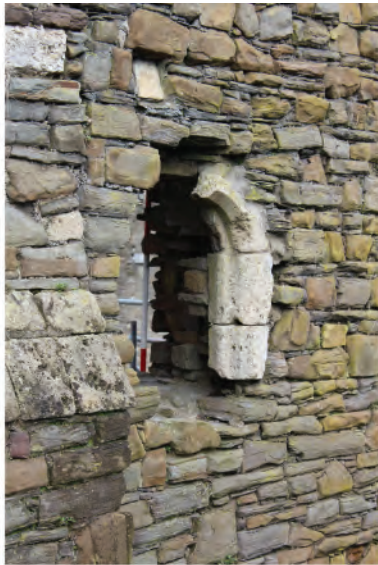
Plate 100: Remains of 13th century dormitory window in east wall (125). Looking northwest.
