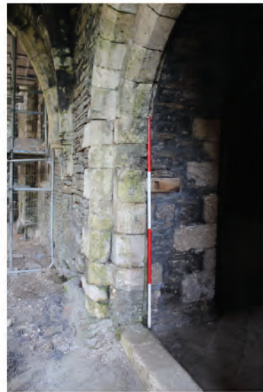
Plate 113. Detail of side jamb in doorway into undercroft (114). Looking southwest.
