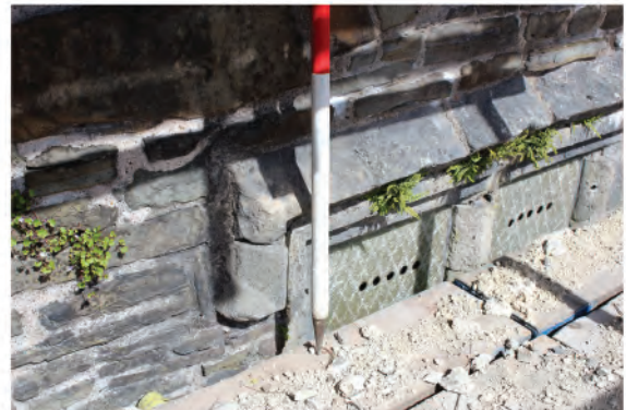
Plate 86: View of hood moulding in window in south wall (62). Looking northeast.
