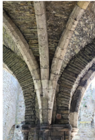
Plate 172. View of rib vaulting and moulded corbels at top of central bridge support pier. Looking south.
