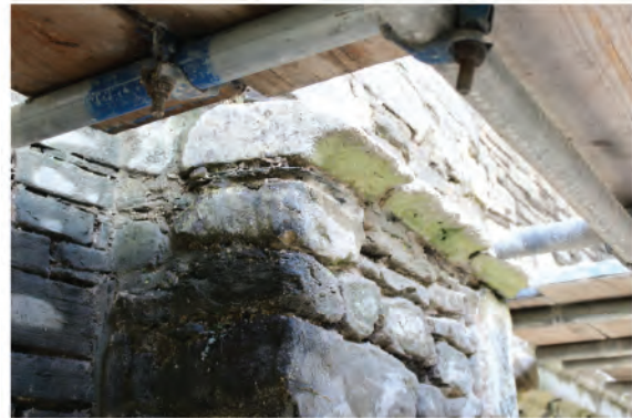
Plate 98: Detail of drip quoins in buttress (101) in east facing elevation of east wall. Looking northwest.
