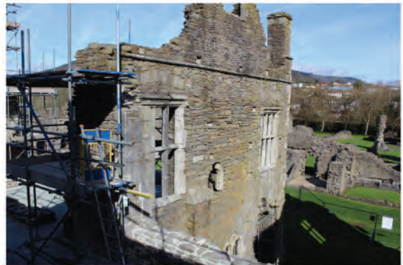
Plate 126. General view of north end of east wall. Looking northwards.
