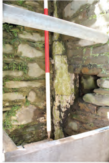
Plate 106. Remains of former tall 13th century lancet window (91) blocked in east wall. Looking southwest.
