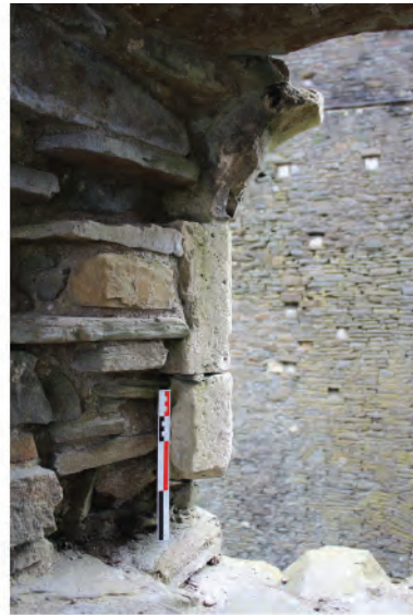
Plate 101: Remains of 13th century dormitory window in east wall (125). Looking east.
