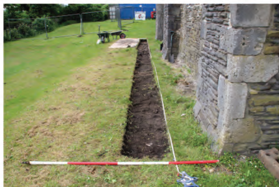
Plate 221. View of drainage trench with turf removed. Looking west.
