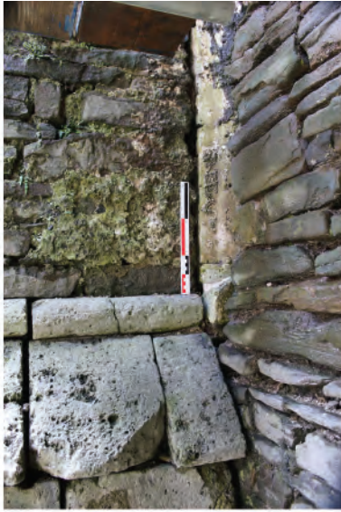
Plate 105. Remains of former tall 13th century lancet window (91) blocked in east wall. Looking southwest.
