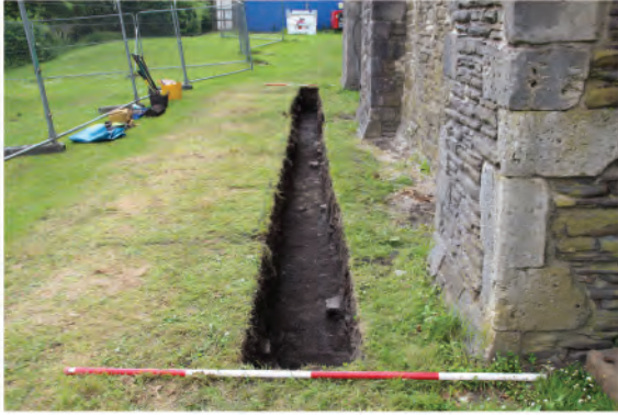
Plate 230. Finished trench. Looking west.
