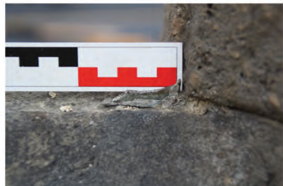
Plate 71. Fragment of lead and glass found in base mullion of late Tudor window in first floor of west wall (8). Looking eastwards.
