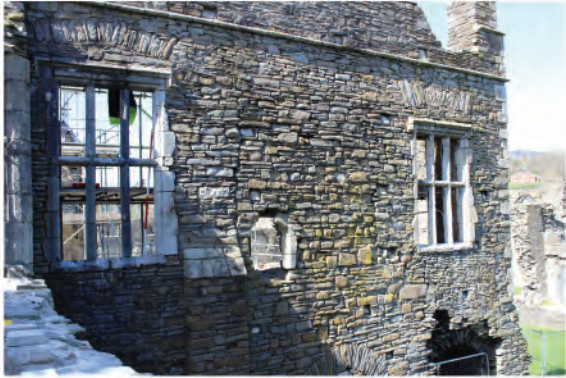
Plate 125. General view of north end of east wall. Looking northwards.
