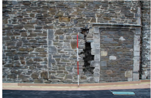
Plate 79: View of blocked 15th century doorway (197) and blocked in 13th century window in west wall (198). Looking west.
