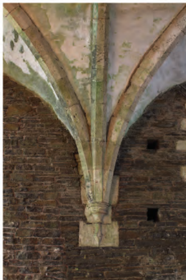
Plate 184. Ribbed vaulting and moulded corbels in undercroft. Looking west.
