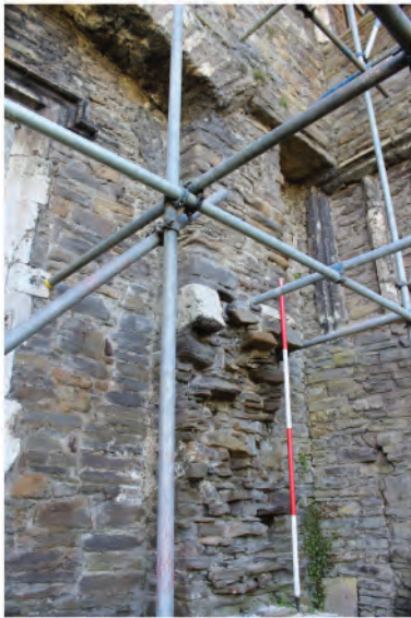
Plate 22: View of buttress (25) and relieving arch (12) in west wall. Looking southwards.
