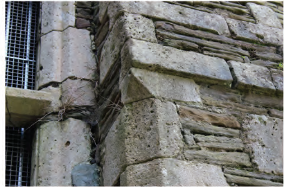
Plate 111. View of chamfered shoulder of buttress in east wall (126). Looking west.
