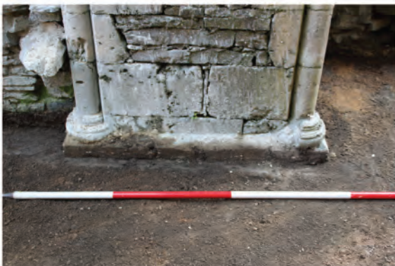
Plate 256. Cleared area around base of bridge support pier at Reredorter end. Looking east.
