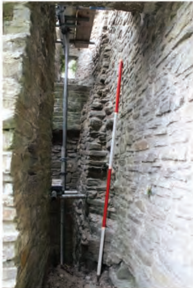
Plate 133. View of interior of vice passage within east wall (81). Looking south.
