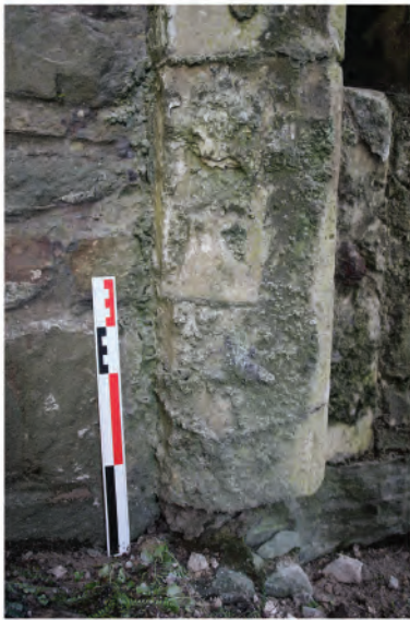
Plate 58: View of doorway jamb and stop in west wall at ground level (46). Looking east.
