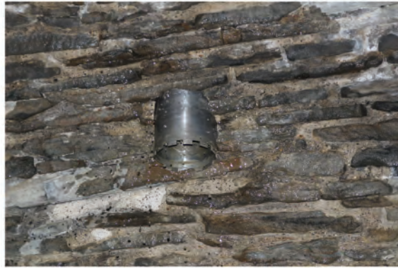
Plate 240. Boring in progress.
