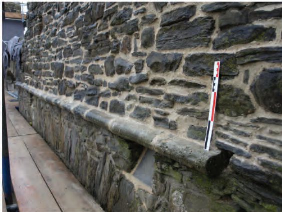
Plate 34: Detail of stringcourse in west wall (209). Looking northwards.
