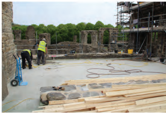
Plate 237. Boring equipment being prepared at point of roof. Looking north.
