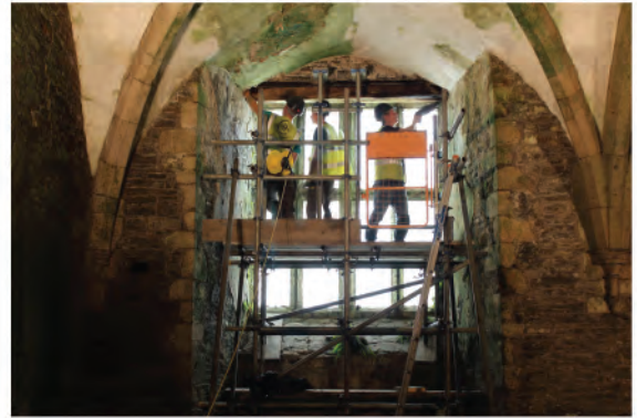
Plate 265. Working shot during timber lintel removal. Looking south.
