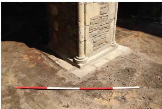
Plate 252. Cleared area around bridge support pier. Looking northeast.
