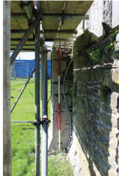
Plate 84: View of buttress (51) in south wall. Looking west.
