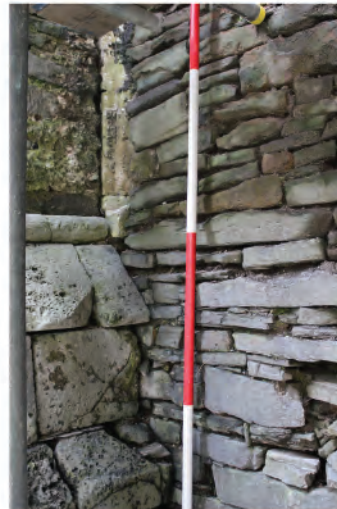
Plate 118. Detail shot showing mouldings from former 13th century lancet window in east wall (91). Looking southwest.
