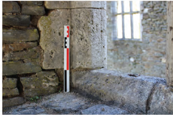
Plate 123. Detail shot showing side jamb in late Tudor window in east wall at north end (129). Looking northeast.
