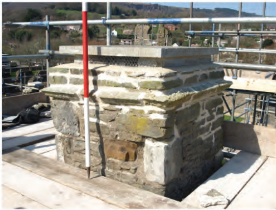
Plate 150. Chimney stack in west wall (1). Looking northwest.
