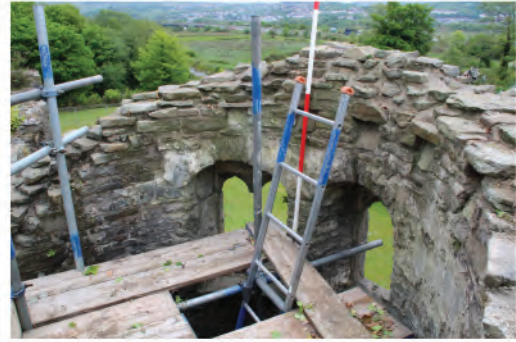
Plate 201. Upper interior level of Abbot's Stairwell. Looking southeast.
