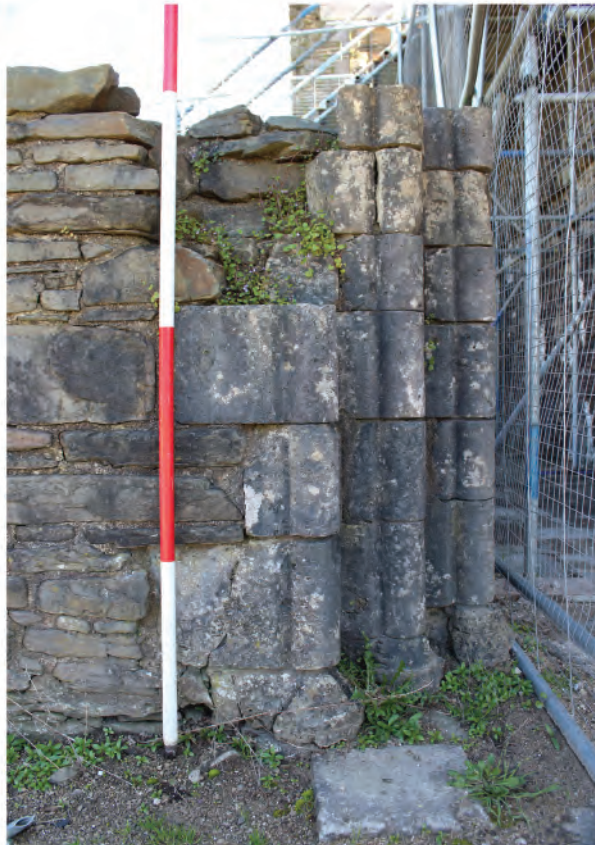
Plate 155. Detail shot of remains of moulded side jambs (15) of Slype passage at north end of west wall. Looking east.
