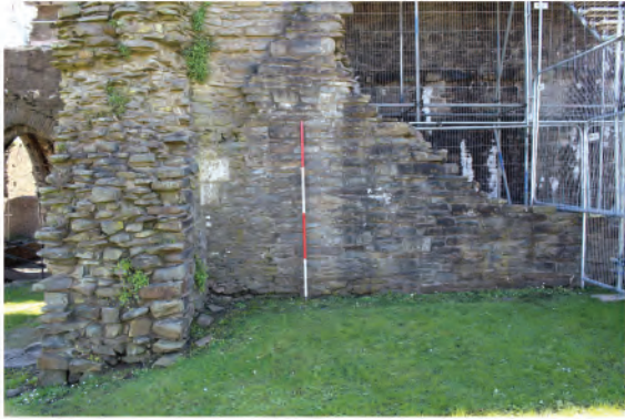
Plate 153. View of north facing elevation of northernmost wall (Parlour). Looking south.
