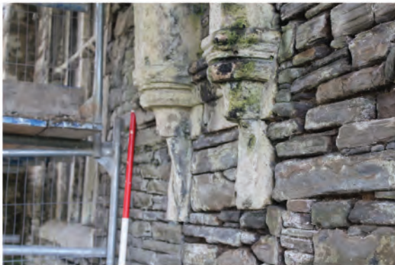
Plate 171. Detail shot of decorative moulded corbels supporting rib vaulting at west end of bridge alongside entrance to undercroft. Looking southwest.
