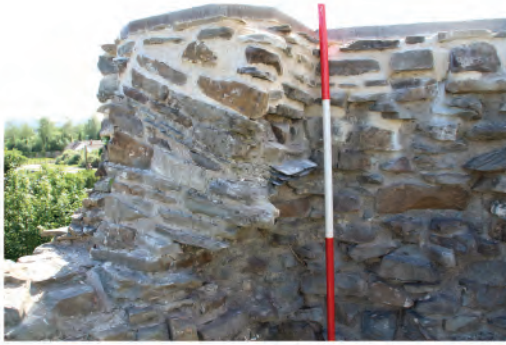
Plate 212. View of spring of former doorway arch at upper level of Abbot's Stairwell. Looking southwest.
