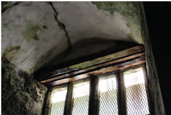
Plate 262. Timber lintels in east window prior to removal. Looking southeast.
