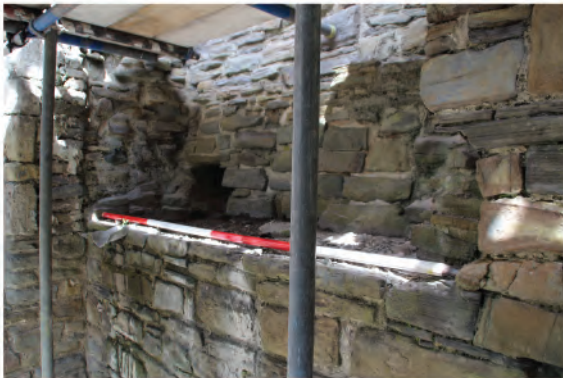
Plate 52: Base of former 15th century doorway in west wall at first floor level (33). Now blocked. Looking northwards.
