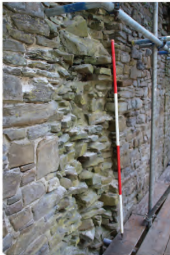
Plate 46: Exposed wall core from former buttress in west wall (34). Looking south.
