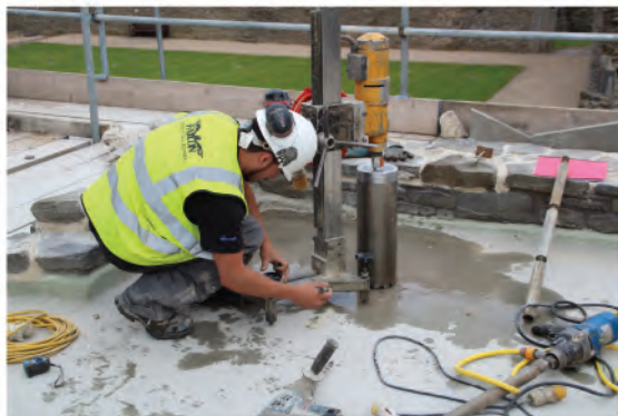
Plate 238. Boring equipment being prepared at point of roof. Looking north
