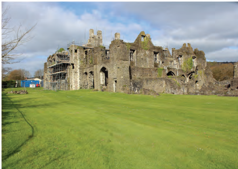
Plate 2. View of Tudor Mansion during consolidation work. Looking northwest.
