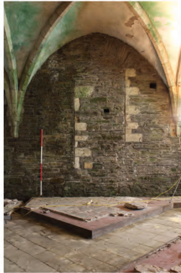
Plate 182. Blocked 13th century lancet window in west wall in undercroft. Looking west.
