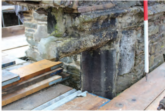
Plate 26: Detail of top and side jamb of oriel window (6). Looking southeast.
