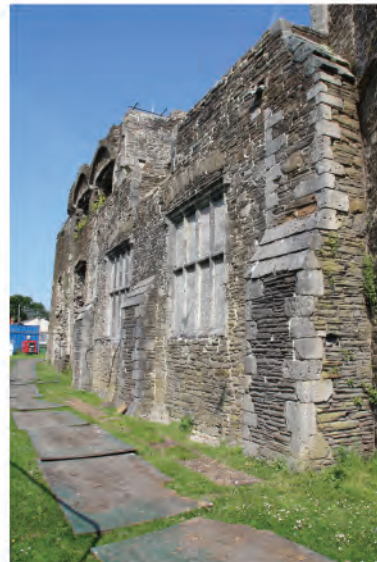
Plate 10: View of South wall following scaffold removal. Looking westwards.
