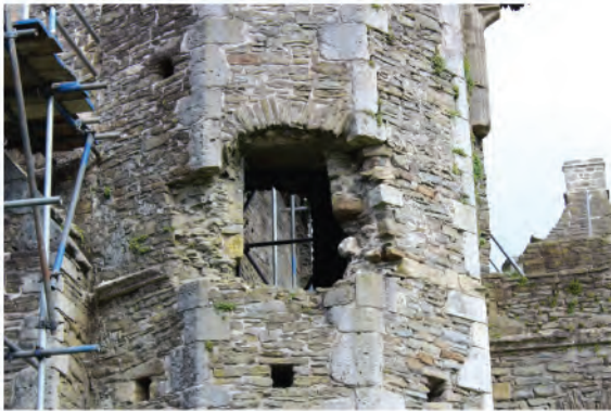
Plate 194. View of 15th - 16th century window in Abbot's Stairwell. Looking north.
