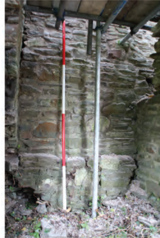
Plate 207. Interior view of Abbot's Stairwell showing blocked former entrance. Looking west.
