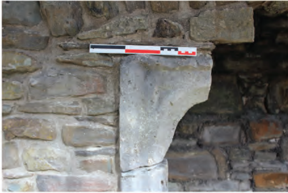
Plate 141. Detail shot of top corner jamb of 15th - 16th fireplace (186) showing sunken spandrel. Looking east.
