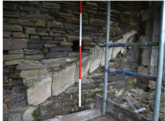
Plate 15: View of remains of Sutton stone handrail alongside Day Stairs in West wall. Looking southeast.
