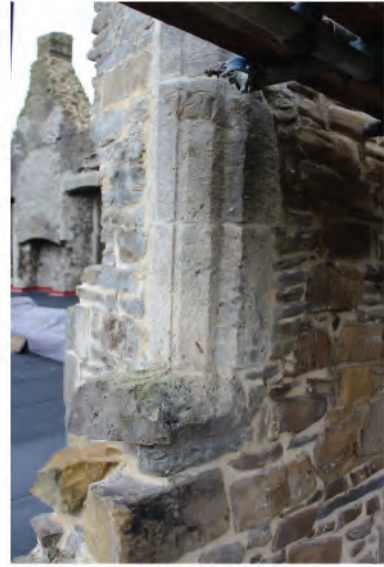
Plate 27: Remains of base and side jamb of northern window in west wall (10). Looking southeast.
