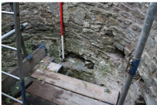
Plate 204. Interior view of Abbot's Stairwell showing remains of steps of newel stairs. Looking east.
