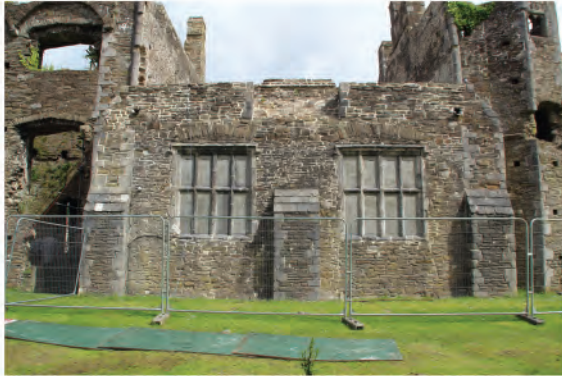
Plate 83: View of south wall following scaffold removal. Looking north.
