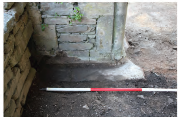
Plate 253. Cleared area around bridge support pier alongside Rredorter. Looking south.
