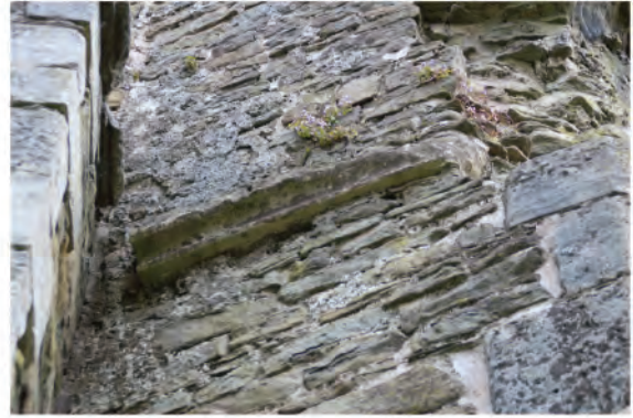
Plate 197. Stringcourse in southwest facing elevation of Abbot's Stairwell. Looking north.
