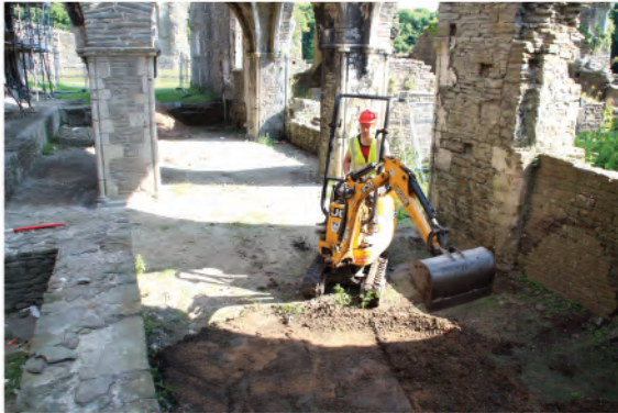
Plate 248. Working shot during clearance of vegetation in courtyard area. Looking northeast.
