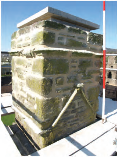
Plate 44: Detail of feature in chimney in west wall (28). Looking northwest.
