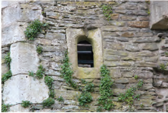
Plate 196. Detail view of small loop window in east elevation of Abbot's Stairwell. Looking west.
