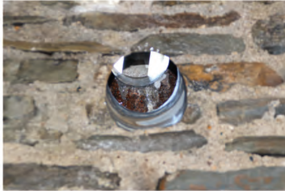
Plate 239. Completed bore hole through barrel vaulting at east end of ceiling.
