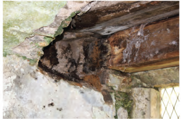
Plate 268. Timber lintel removed in west window. Looking southeast into beam slot.
