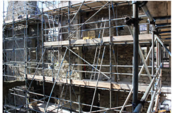
Plate 128. General view of east wall with scaffolding in place. Looking west.
