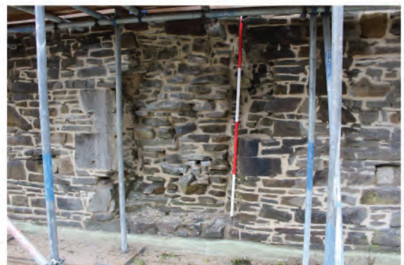
Plate 77: Remains of blocked in former 13th century dormitory window (200) in west wall internal side. Looking west.
