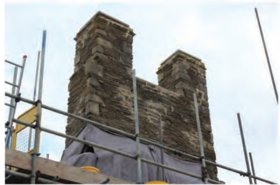
Plate 134. Chimney pair at southern end of east wall. Looking northwest.
