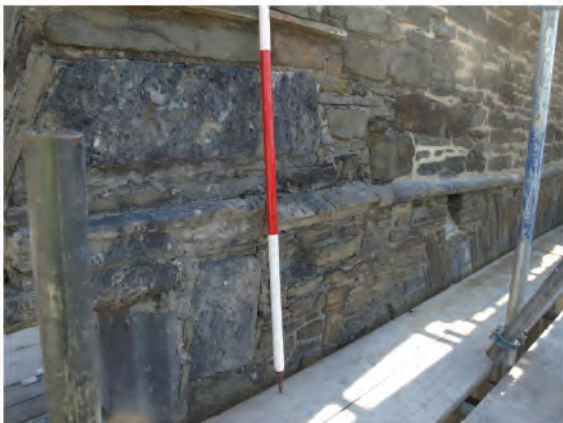
Plate 36: Detail shot showing side jambs in oriel window (6) and replaced stringcourse. Looking southeast.
