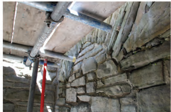
Plate 55: Detail of top arch of former 13th century lancet window (41) in west wall. Looking north
