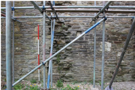
Plate 107. Scarring in east facing external elevation of east wall at far southern end (86). Looking west.
