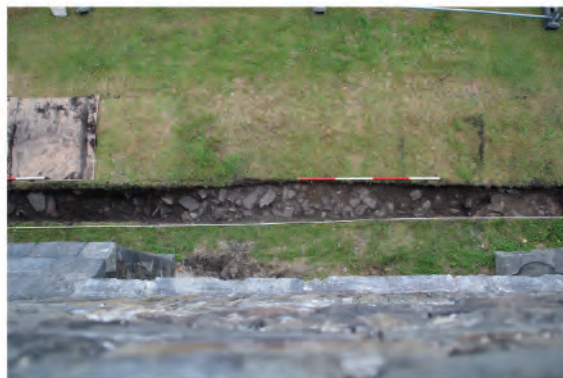
Plate 223. Overhead view of drainage trench showing stone rubble spread.
