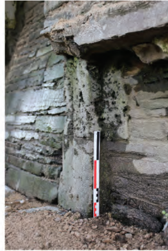
Plate 116. Detail view showing moulded Sutton stone below buttress (102) in east wall. Looking northwest.
