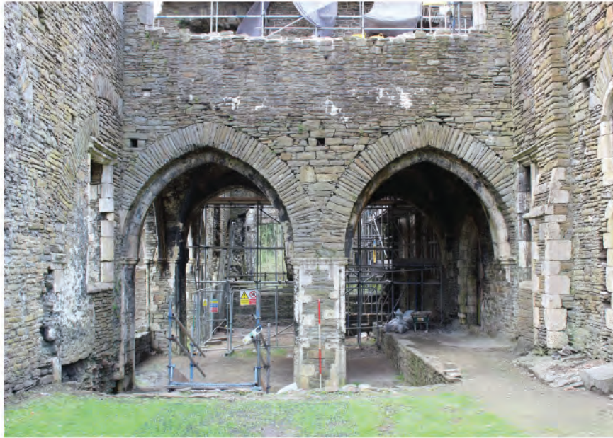
Plate 156. View of north facing north wall of vaulted bridge. Looking south.
