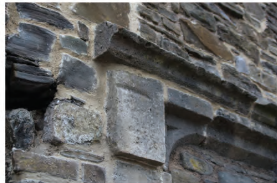
Plate 81: Detail showing hood and top shoulder of flat arch of blocked late 15th century doorway in west wall. Looking northwest.
