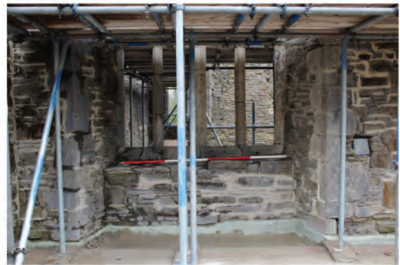
Plate 151. Late Tudor square headed window in east wall (107). Looking east.
