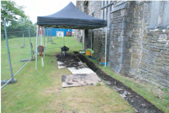
Plate 226. Working shot. Looking west.
