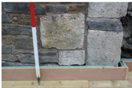
Plate 82: Re-used ashlar quoin with mason's mark 'V' used as block in stone of late 15th century doorway in west wall (197). Looking west.
