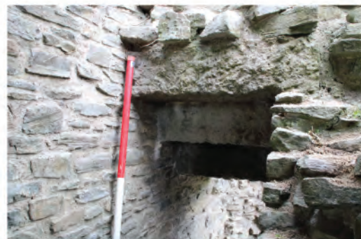
Plate 205. Interior view of vice passage showing limestone blocks supporting roof of passage. Looking north from within Abbot's Stairwell.
