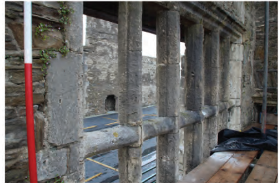
Plate 35: View of late Tudor mullioned window (8) in west wall at first floor level. Looking southeast.
