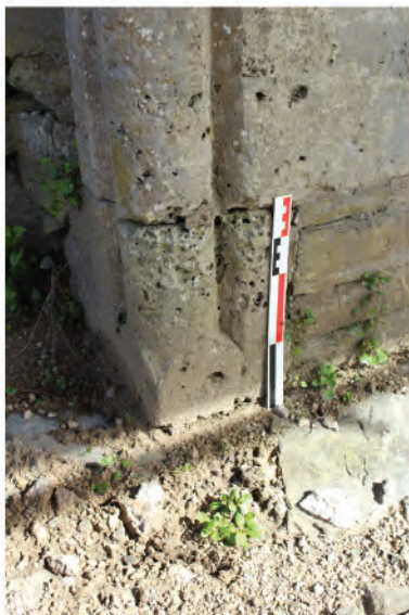
Plate 18: Detail of base order of door jamb into Slype passage at north end of west wall (South side). Looking southeast.
