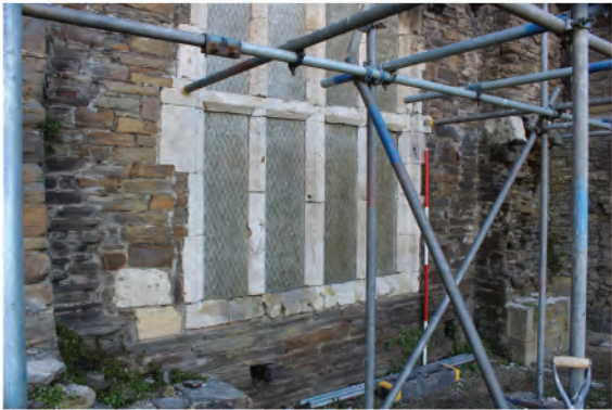
Plate 28: View of late Tudor window in west wall (24). Looking southwards.
