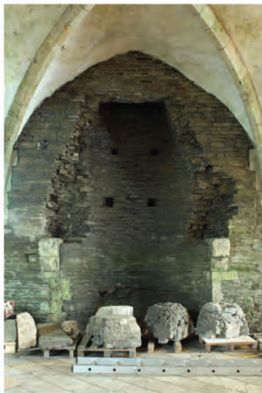
Plate 180. View of fireplace in east wall of undercroft. Looking west.
