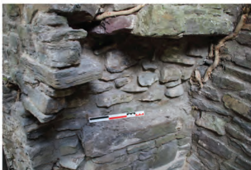
Plate 216. View of remains of spring of arch of former doorway in first floor level of Abbot's Stairwell. Looking southwards.
