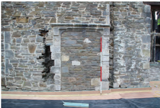
Plate 80: View of blocked late 15th century doorway (197). Looking west.
