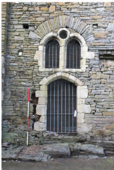
Plate 91: View of doorway (136) into Novice Room in east wall. Looking west.
