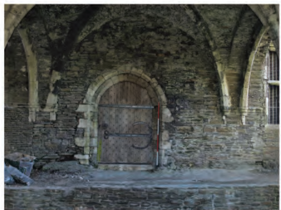
Plate 130. Doorway in Undercroft (114). Looking west.
