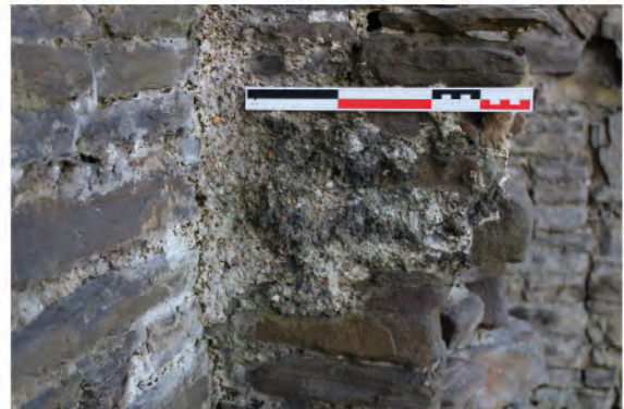
Plate 23: Detail of remains of historic render at side of buttress and below relieving arch (11).
