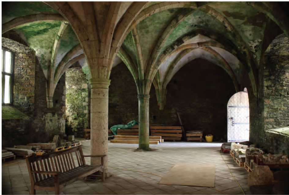
Plate 175. General view of Undercroft / Day Room. Looking north.
