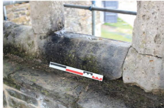
Plate 69: Detail of base jamb in late Tudor window in west wall (8). Looking west.
