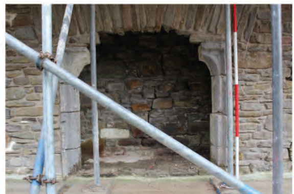
Plate 140. View of 15th - 16th century fireplace (186) in west facing internal elevation of east wall. Looking east.
