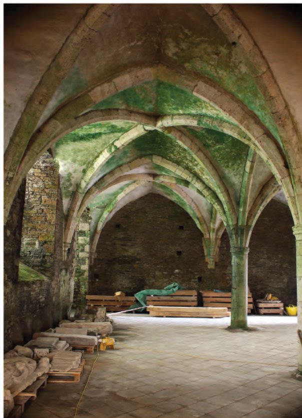
Plate 176. General view of Undercroft / Day Room. Looking north.
