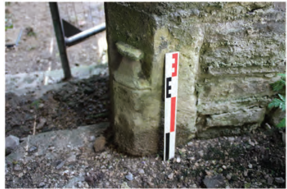
Plate 59: Detail shot of bottom order stop moulding in western jamb of doorway in E-W cross wall (46). Looking south at opposing west side of doorway. Other stop heavily weathered.
