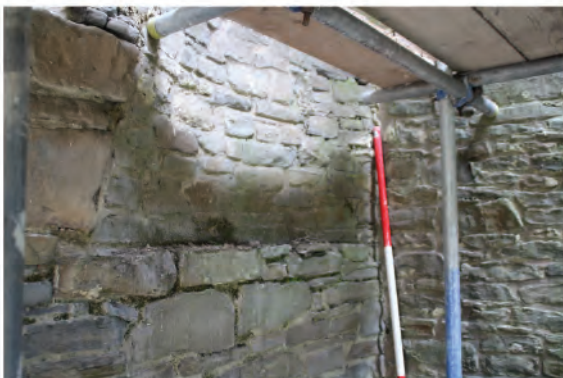
Plate 54: Curving feature in west facing elevation of west wall at first floor level. Part of former stair arrangement (37). Looking south.
