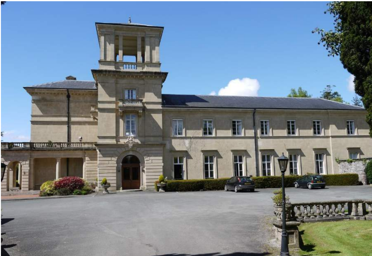
Photo 20. View of eastern facade
