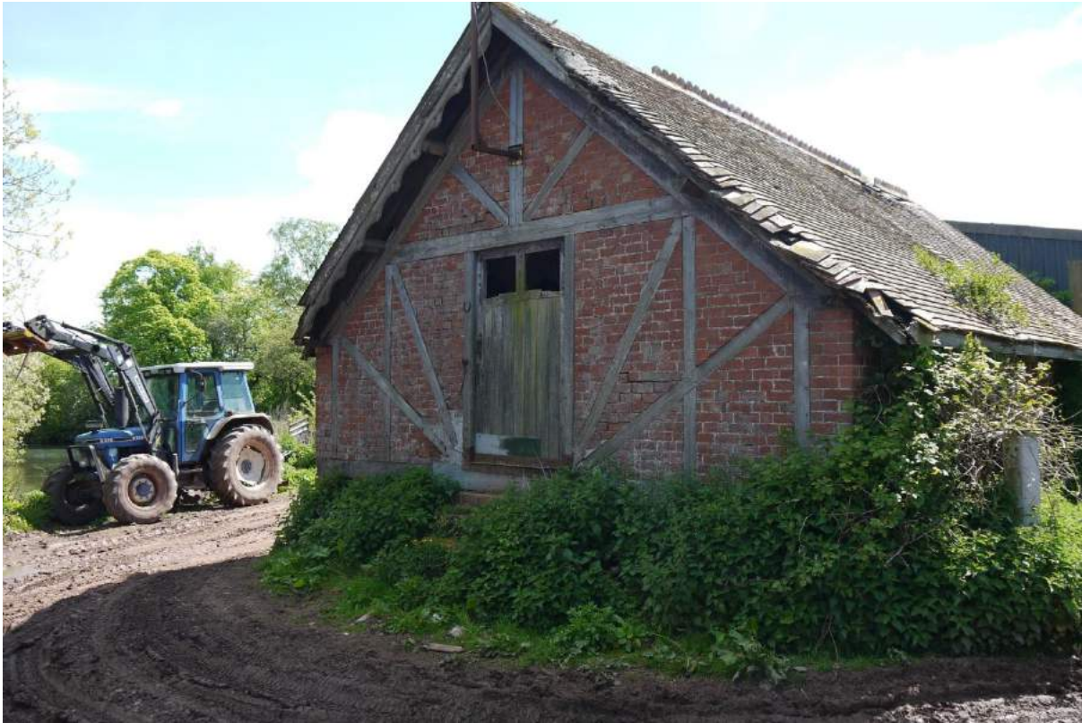
Photo 5. Brick and timber structure next to lake, shown on tithe map.
