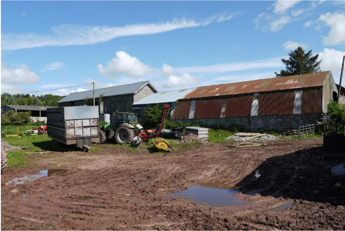
Photo 1. Location for new barns to rear of building on right, looking north
