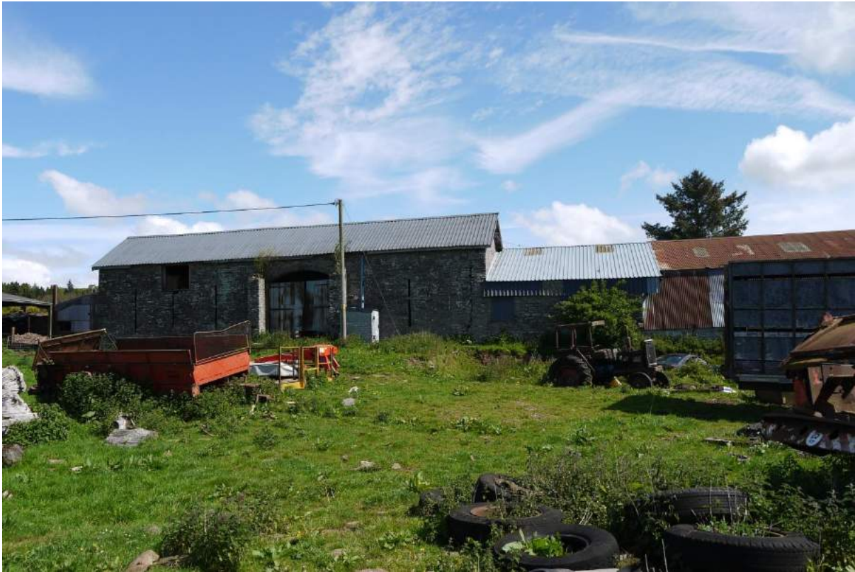
Photo 3. View to north, stone barn range is on the left
