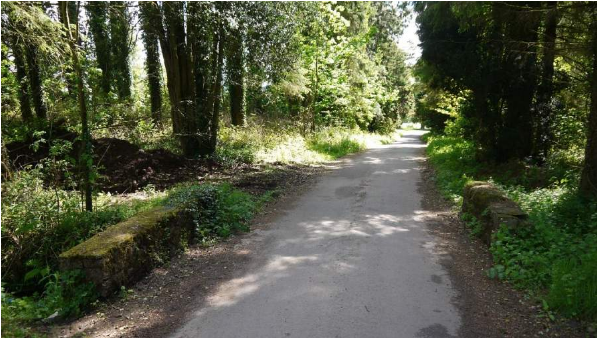
Photo 13. Stone bridge, looking southeast
