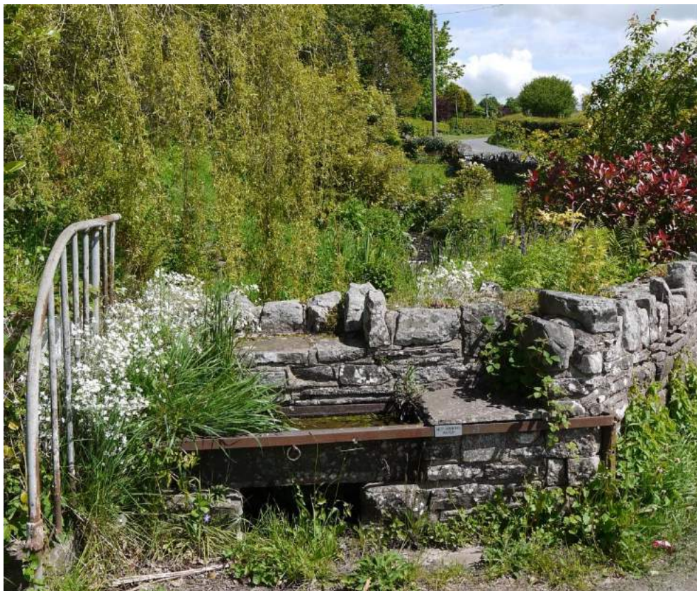
Photo 12. Water trough, looking northeast opposite Smithy
