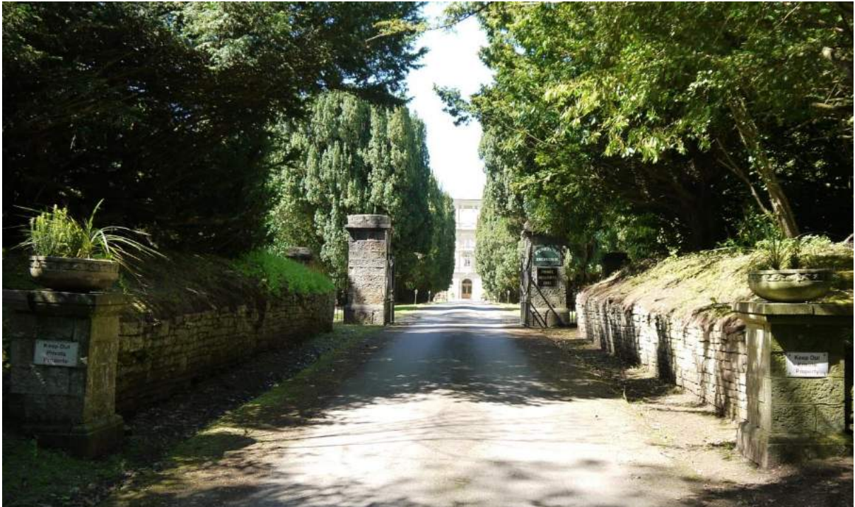
Photo 16. Gate piers and gates looking west to house
