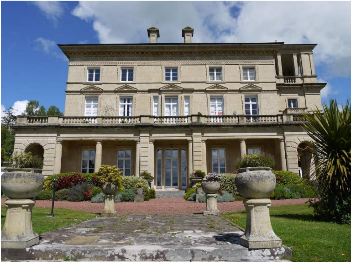
Photo 19. View of southern facade
