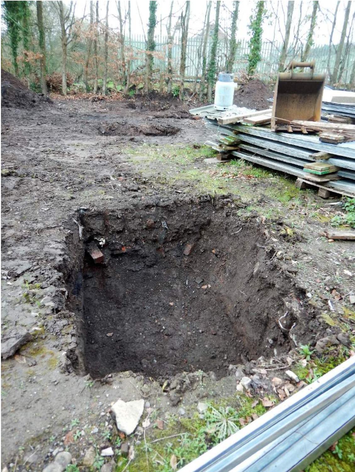
Plate 4: General view of test pits 4, 5 and 6; shot facing SW
