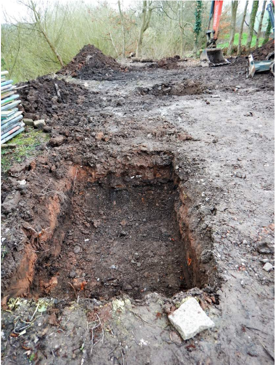
Plate 3: General view of test pits 1, 2 and 3; shot facing SW
