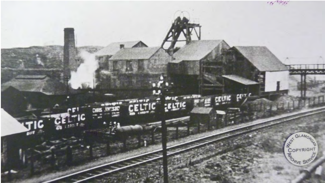
Photo 5: View of Oakwood Colliery (ERM01) from the 1920s, looking southeast. Image courtesy of West Glamorgan Archive Service.
