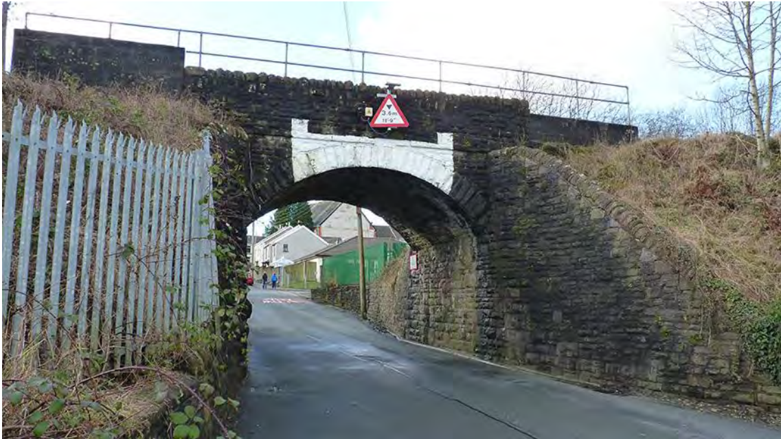
Photo 23: View west of the railway bridge over Ewenny Road.
