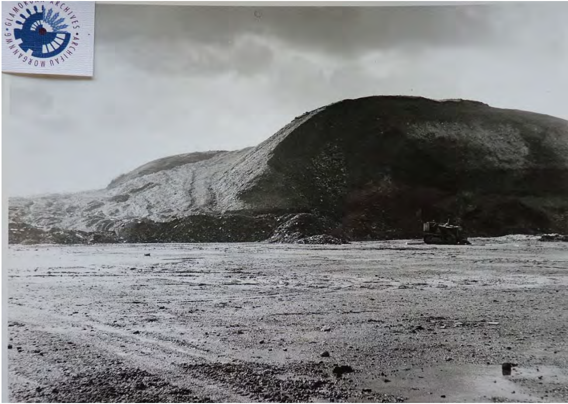
Photo 7: Clearance works landscaping the former Oakwood Colliery tip, demonstrating the large amounts of material that have either been landscaped into or formerly cover the area of proposed development. Image courtesy of Glamorgan Archives.
