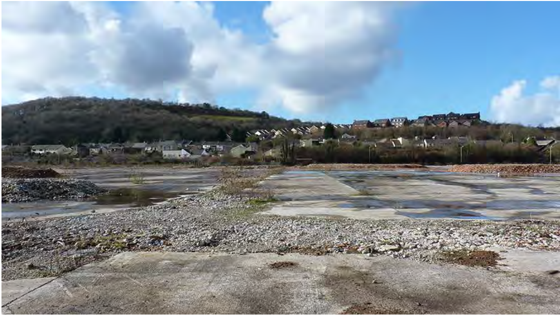
Photo 13: General view looking west across the site.
