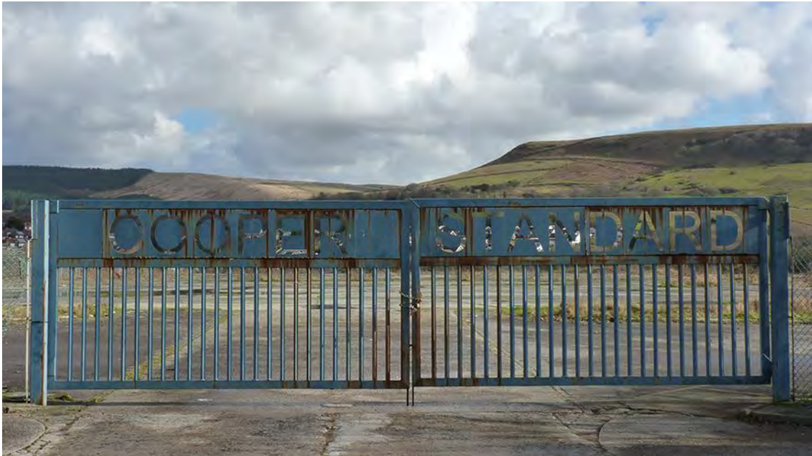
Photo 1: Gated entrance off Oakwood Drive to the former Cooper Standard factory.
