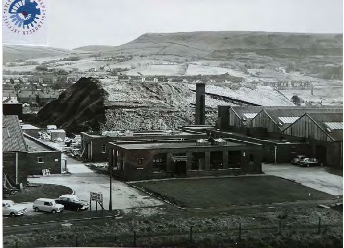
Photo 8: Image from the 1960s looking east across the former factory buildings with remains of the coal tip behind. Image courtesy of Glamorgan Archives.
