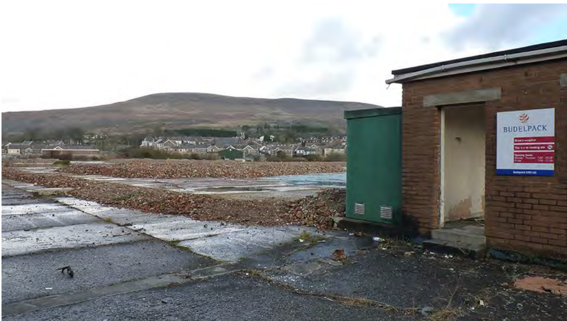
Photo 14: Looking northeast past the only standing building remaining on site.
