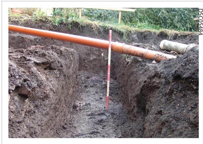
Plate 09: Depth of excavation beneath prepared surface 800mm
