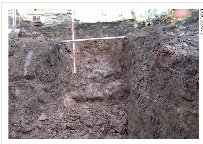
Plate 03: Building foundation under west door. Rubble masonry [116] over [118], no slab, over [114]. In the foreground [113] an isolated line of rounded sandstone boulders
