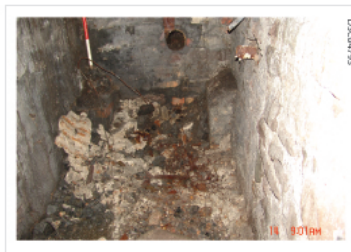
Plate 07: N wall boiler house
