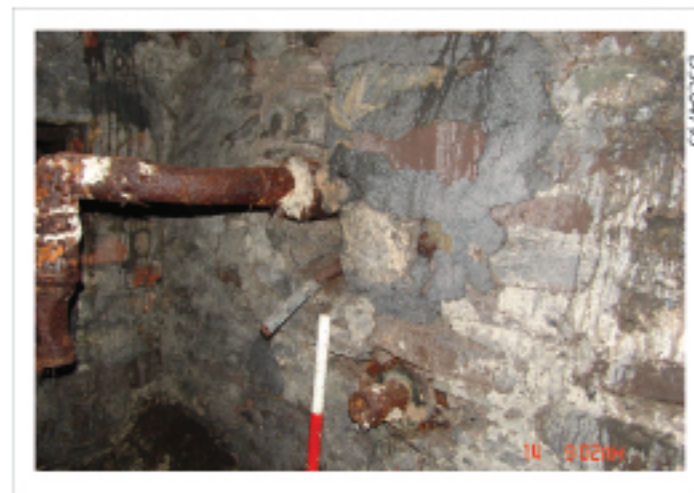
Plate 09: W wall, boiler house. Pies through W wall
