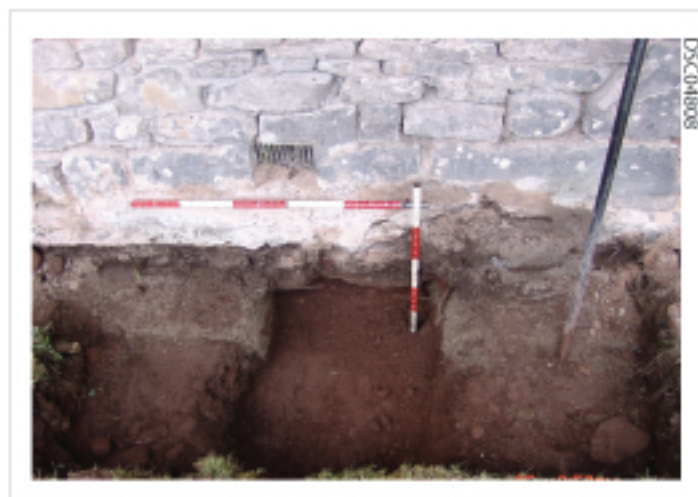
Plate 10: N wall underpinning
