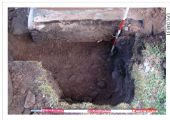
Plate 12: W wall underpinning
