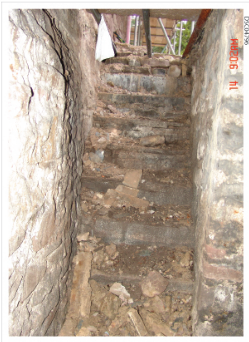
Plate 05: Boiler house stairwell
