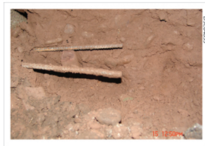
Plate 13: W wall, underpinning and N wall underpinning rebar
