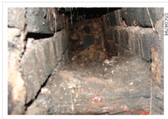
Plate 08: N wall boiler house. Flue duct
