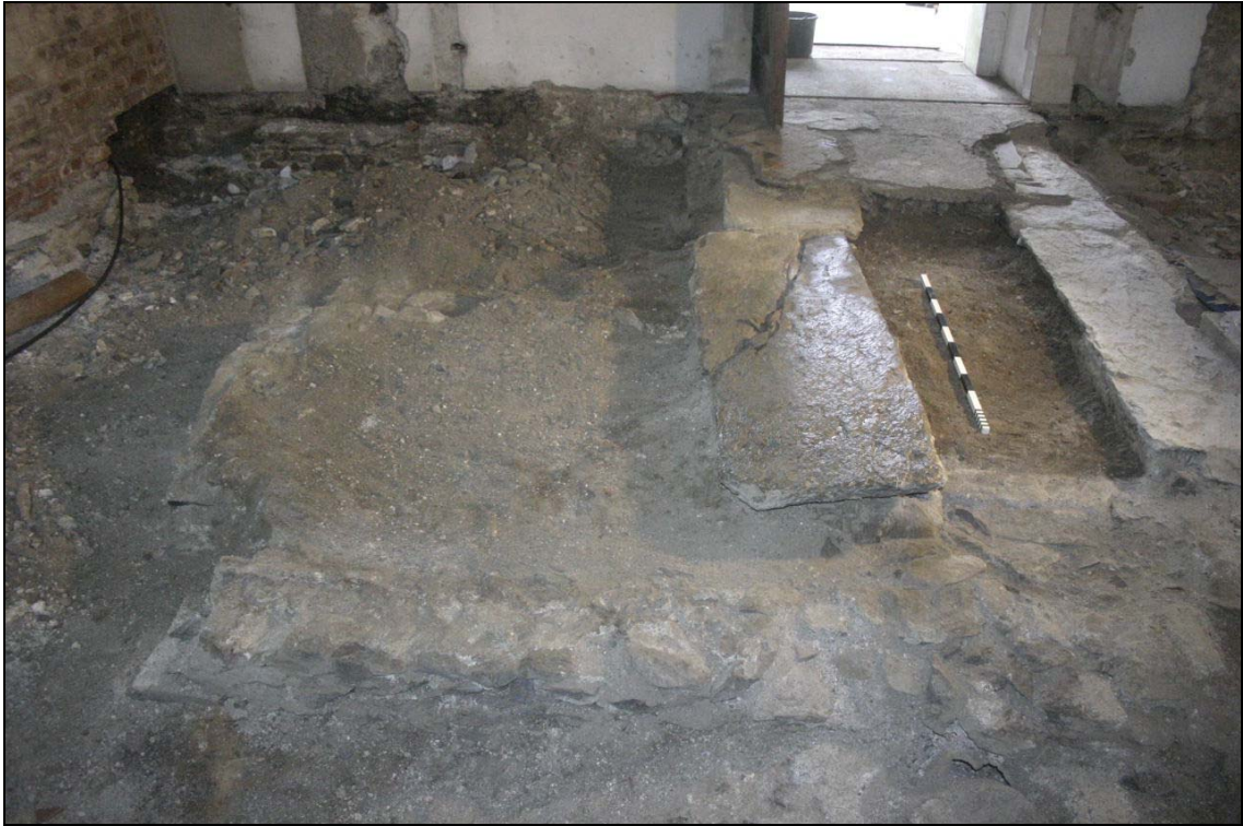
Fig. 3 The re-used grave slabs in the nave as a levelling foundation. 1m scale. Photo CPAT 3805-0003
