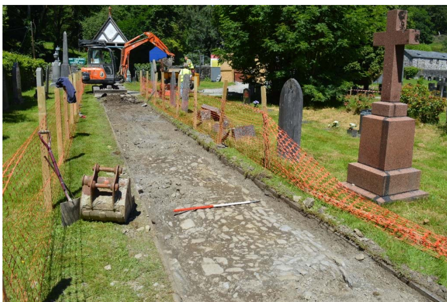
Fig. 19 Cobbled path (52) viewed from the south-east CPAT 3843-0039
