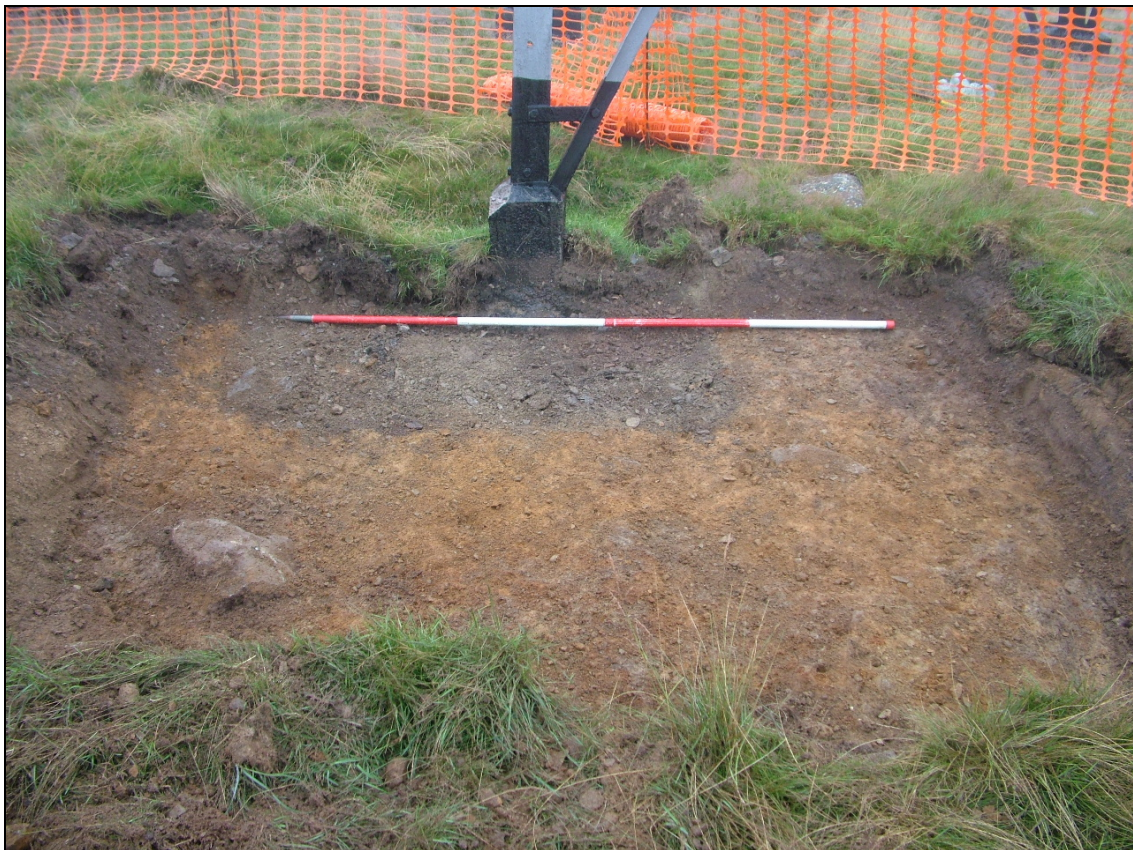
Fig. 3 View of the test excavation area with the west leg of tower AD27 behind; the backfill of the foundation excavation is clearly visible. Photo CPAT 3656-0025
