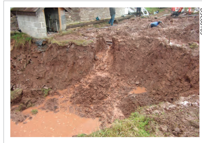
Plate 10: Overview of bank removal
