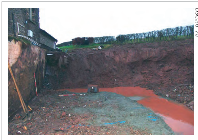
Plate 07: West retaining wall with footings 1 & 2
