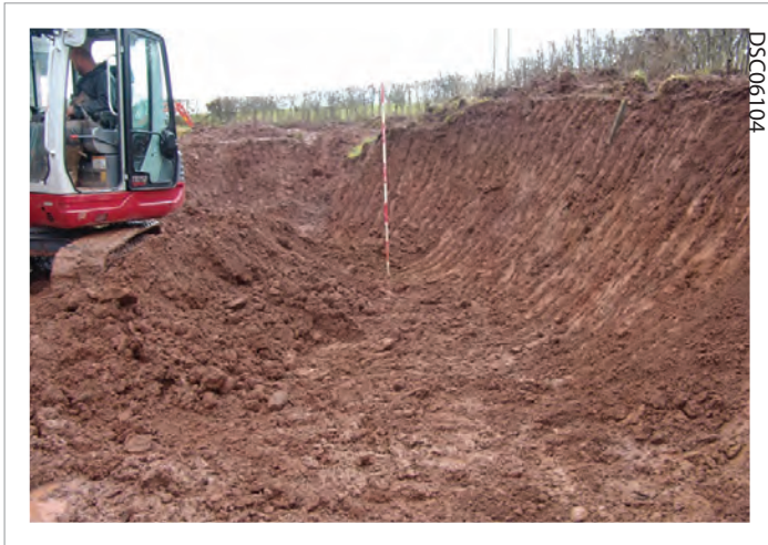
Plate 09: Extent of bank removal, final
