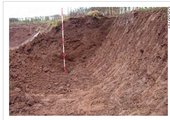
Plate 08: Extent of bank removal
