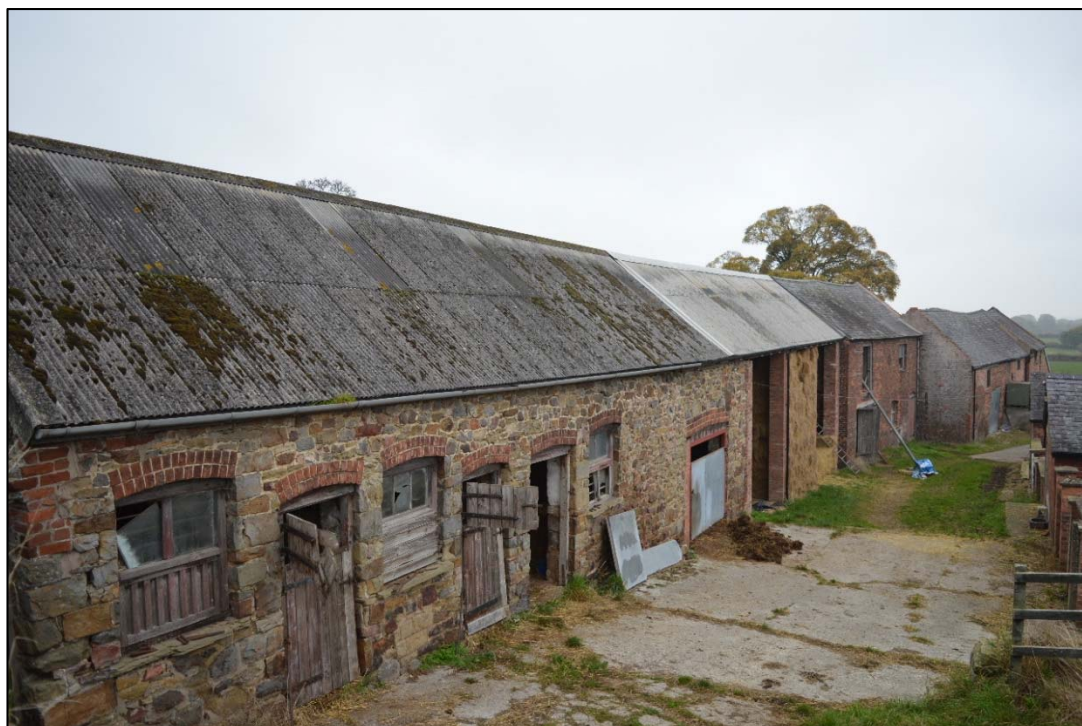
Fig. 12: The main historic range of farm buildings on the north side of the farmyard, from the west-south-west (CPAT 4245-0003)
