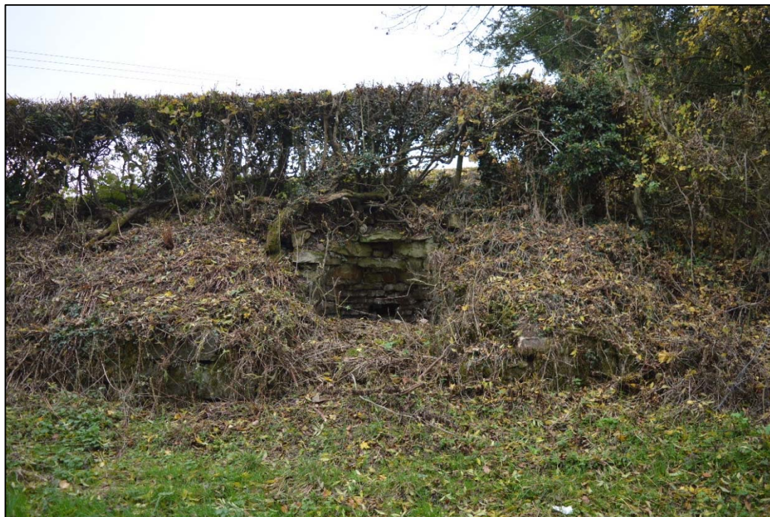
Fig. 11: The Cadwgan Hall limekiln, viewed from the road to its north (CPAT 4245-0013)
