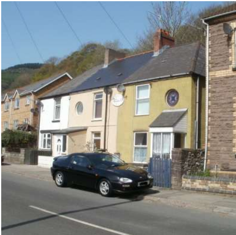
Figure 7: the former Zoar Chapel Risca, now three private houses (© Robert Jeffrey Southall)
