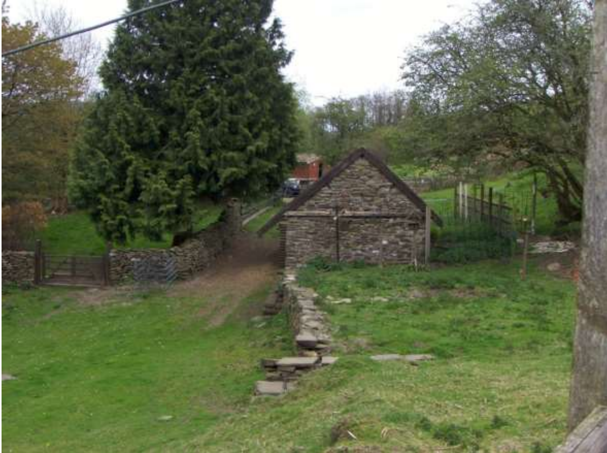
Figure 14: Renovated outbuilding in the yard opposite the house (© Robert Jeffrey Southall)
