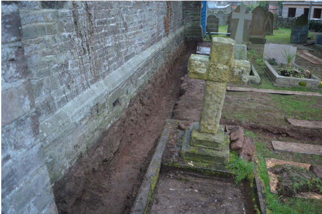
Fig. 3 Trench section along the north side of the nave CPAT 4308-0008
