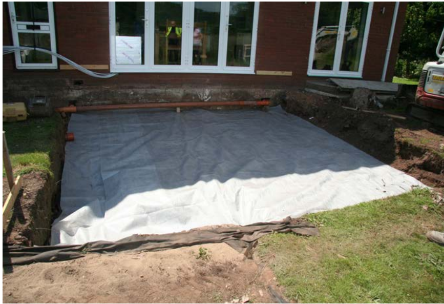
Geotextile over foundation trench (looking east)
