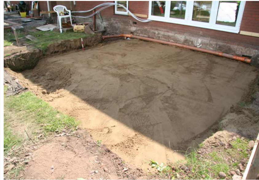
Sand cover over geotextile within foundation trench (looking south-east)
