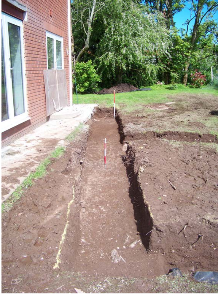
Trench 2 and 3: Looking north-northwest
