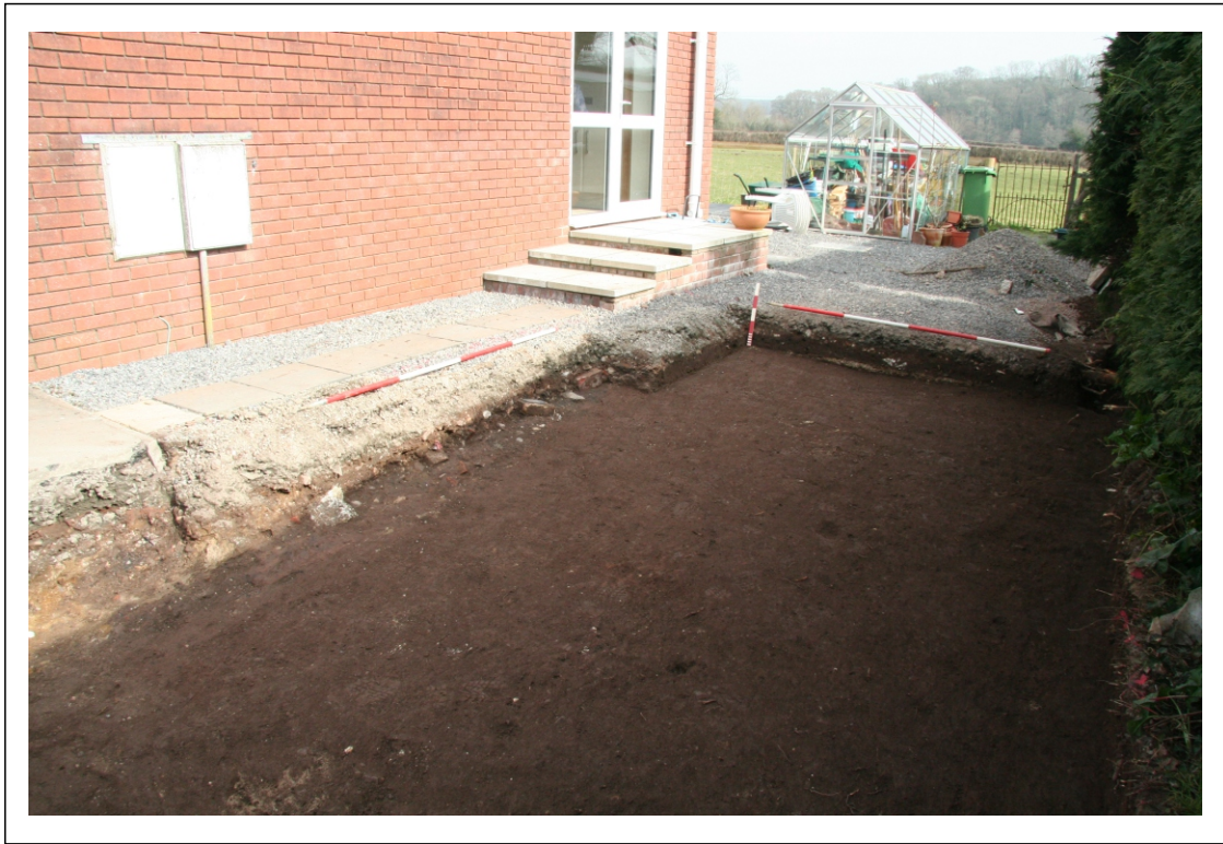
Plate 3: View north of evaluation trench sections
