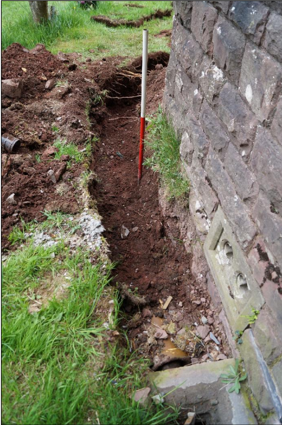
Plate 15: ASG2018_115, Southeast end of Trench 2 adjacent to the church, showing the ceramic drain pipe which was broken and silted-up, looking west southwest.
