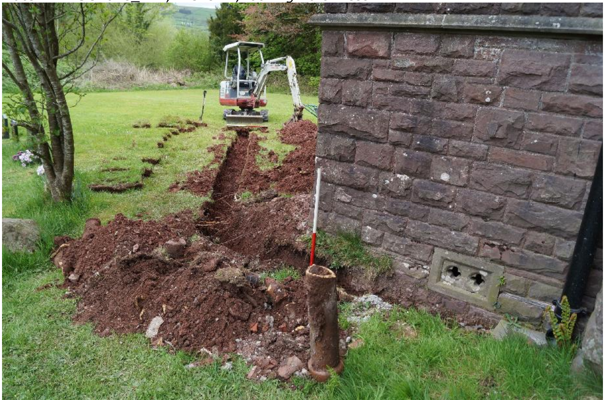
Plate 18: ASG2018_118, Trench 2 with silted-up , broken drainpipe, looking northwest.
