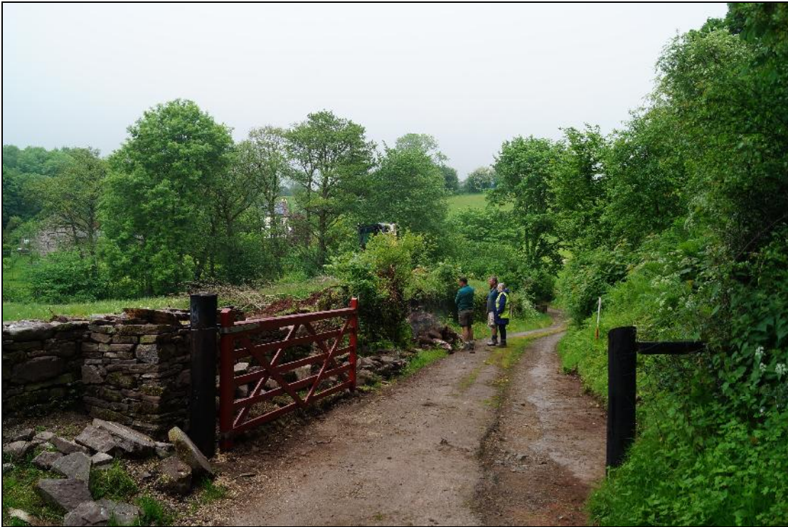
Plate 15: SEL2018_115, General view showing the western section to the east of the gate and the short wall at right angles, both reconstructed, looking east-northeast
