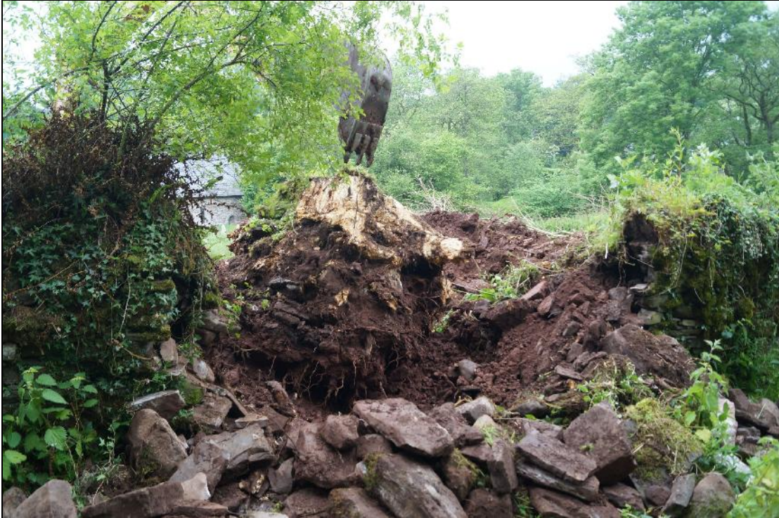
Plate 17: SEL2018_117, Removing the tree bole, looking northeast.
