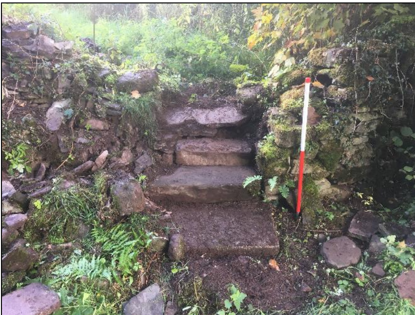
Plate 26: SEL2018_126, The steps through the eastern end of the section E after cleaning of vegetation and soil, looking north.
