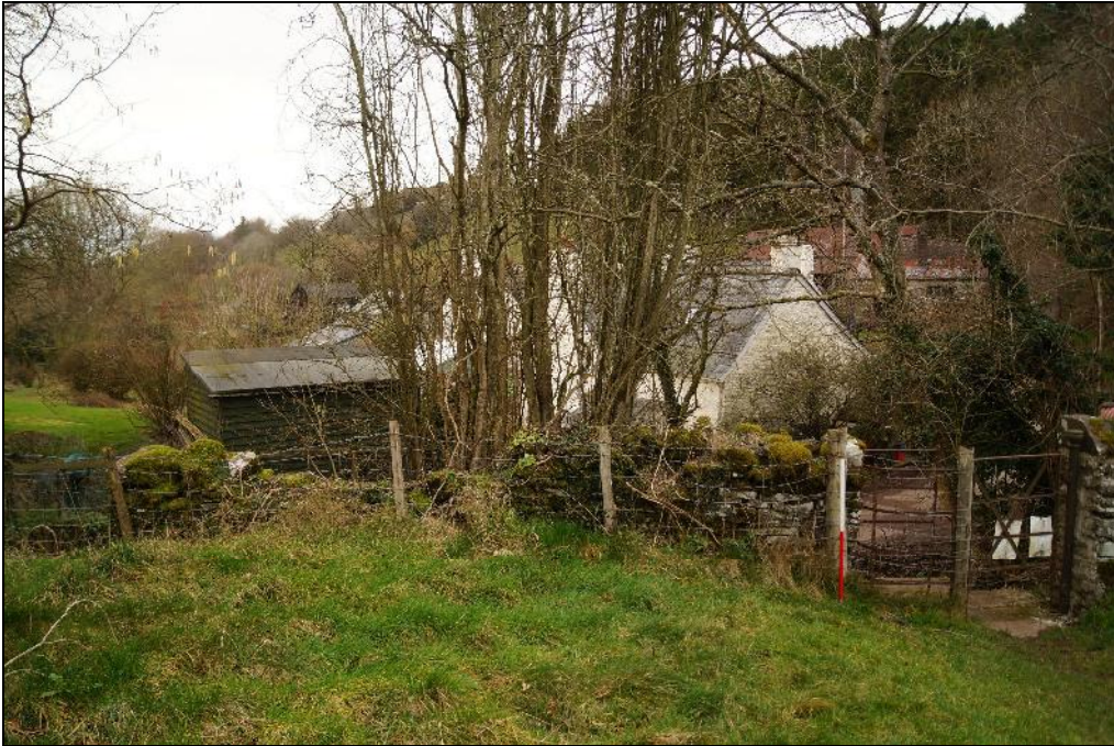
Plate 35: SEL2018_135, Section of the western boundary wall just to the south of the gateway, looking northwest.
