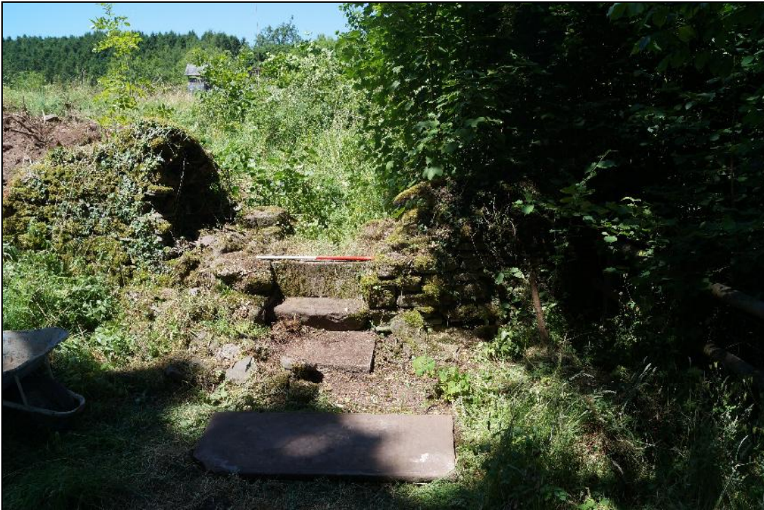
Plate 22: SEL2018_122, The former steps through the eastern end of the southern boundary wall. The large slab, found to be a grave slab, was originally the top step in the wall line, looking north-northwest.
