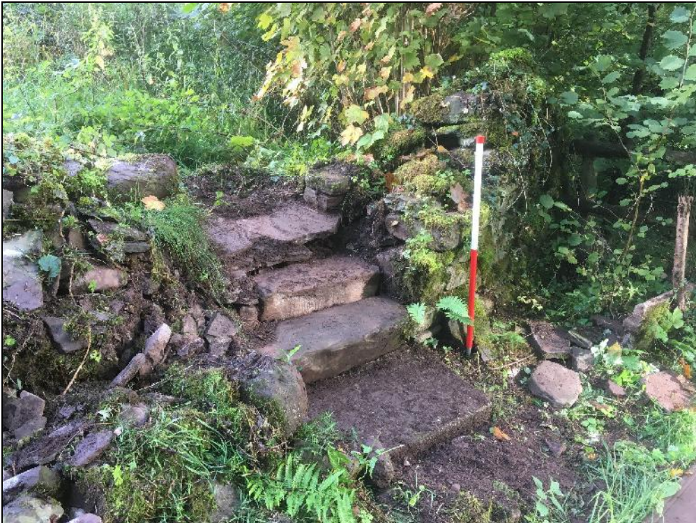
Plate 27: SEL2018_127, The steps through the eastern end of the section E after cleaning of vegetation and soil, looking northeast.
