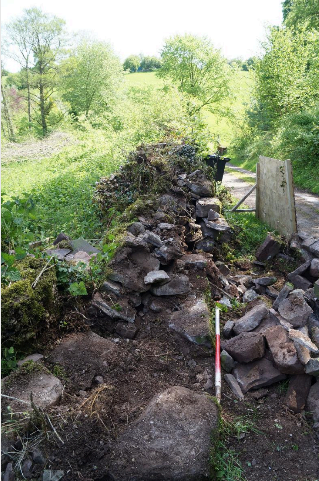
Plate 13: SEL2018_113, Next section of wall dismantled, looking east.
