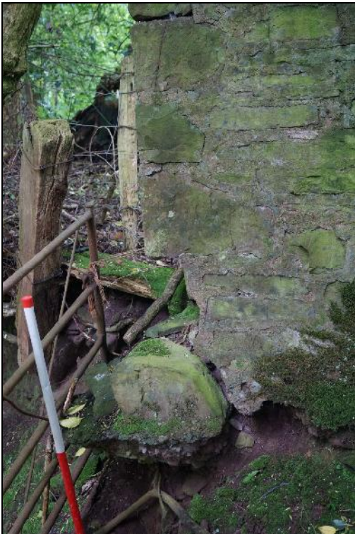
Plate 34: SEL2018_134, The base of the northern end of the northwest wall, RV Williams Drawing number 3892/07, note 8. Underpinning previously attempted, looking east-northeast.
