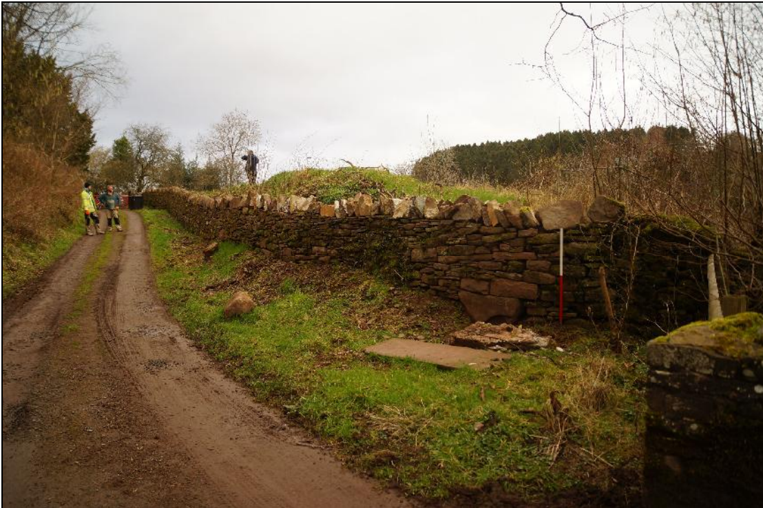
Plate 33: SEL2018_133, Completed restoration of the southern boundary wall, looking west.
