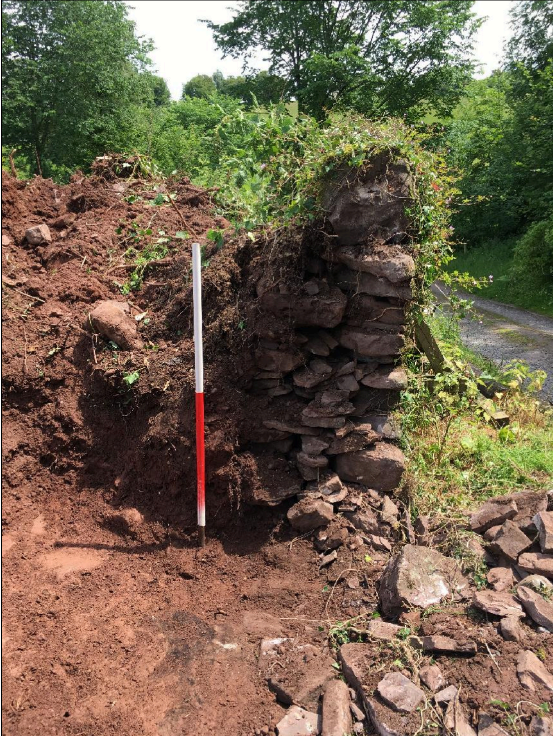
Plate 19: SEL2018_119, Tree bole and roots removed and section through wall and earth behind excavated, looking east.
