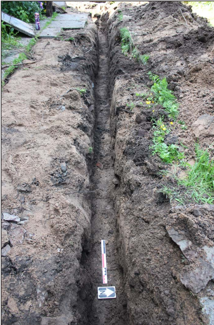
Plate 23: Trench E, from the east. Scale 0.3m.
