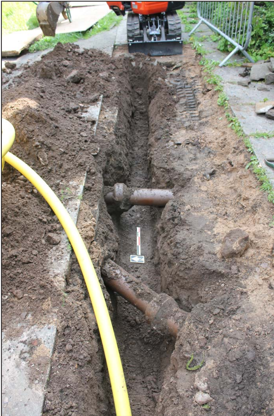
Plate 28: Trench F, from the west. Scale 0.3m.
