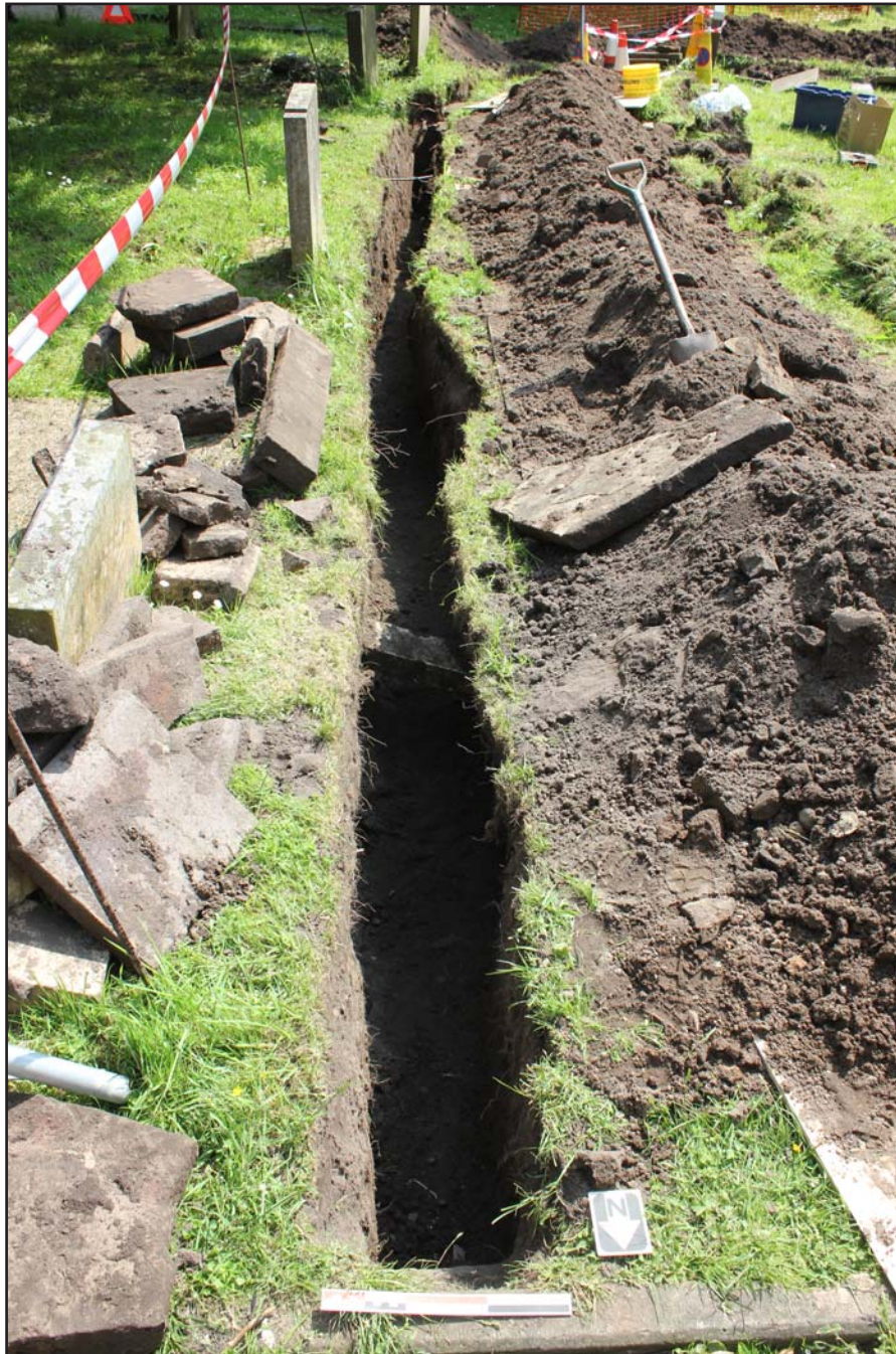
Plate 15: Trench C, from the north. Scale 0.3m.
