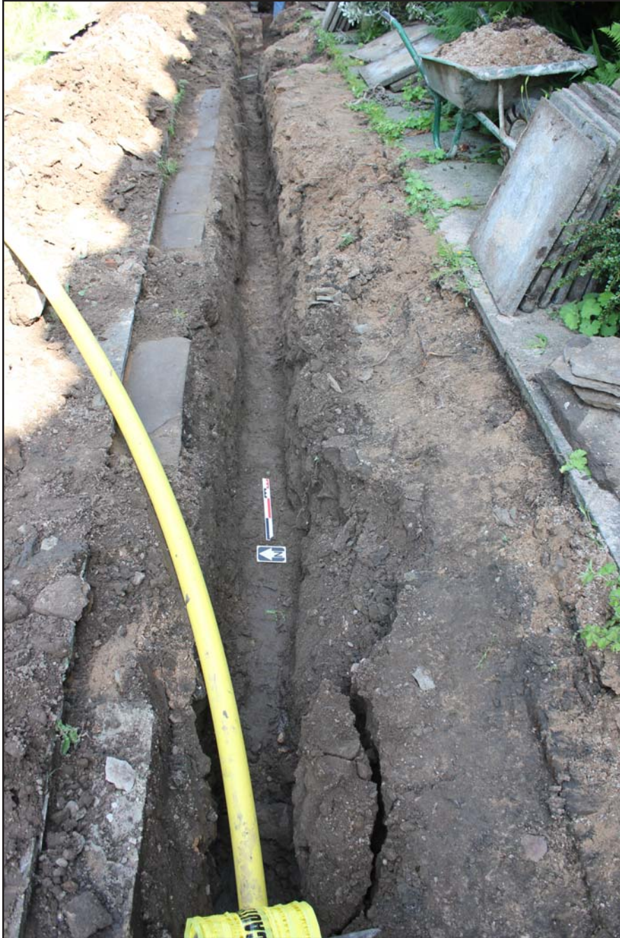
Plate 29: Trench G showing remnants of (1009), from the west. Scale 0.3m.
