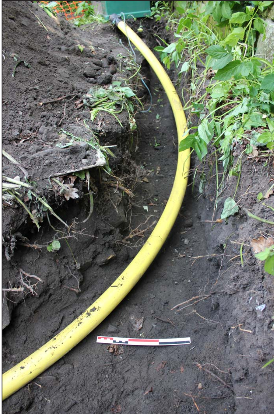
Plate 01: Trench A (east-west section) post excavation, from the west. Scale 0.3m.
