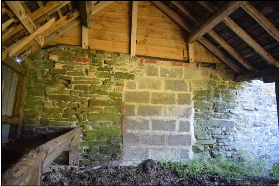
Fig. 6 Cart shed, viewed from the west showing infilled later doorway into cowshed Photo CPAT 4942-015
