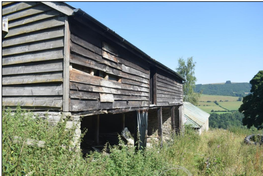
Fig. 3 Cart shed, viewed from the south Photo CPAT 4942-018
