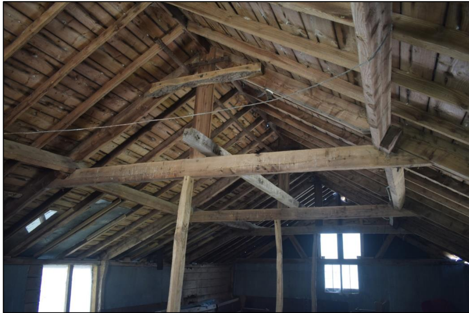
Fig. 8 Intermediate king post roof truss within the cart shed Photo CPAT 4942-029
