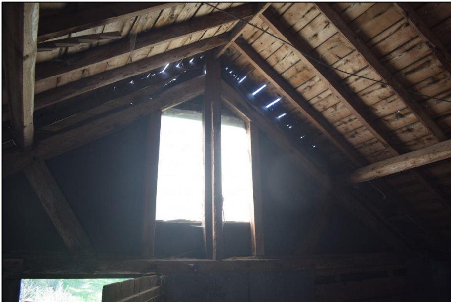
Fig. 7 Compound truss on south gable end of cart shed Photo CPAT 4942-033
