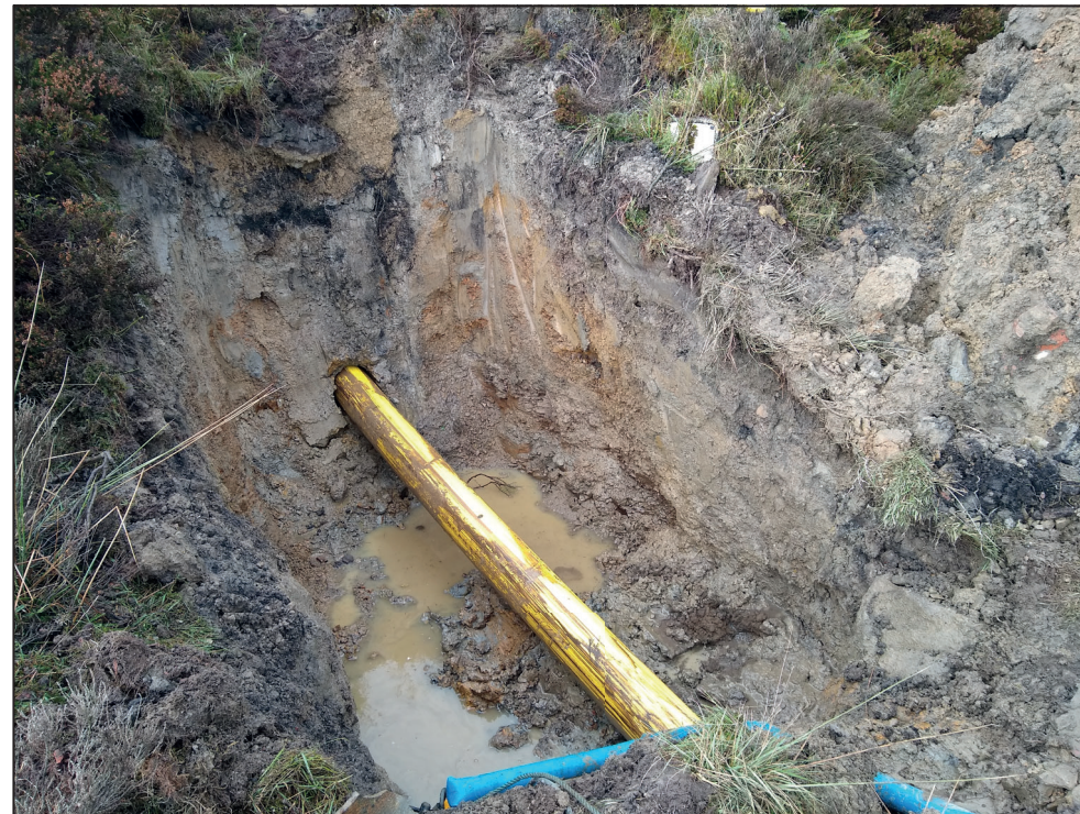
Trench 5, working shot
