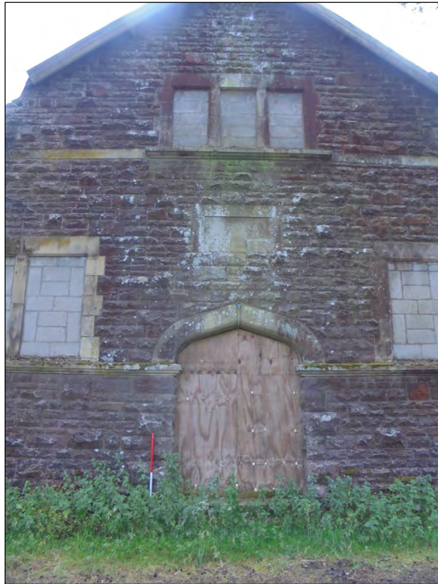
Photo 5 Detail of main elevation of building A
