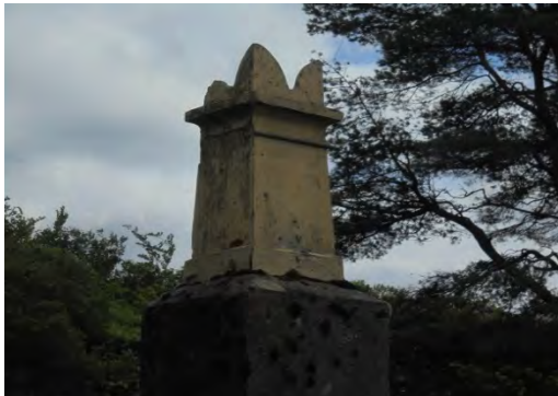
Photo 12 Reservoir Keeper's Cottage (C) detail of chimney
