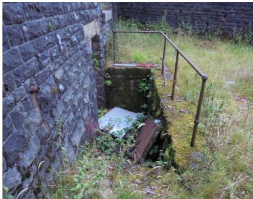
Photo 9 Staircase to basement
