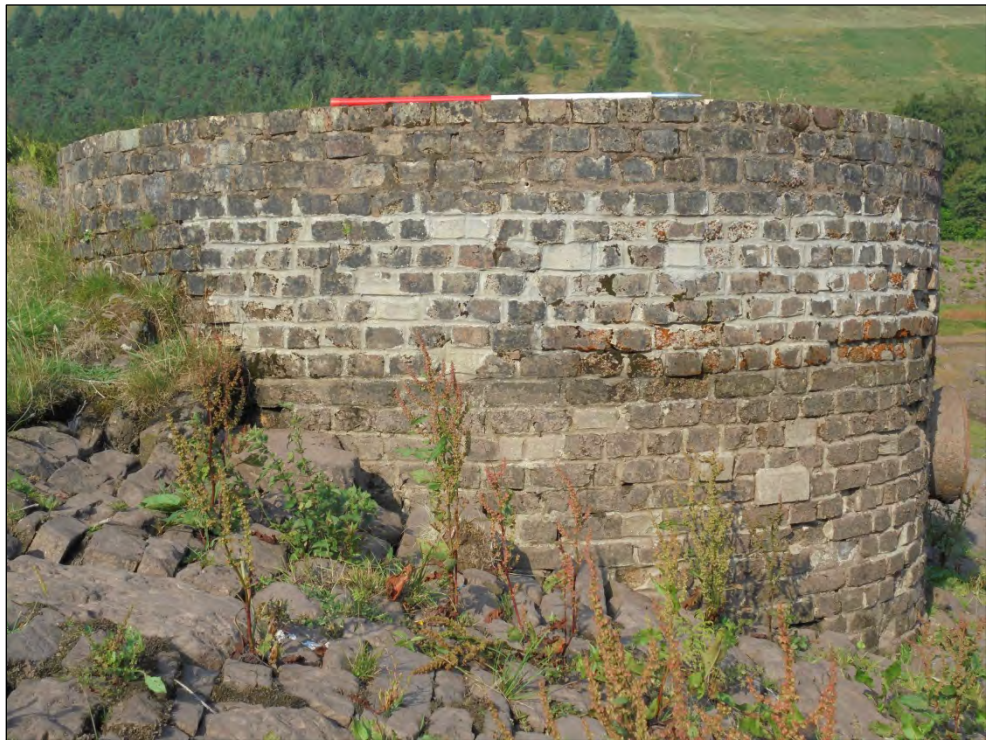
Photo 22 Valve Tower (E) facing west
