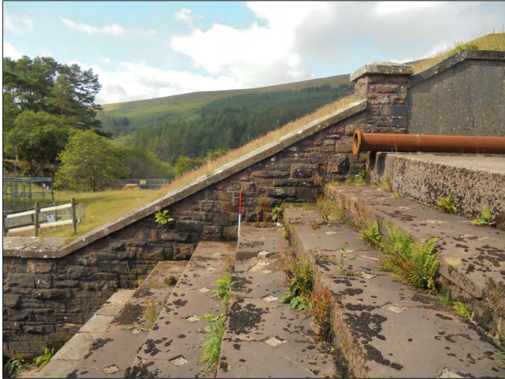
Photo 27 Spillway (G) detail of byewash facing south-west
