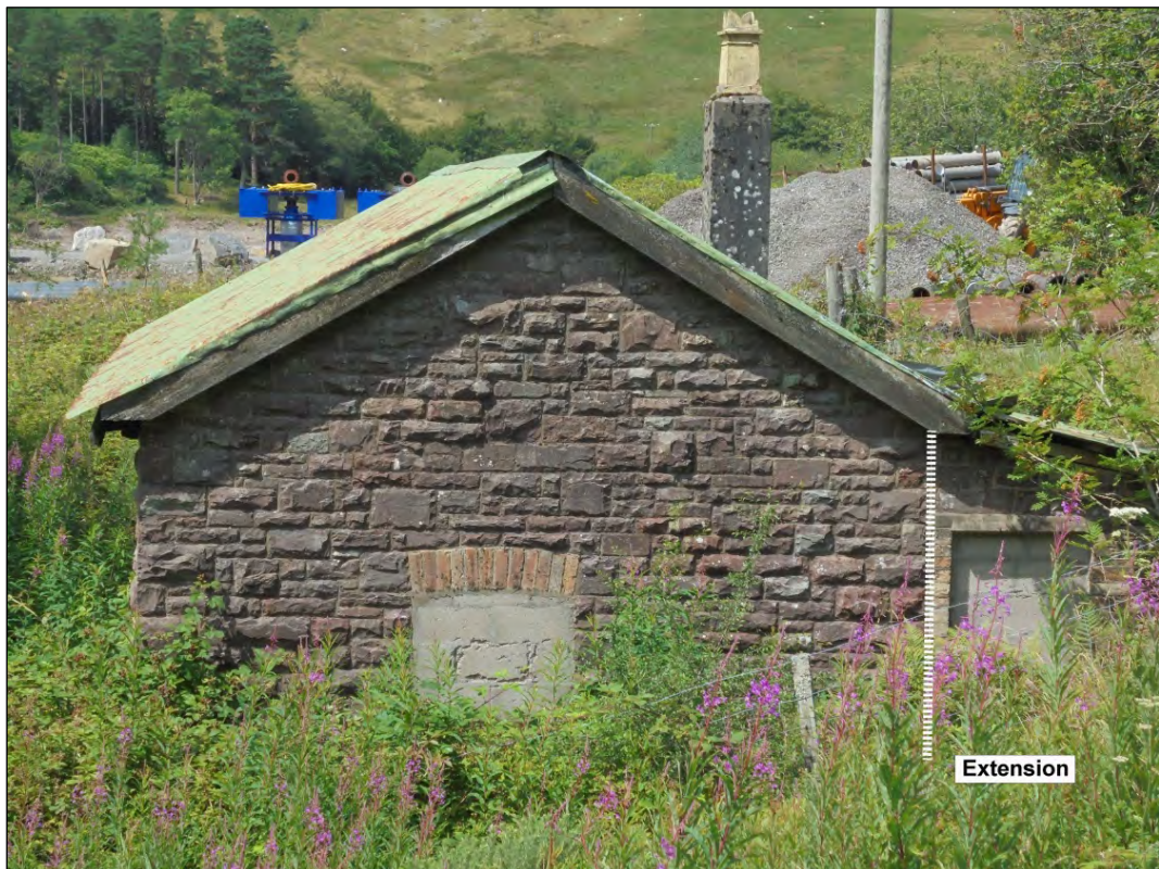
Photo 14 Reservoir Keeper's Cottage (C) west facing elevation
