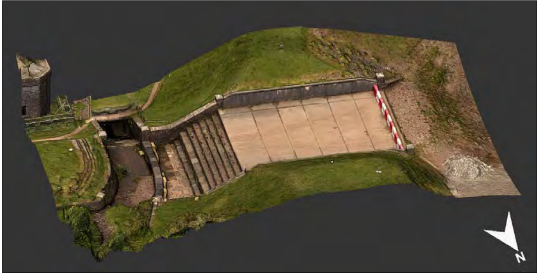
Fig. 23 Structure G (spillway) photogrammetric model
