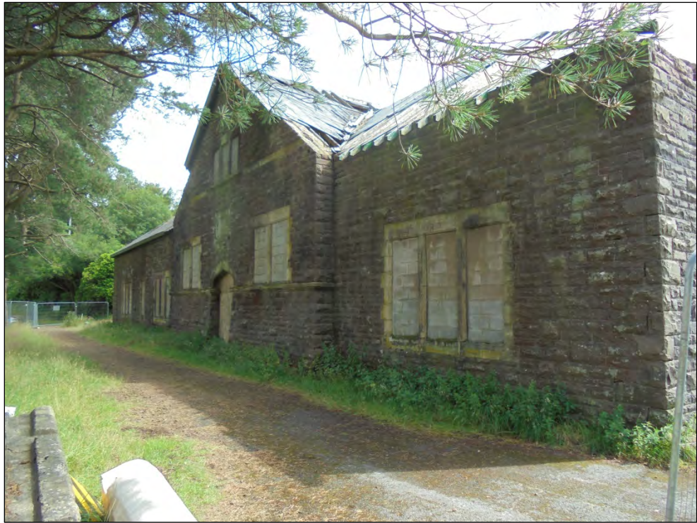
Photo 1 Filter House (A) main elevation
