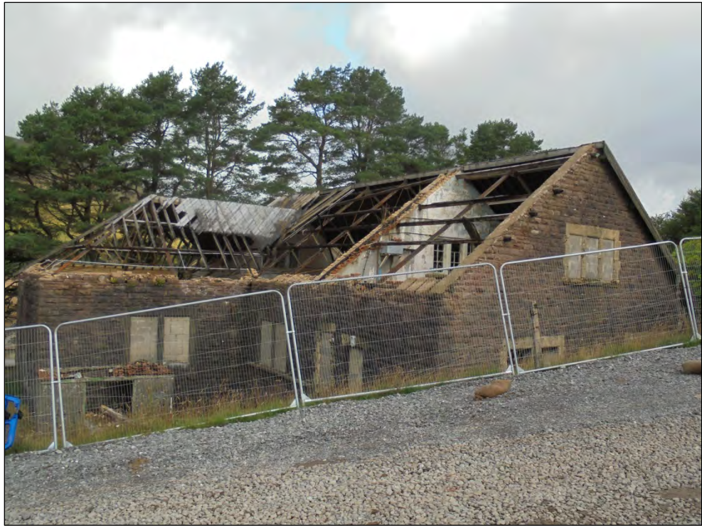
Photo 3 Filter House (A) south and south-east facing elevations
