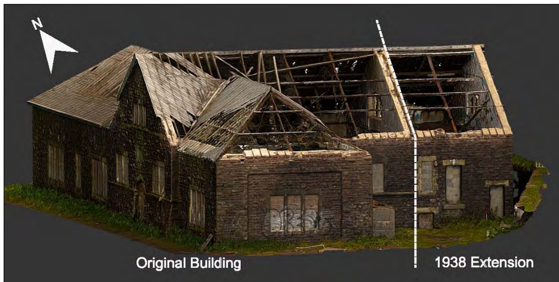
Fig. 13 Photogrammetric model of Building A and Extension B
