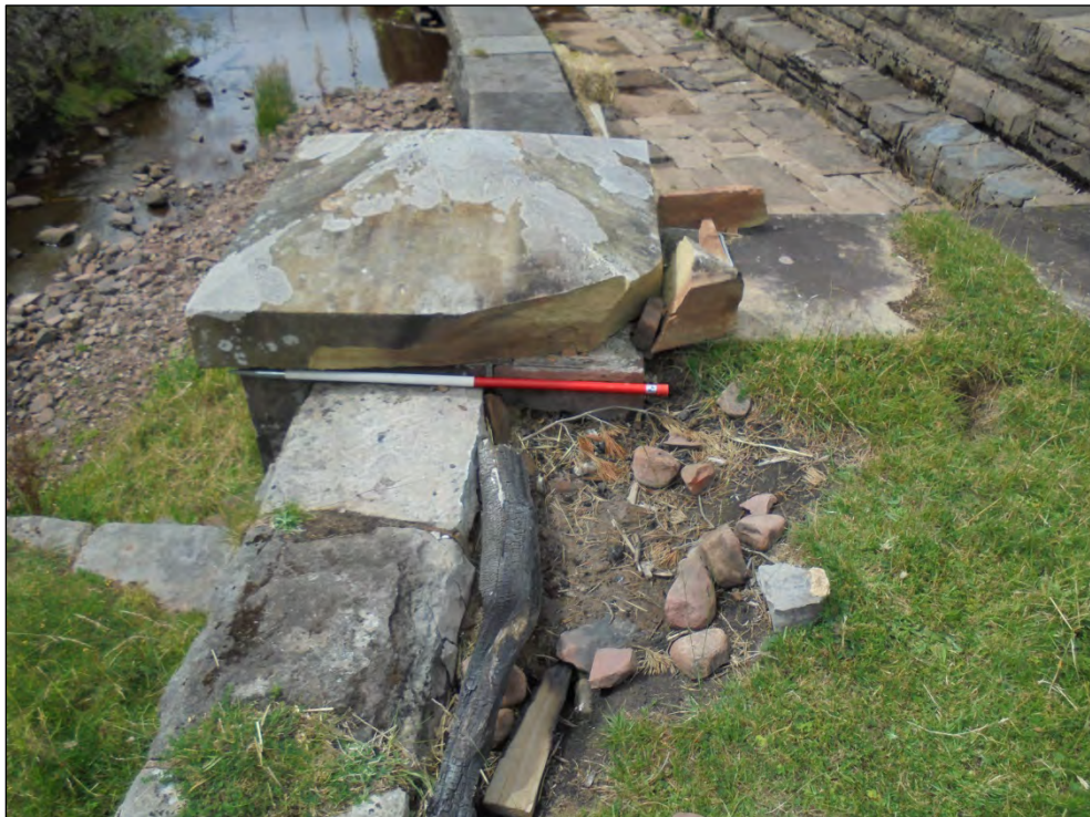
Photo 28 Spillway (G) detail of pier and wall
