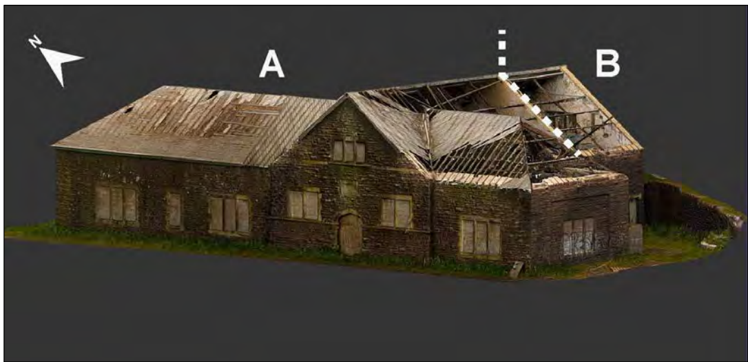
Fig. 12 Filter House (A) and Extension (B) photogrammetric model
