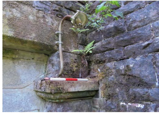
Photo 8 Detail of fixture on north-east facing elevation
