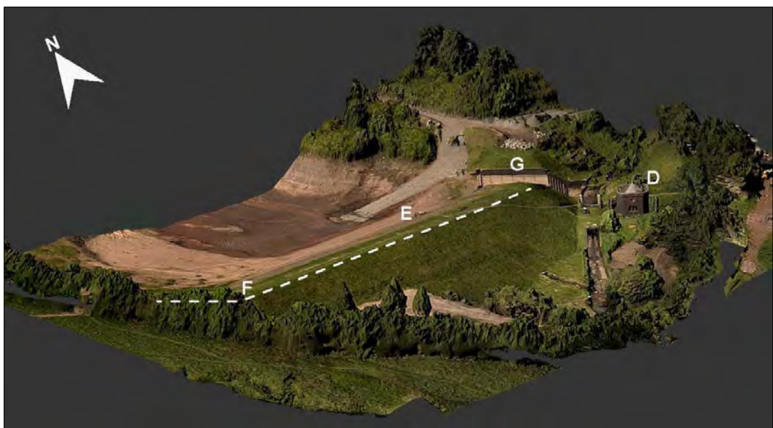
Fig. 21 Dam (F) photogrammetric model facing north-east
