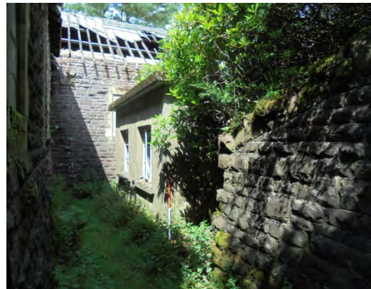
Photo 10 Small extension (B1) to the north
