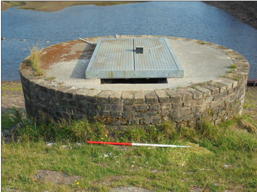
Photo 21 Valve Tower (E) facing north
