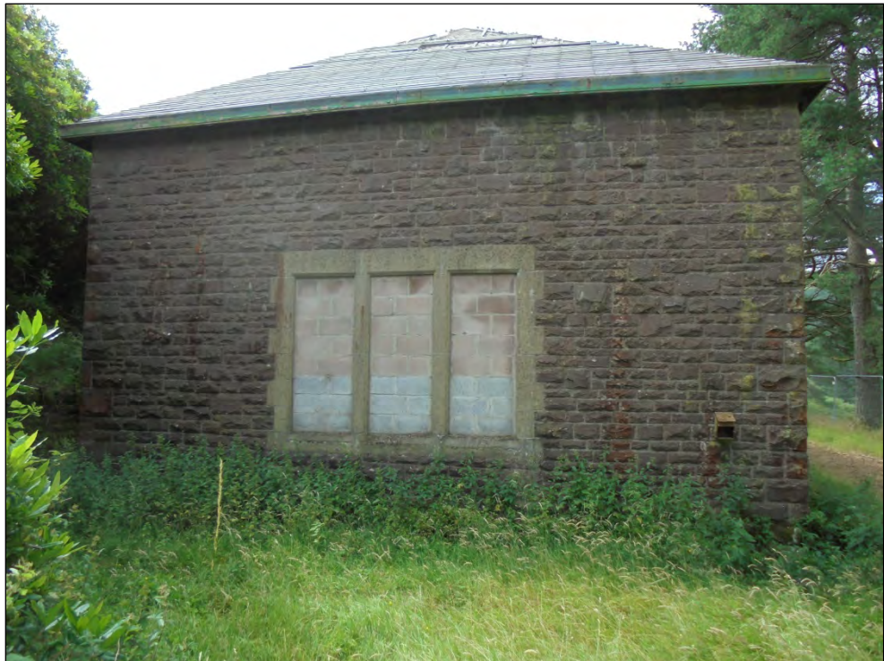
Photo 4 Filter House (A) north facing elevation
