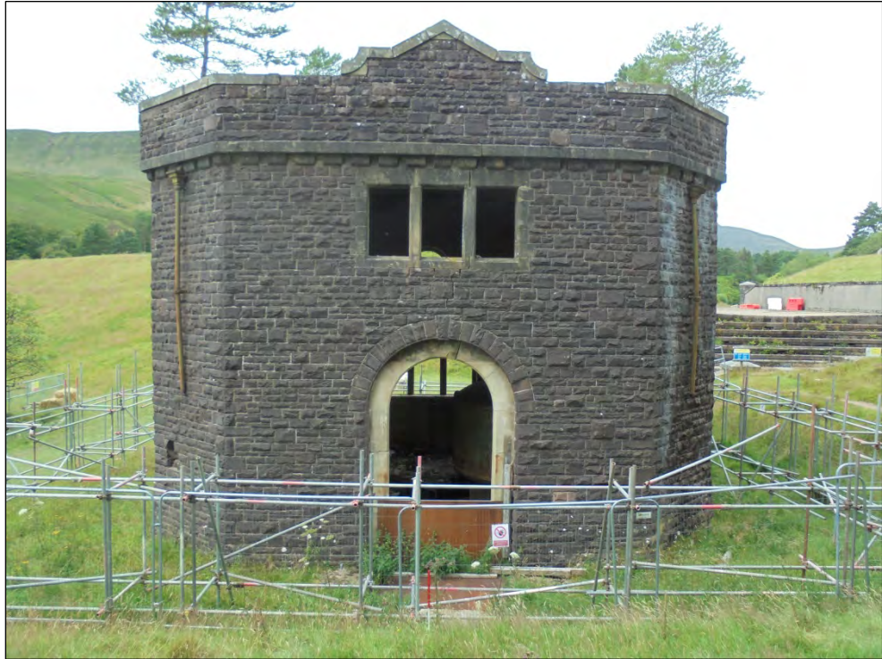
Photo 15 Grade II Listed Old Filter House (D) south-east facing elevation
