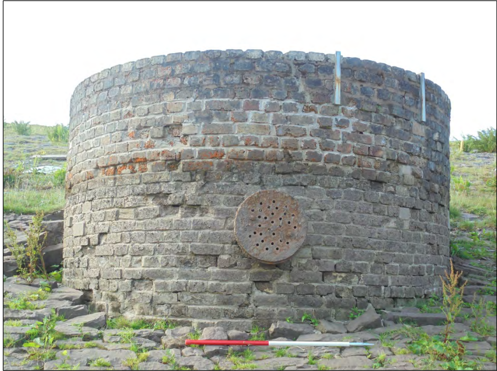
Photo 23 Valve Tower (E) facing south
