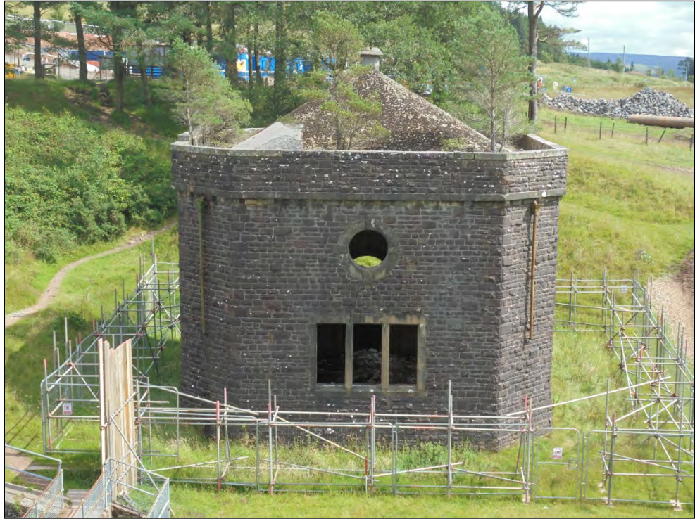
Photo 17 Grade II Listed Old Filter House (D) north-west facing elevation
