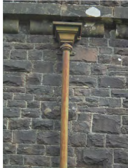
Photo 20 Detail of cast iron drain pipe and hopper
