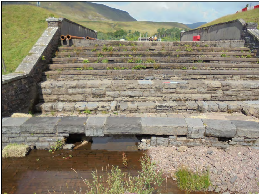
Photo 30 Spillway (G) facing north-west
