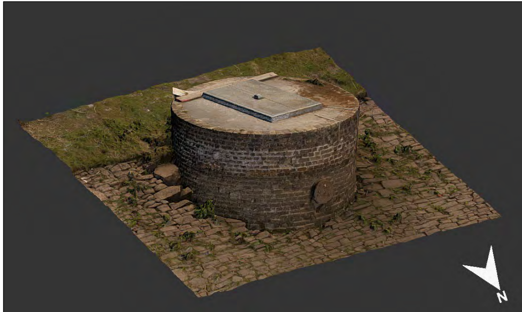
Fig. 18 Valve Tower (E) photogrammetric model
