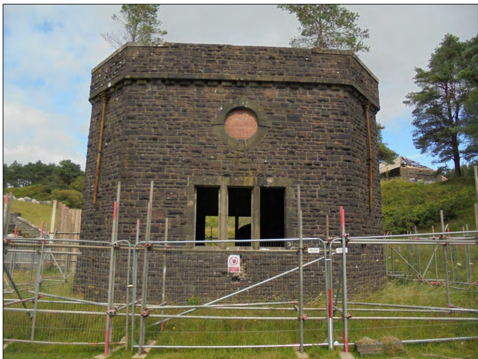
Photo 16 Grade II Listed Old Filter House (D) south facing elevation
