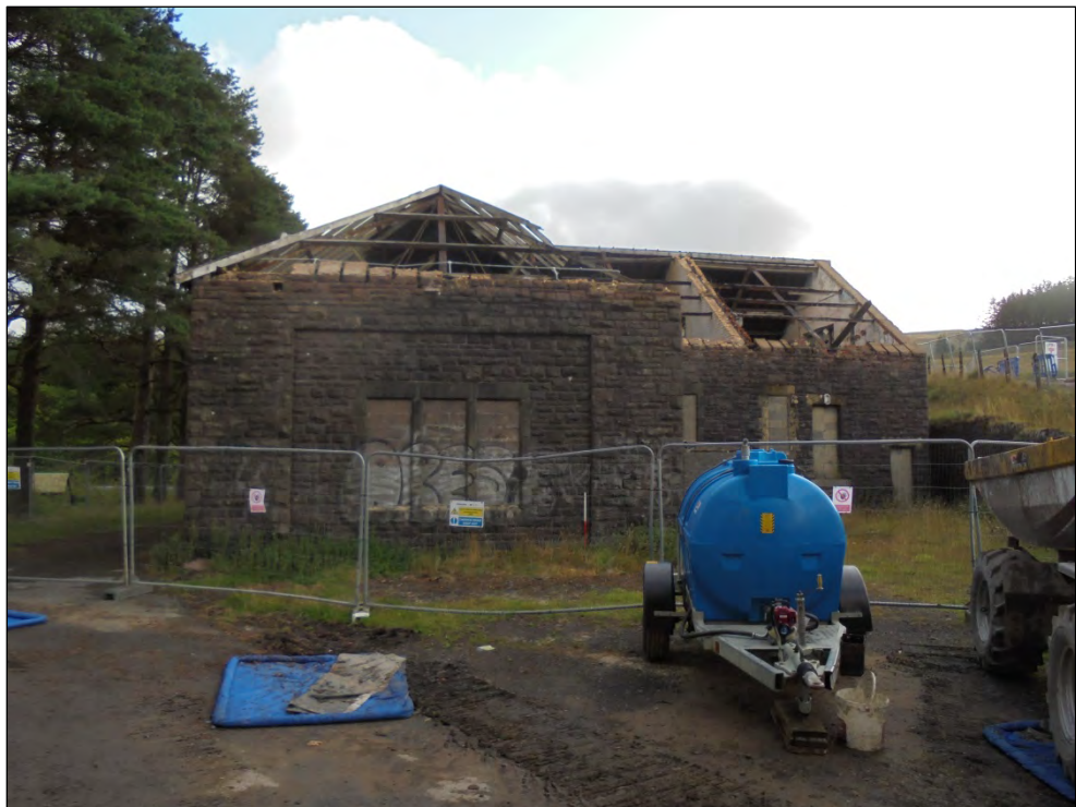
Photo 2 Filter House (A) south facing elevation
