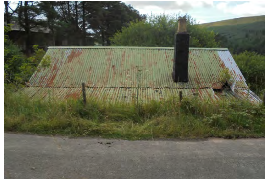
Photo 13 Reservoir Keeper's Cottage (C) north facing elevation
