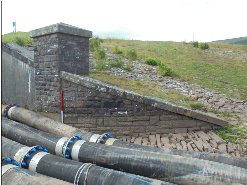
Photo 26 Spillway (G) detail of wall and pavement facing south
