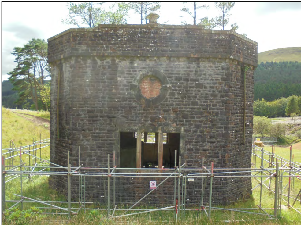
Photo 18 Grade II Listed Old Filter House (D) north-east facing elevation
