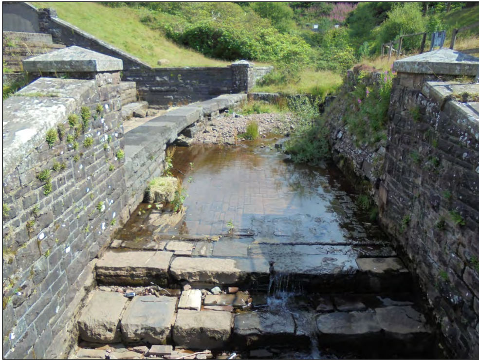
Photo 29 Spillway (G) facing north-east
