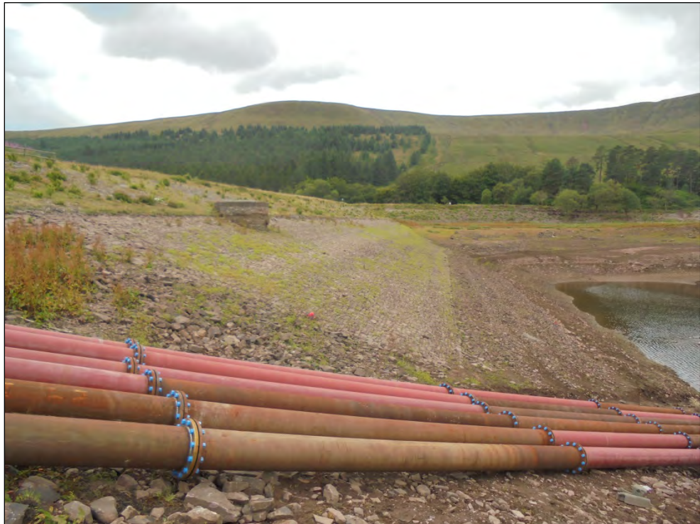
Photo 24 Dam (F) facing west
