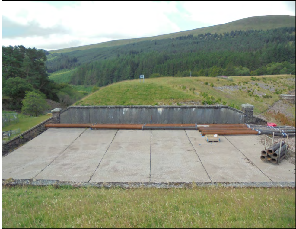
Photo 25 Spillway (G) facing south-west
