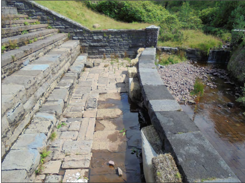
Photo 31 Spillway (G) facing north-east
