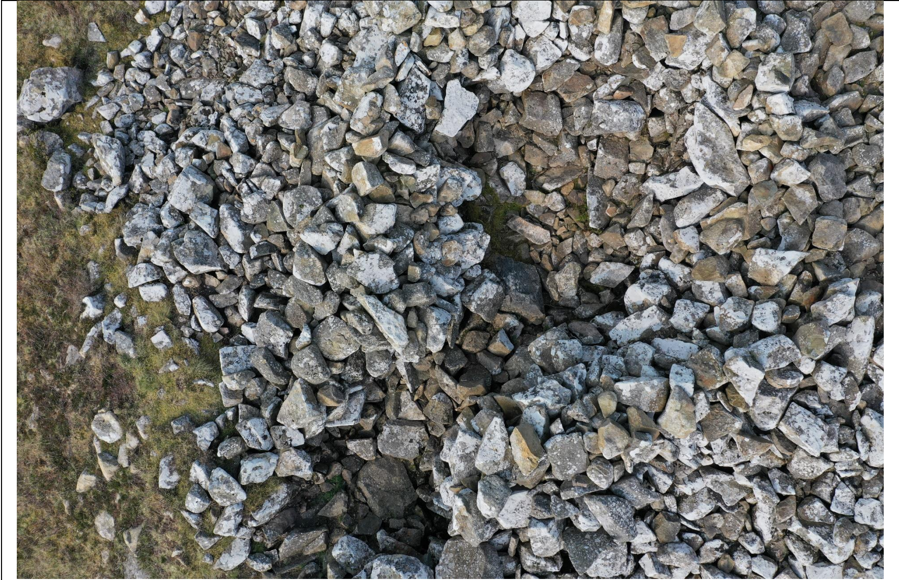
Figure 12. Aerial view of rim and depression prior to reconsolidation work.
