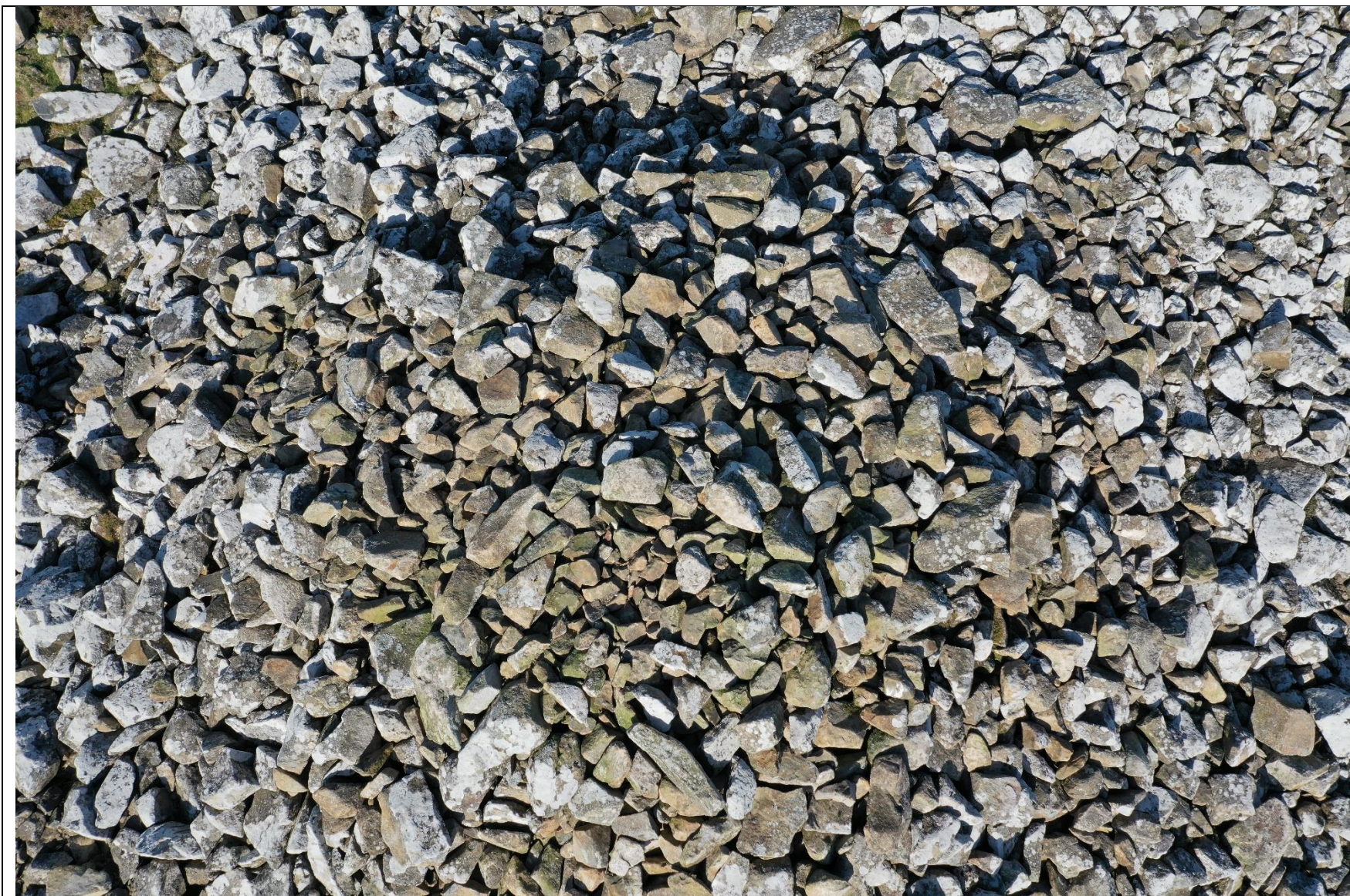
Figure 11. Aerial view of peak after reconsolidation work.
