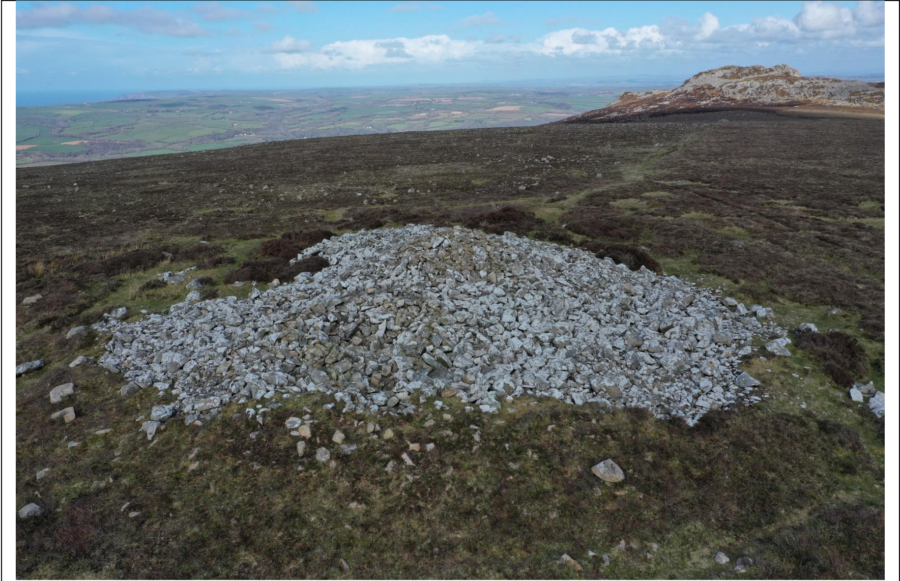
Figure 9. Monument towards north after reconsolidation work.
