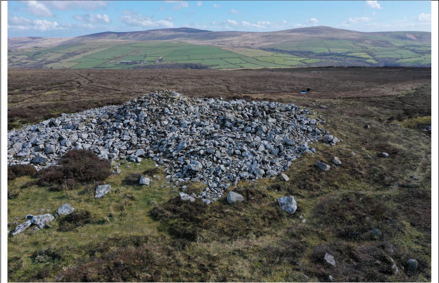
Figure 3. Monument towards south after reconsolidation work.
