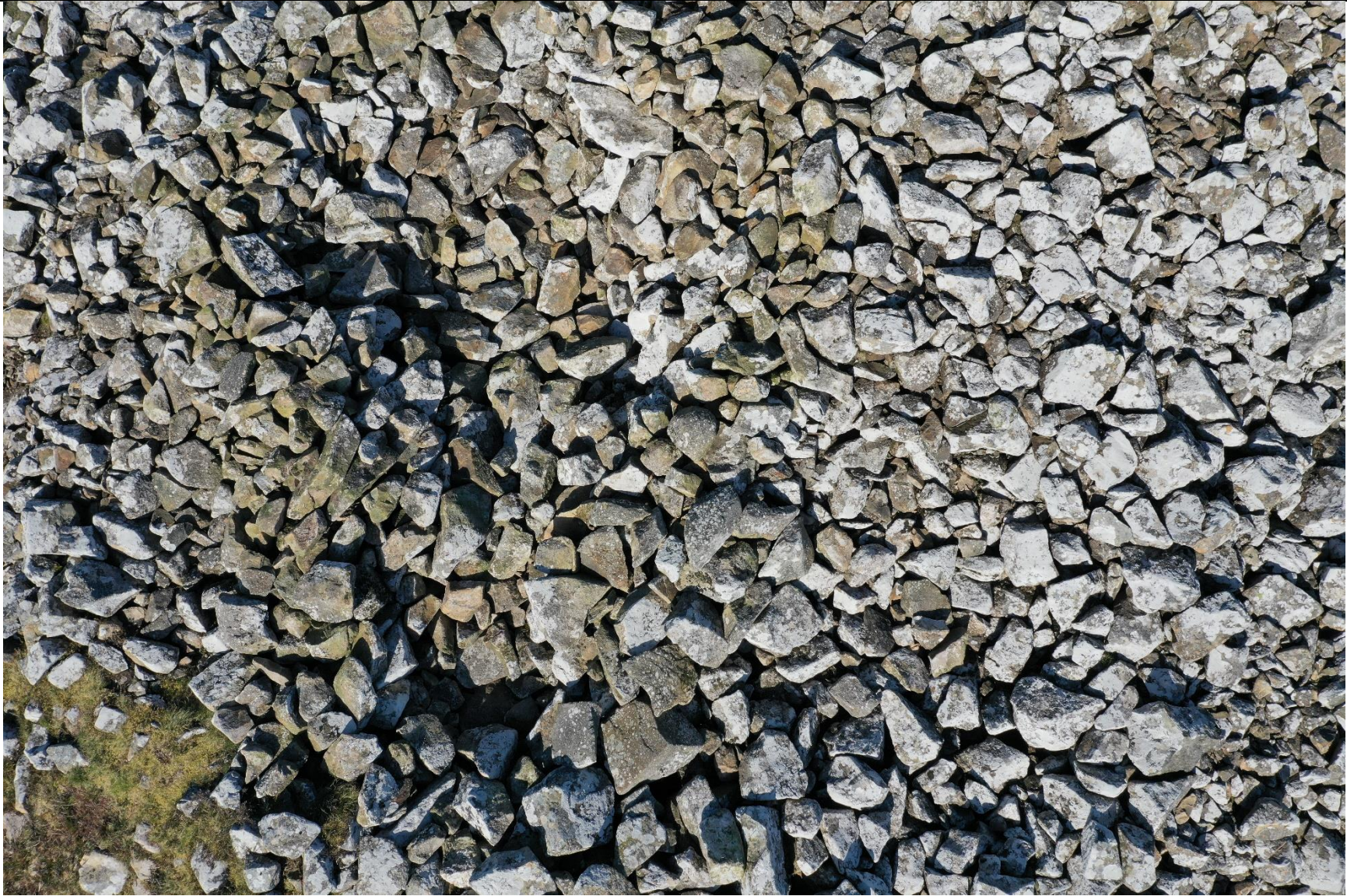
Figure 13. Aerial view of rim and depression after reconsolidation work.
