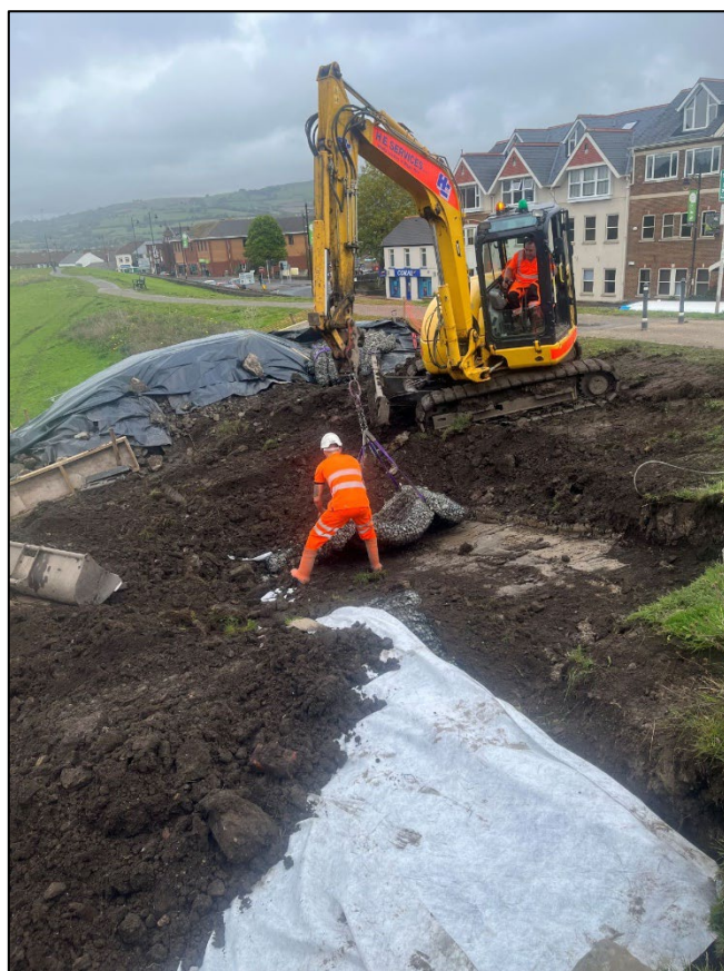
Plate 6: Area 1 E, working shot: laying of pre-filled rock mattress. View to northeast.
