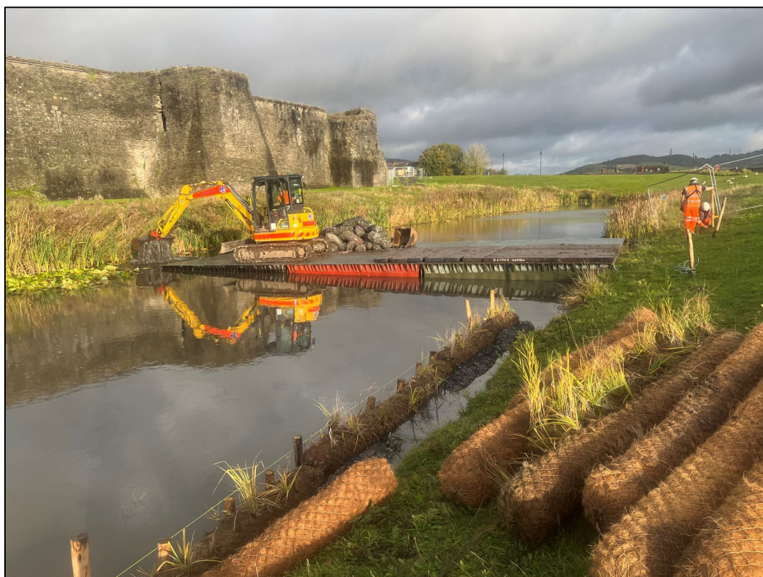
Plate 7: Area 2, laying of coir rolls. View to north.
