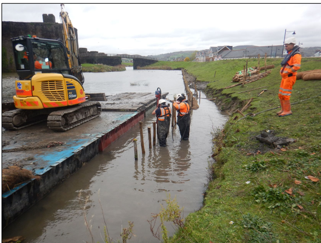
Plate 9: Area 3, south end. Driving stakes ready to receive coir rolls. View to northeast.
