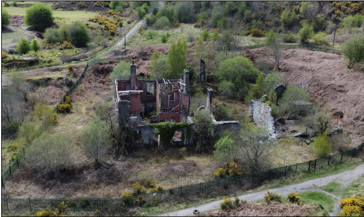
Plate 5. Aerial photograph of British Ironworks Office and Foundry Quadrangle (ID54) (view south)
