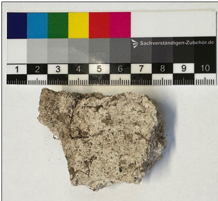
Plate 30. Location 13 NW Service Room, soft white render (*03) applied to the interior of chimney flue [1305] with small black stone aggregate flecks and straw bonding. Lack of smoke blackening suggest only in-situ for short period of time before blocking occurred, 16 th - 17 th century.
