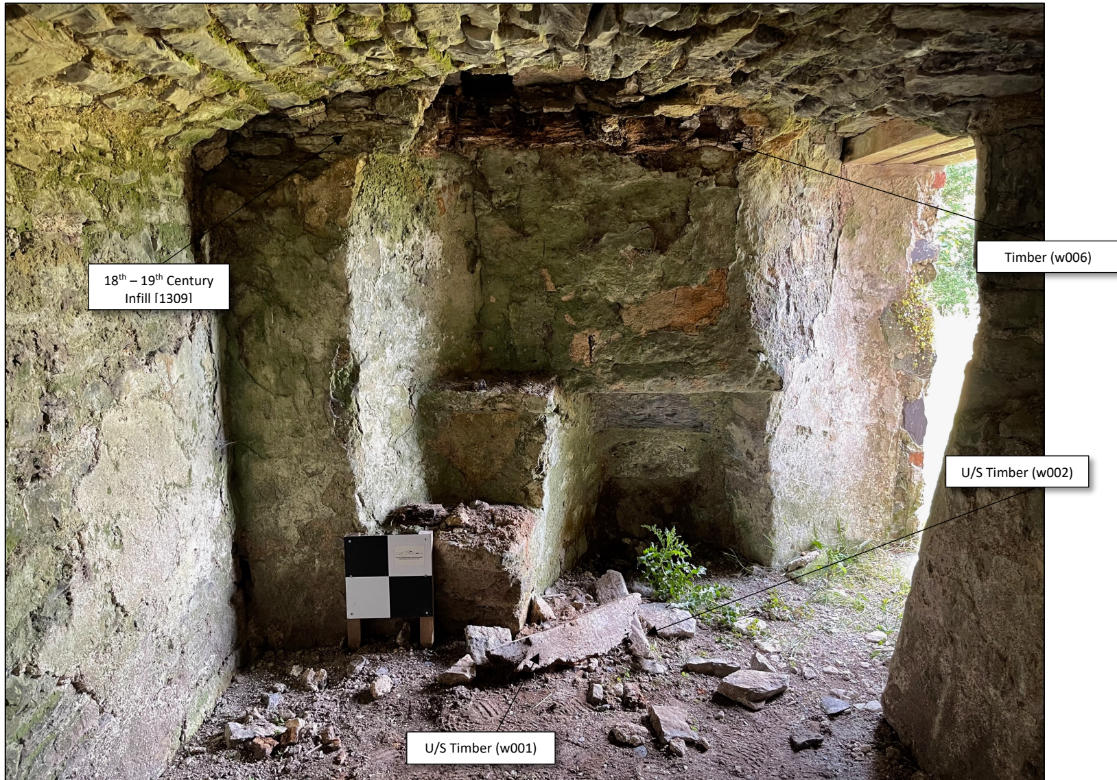
Plate 1. Location 13 NW Service Room, view to SW of hearth/fireplace, Timber (w006) and U/S Timbers (w001) and (w002) recovered from the floor.
