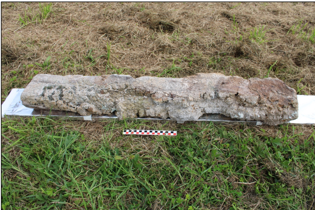
Plate 19. Location 15 Medieval Tower/19 th Century Kitchen, reused sawn timber (w004) recovered from within the masonry internal NE facing wall of the former medieval tower [1501].
