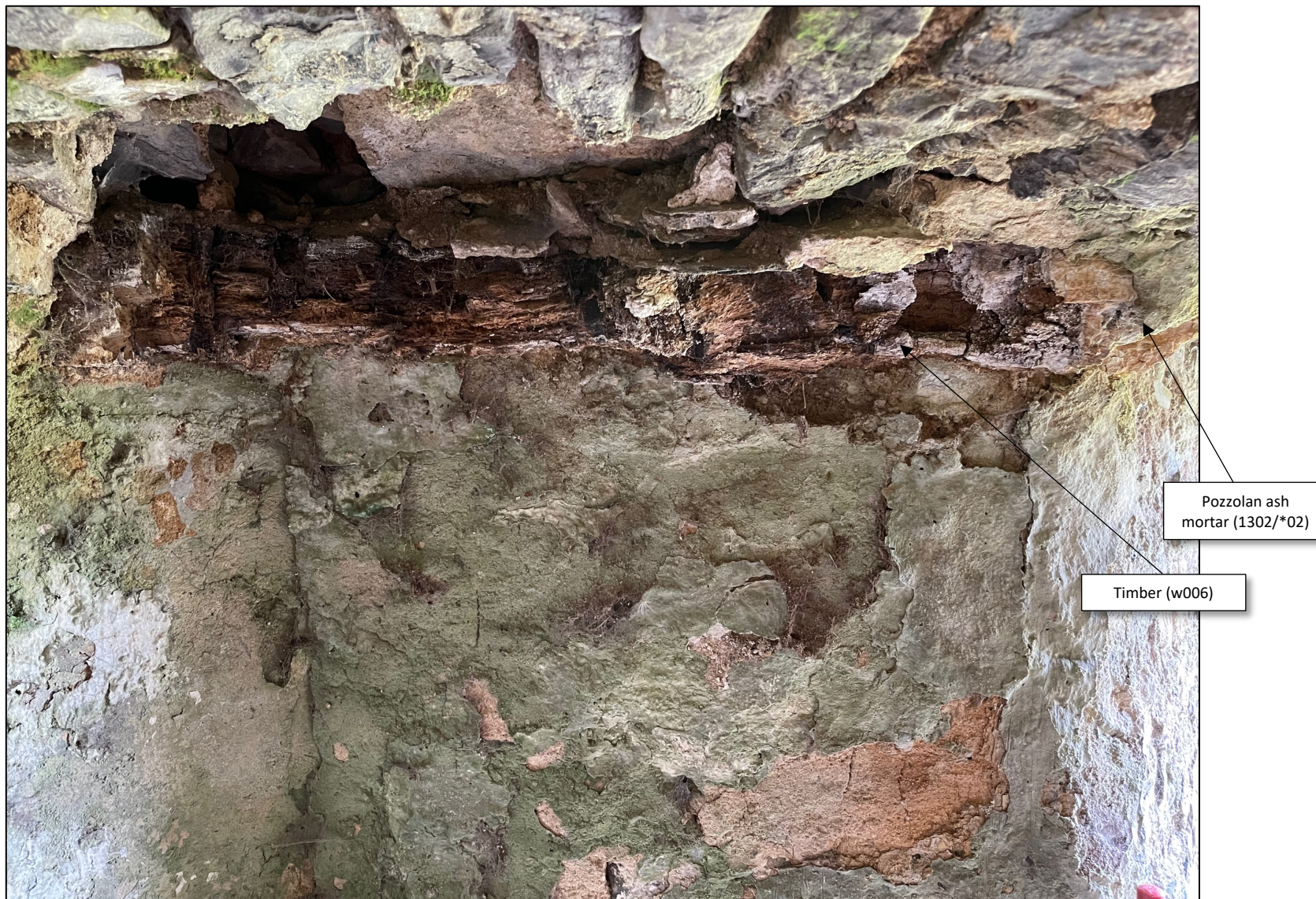
Plate 2. Location 13 NW Service Room, view to SW of Timber (w006).
