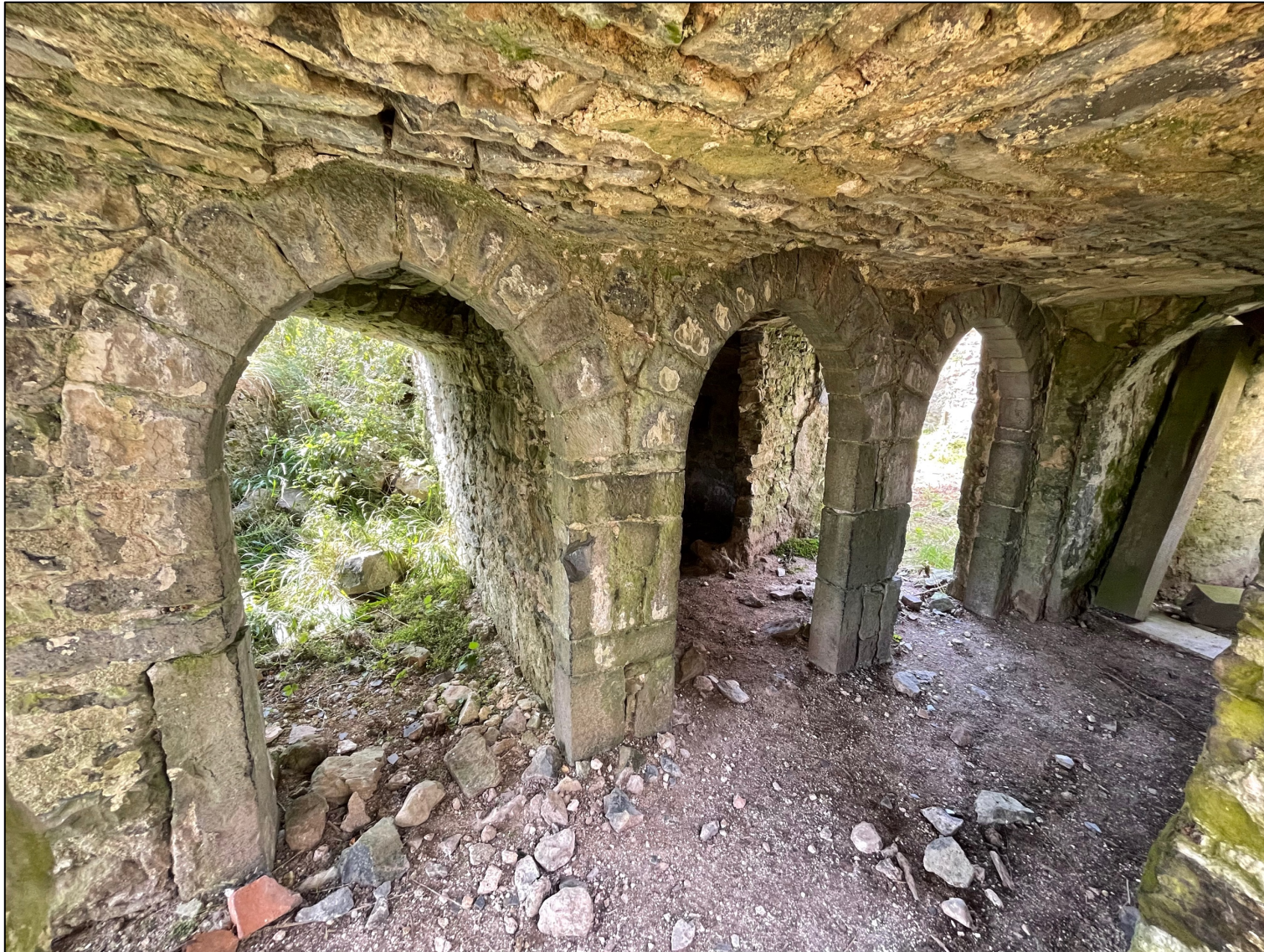
Plate 3. Location 13, view to W of medieval cross passage. Three two-centred stone arched doors leading to vaulted service rooms and Solar room above.
