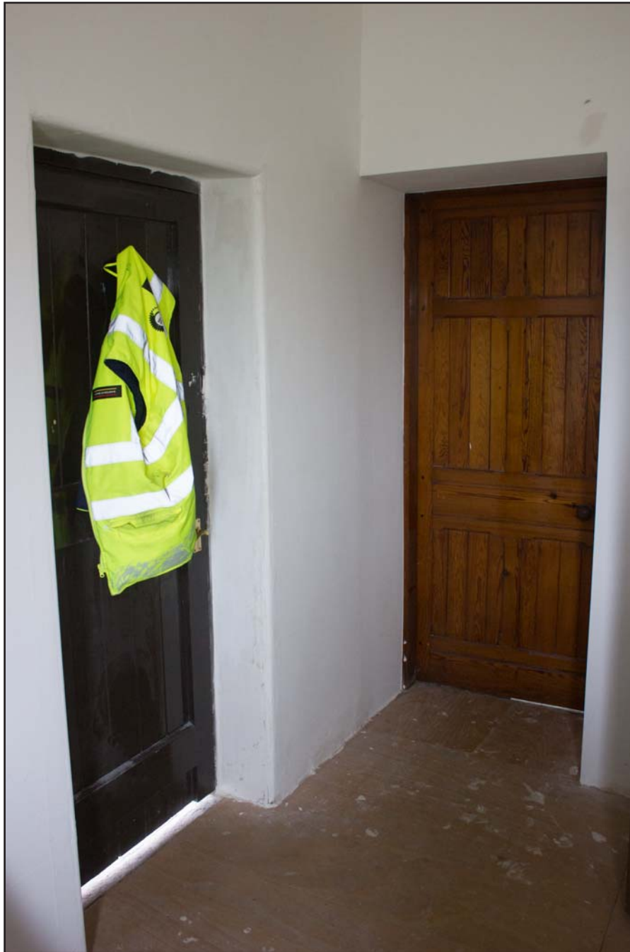
Plate 55: Vestry, Gwynfa Chapel, Pen-y-ffordd, Holywell, Flintshire - from the northwest - no scale
