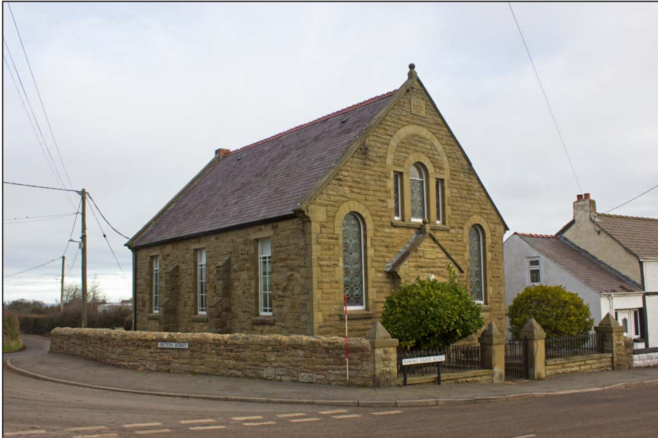
Plate 03: External oblique south & west elevations of Gwynfa Chapel, Pen-y-ffordd, Holywell, Flintshire - from the southwest - 2.00m scale
