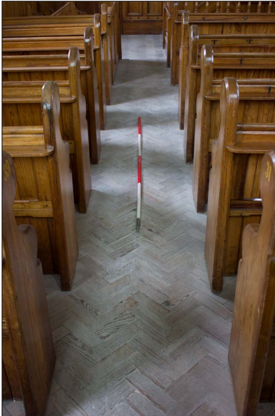
Plate 50: Parquet floor of eastern aisle within Gwynfa Chapel, Pen-y-ffordd, Holywell, Flintshire - from the south - 2.00m scale
