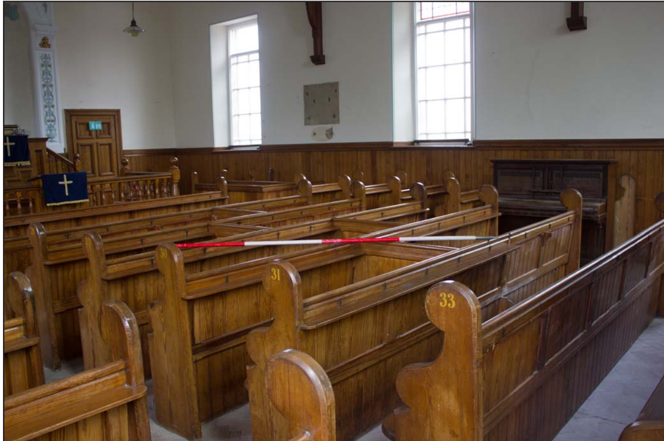
Plate 36: Oblique shot of rear pews Gwynfa Chapel, Pen-y-ffordd, Holywell, Flintshire - from the southwest - no scale
