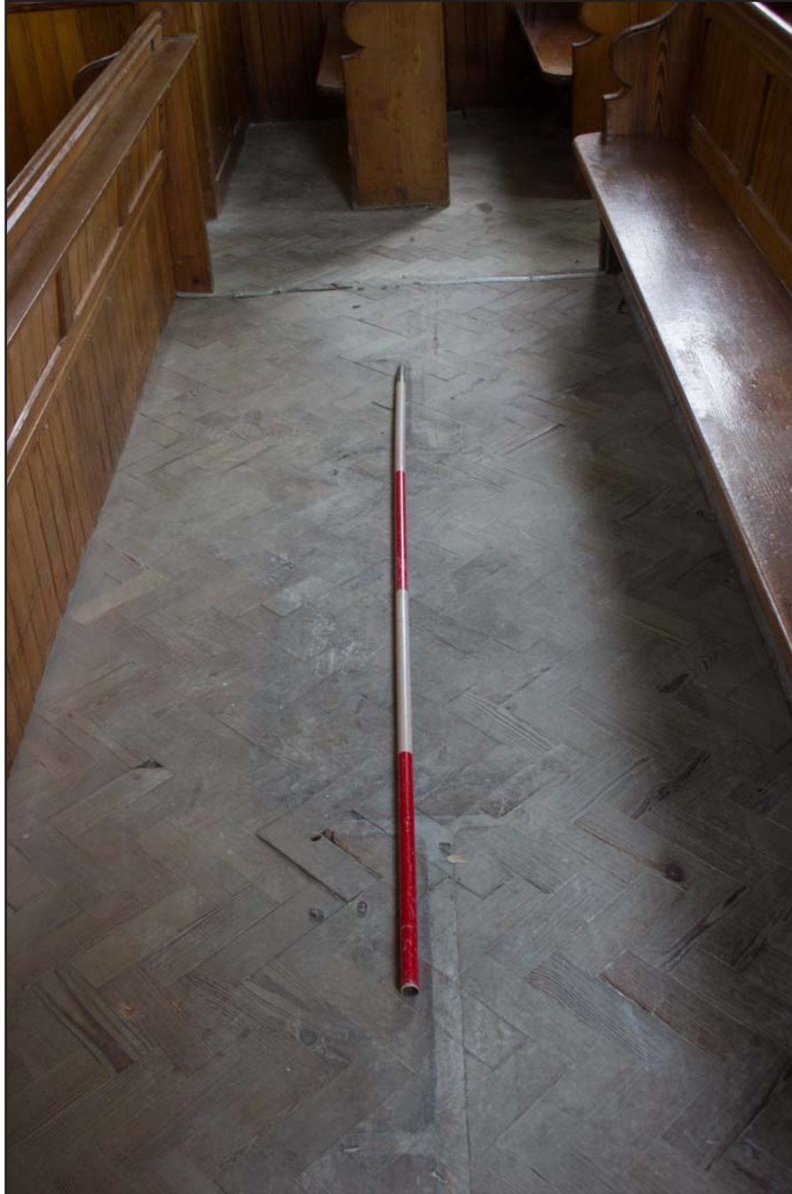
Plate 51: Parquet floor in centre of Gwynfa Chapel, Pen-y-ffordd, Holywell, Flintshire - from the west - 2.00m scale
