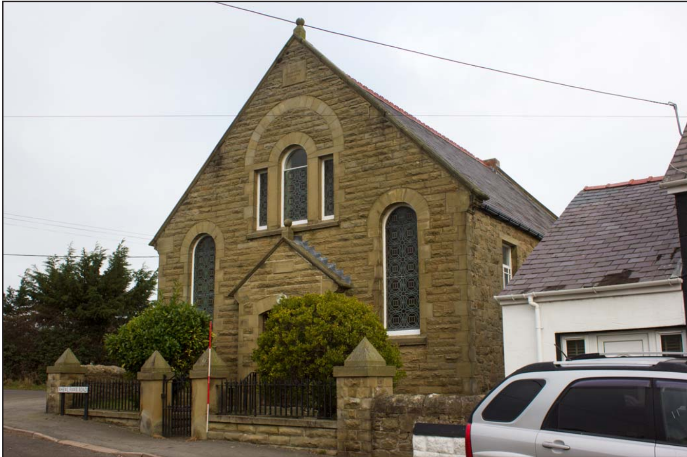
Plate 01: External oblique south & east elevations of Gwynfa Chapel, Pen-y-ffordd, Holywell, Flintshire - from the southeast - 2.00m scale
