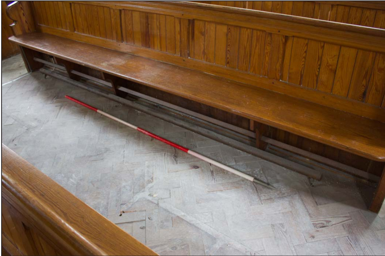
Plate 52: Under pew heater, Gwynfa Chapel, Pen-y-ffordd, Holywell, Flintshire - from the northwest - 2.00m scale
