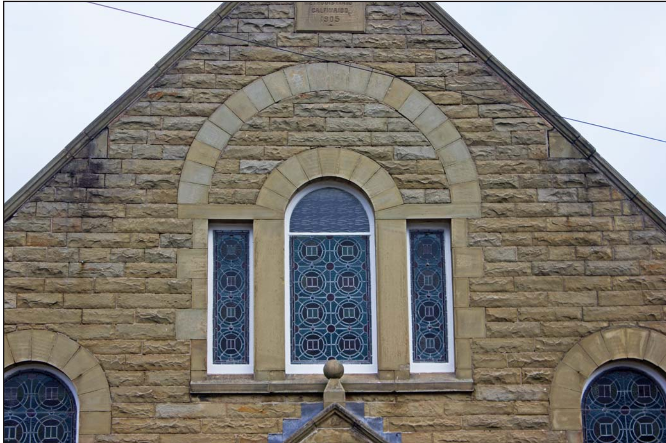
Plate 14: First storey window, southern elevation, Gwynfa Chapel, Pen-y-ffordd, Holywell, Flintshire - from the south - no scale
