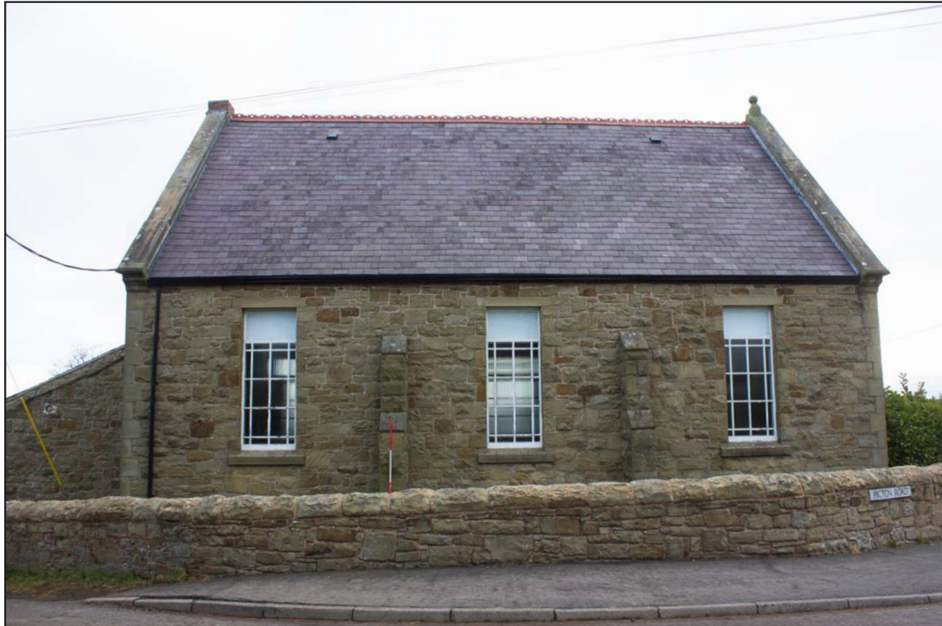
Plate 04: External western elevation of Gwynfa Chapel, Pen-y-ffordd, Holywell, Flintshire - from the west - 2.00m scale
