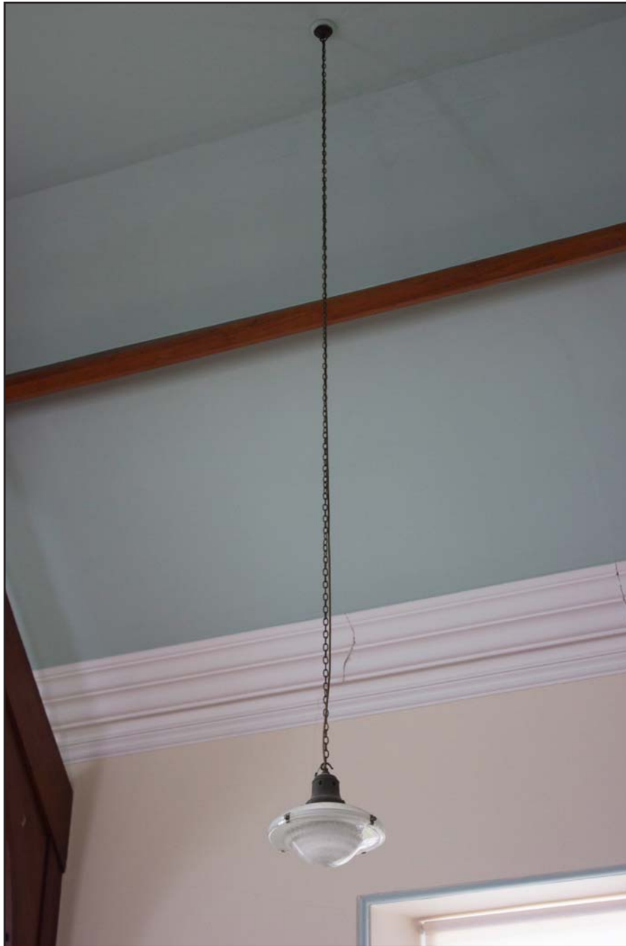
Plate 46: Light fitting hanging from the ceiling of Gwynfa Chapel, Pen-y-ffordd, Holywell, Flintshire - from the east - no scale
