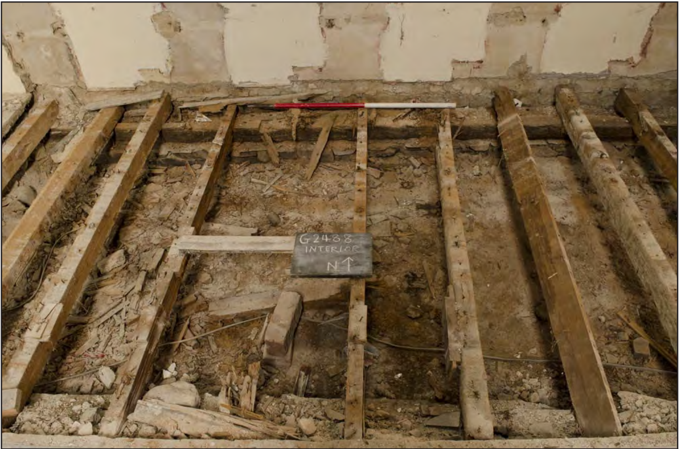
Plate 09: Exposed floor joists along northern wall adjacent to entrance; scale: 1x1m (archive reference: G2488_087).
