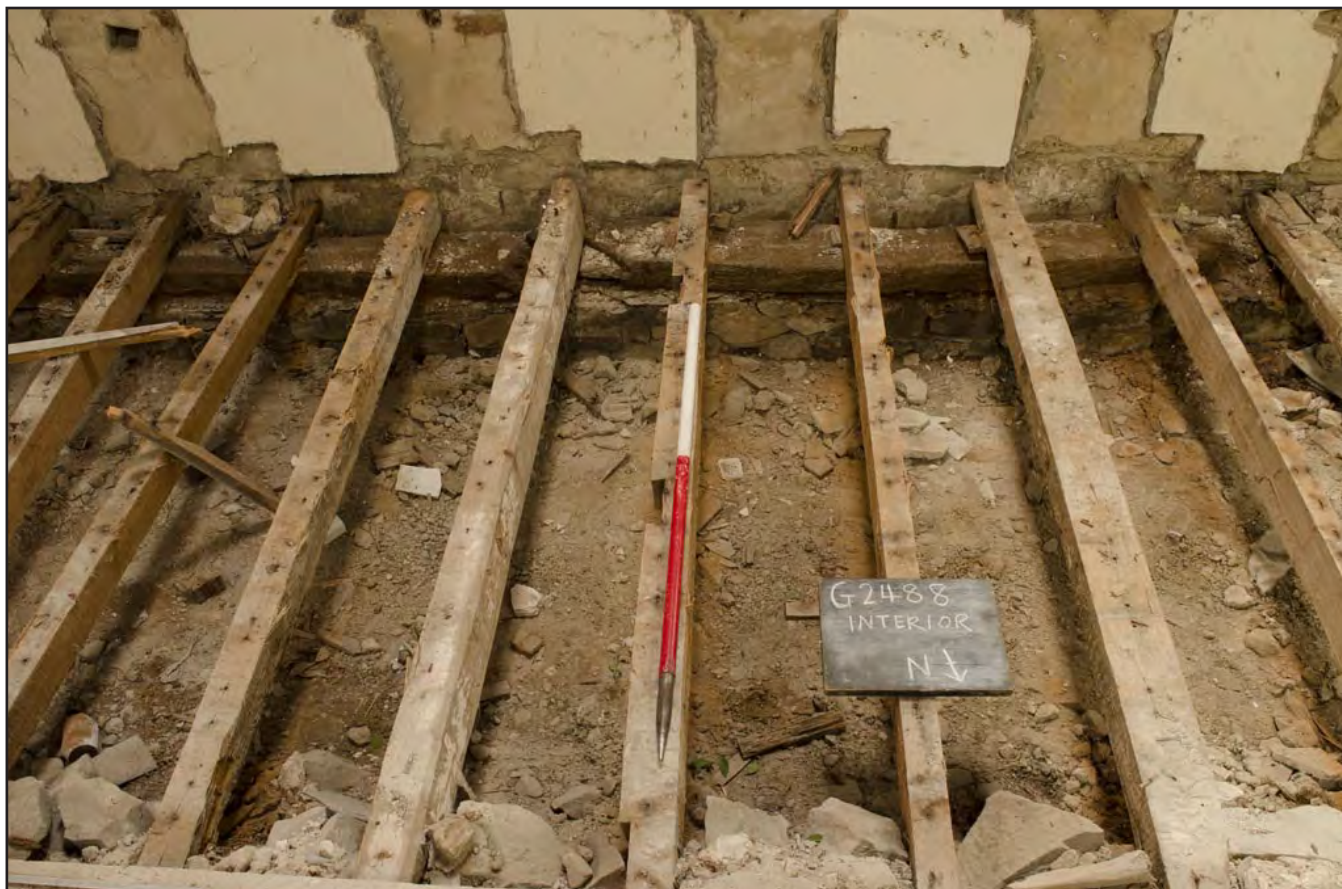
Plate 05: Exposed floor joists at southern end of the church; scale: 1x1m (archive reference: G2488_080).
