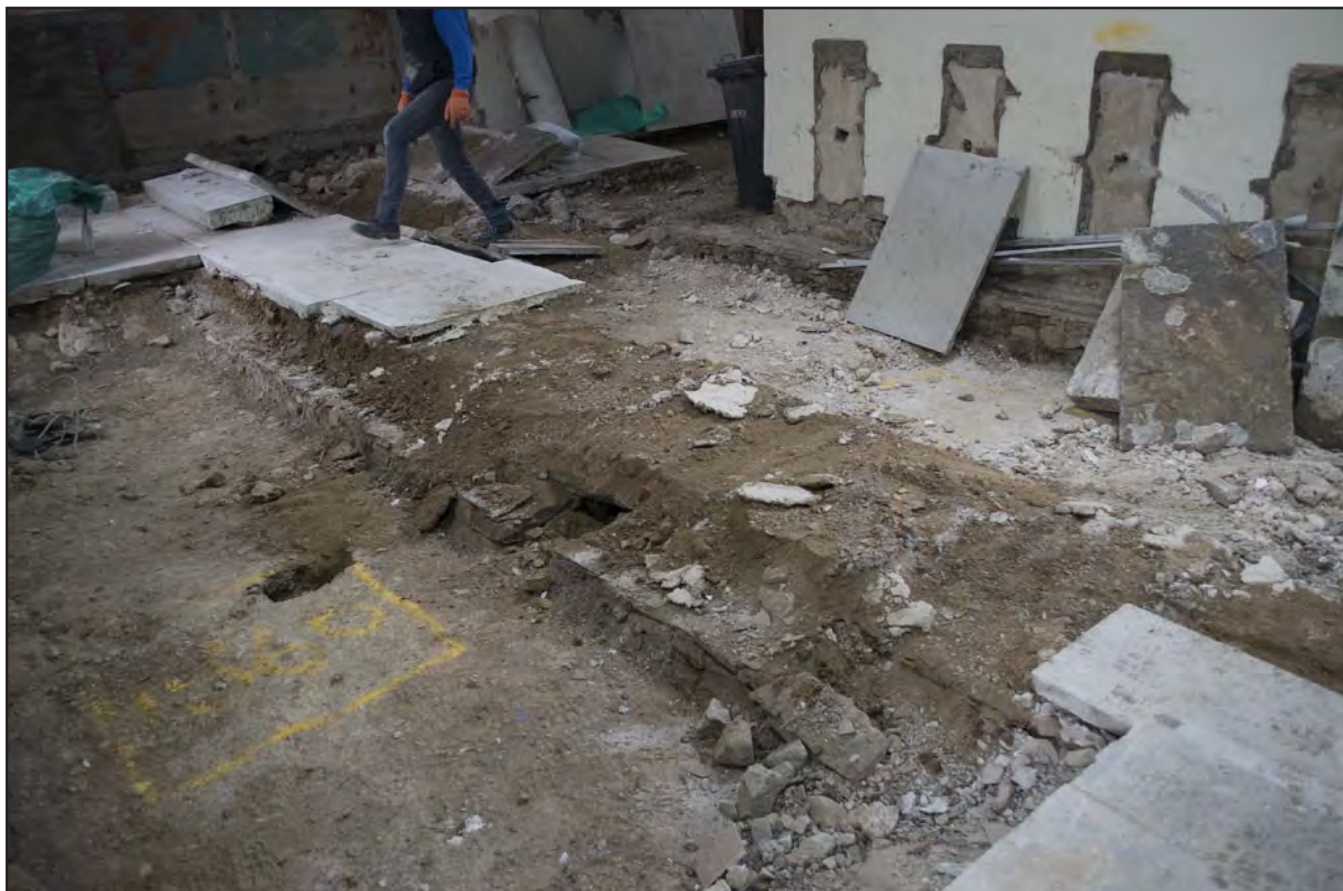
Plate 31: Removal of stone floor slabs; scale not used (archive reference: G2488_146).
