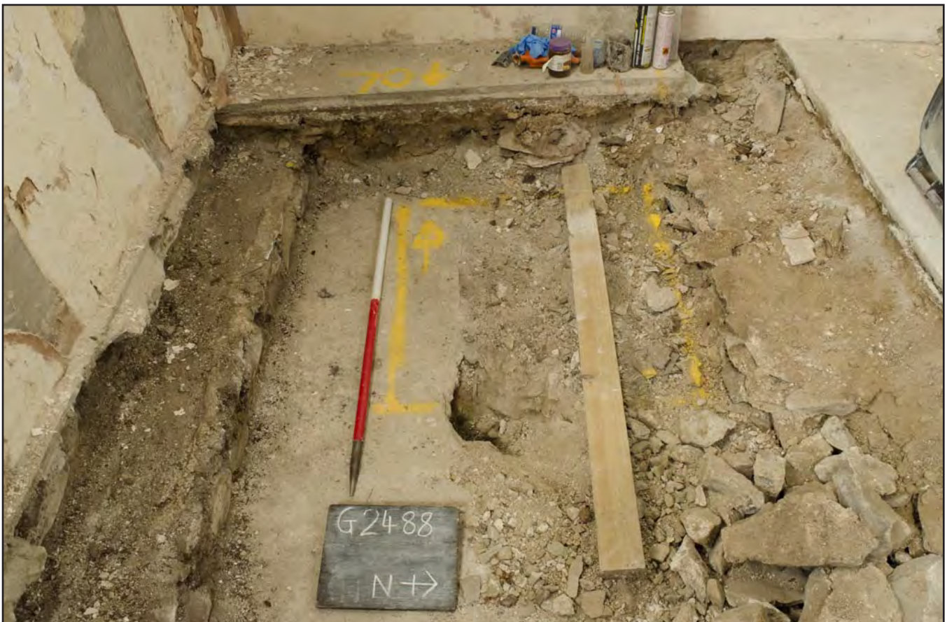
Plate 24: Southwest mezzanine base location and concrete floor exposed; scale: 1x1m (archive reference: G2488_121).
