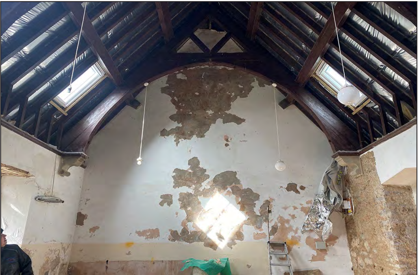
Plate 34: Western church wall after flaked plaster removed; scale not used (archive reference: client photo).
