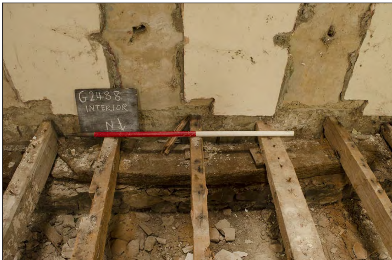
Plate 07: Joists resting on wooden plank and joist hangers along southern wall of church; scale: 1x1m (archive reference: G2488_081).
