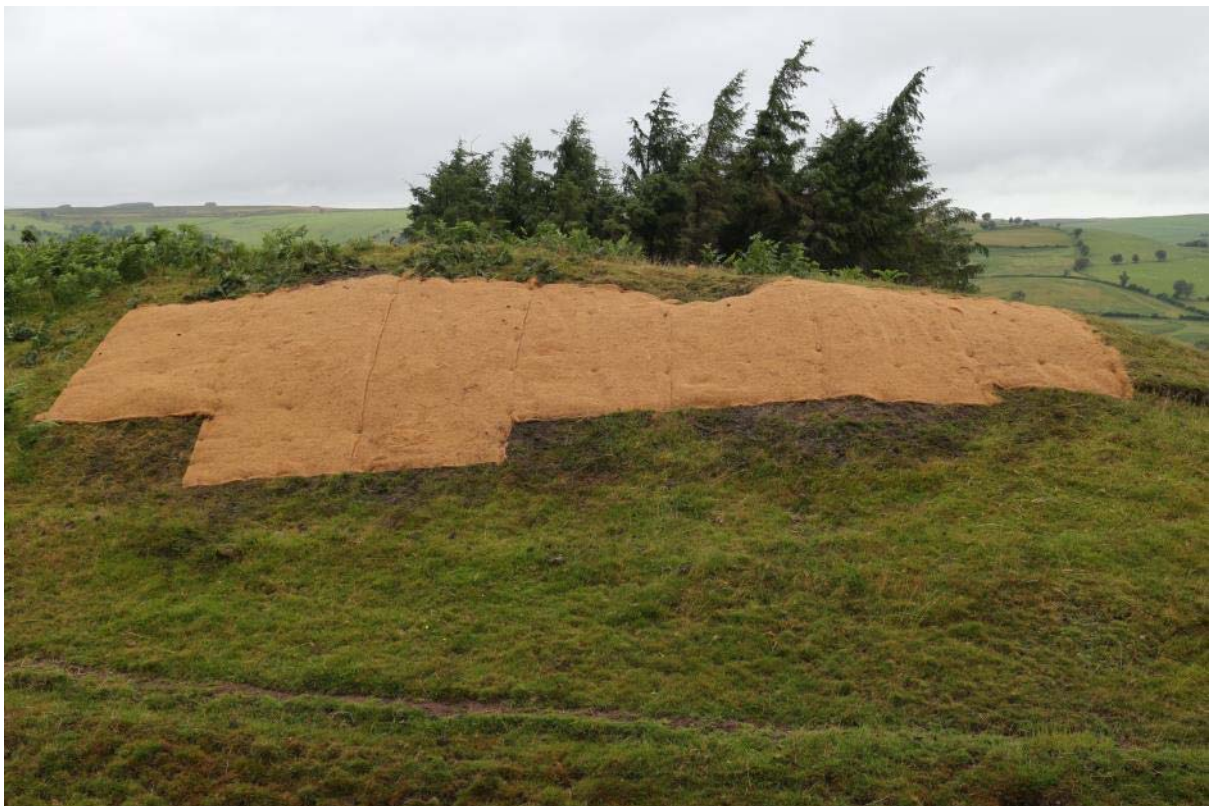
Locations 1 & 2, completed repair, IMG_7485, 20.07.2015
