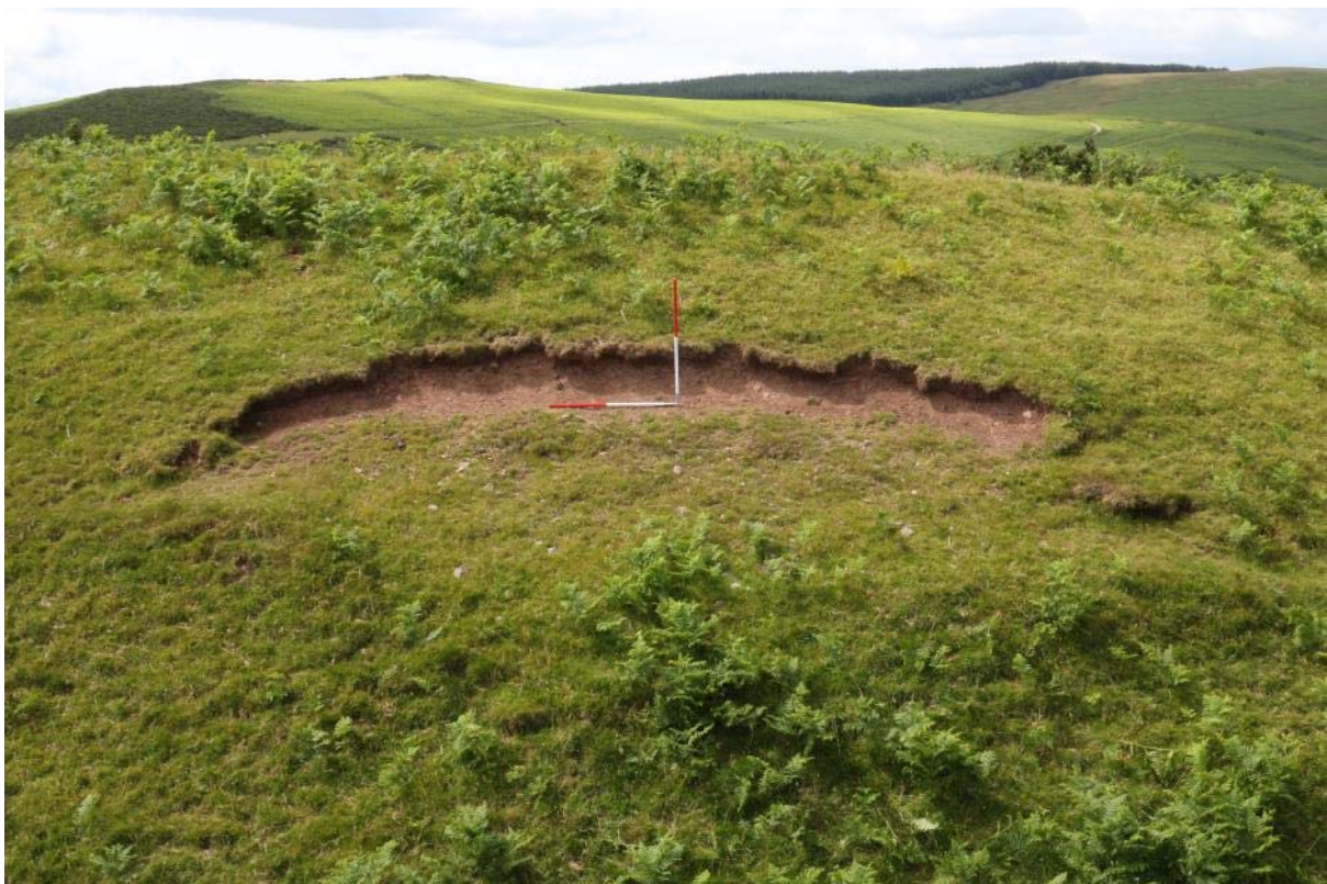
Location 9, before repair, IMG_7458, 18.07.2015
