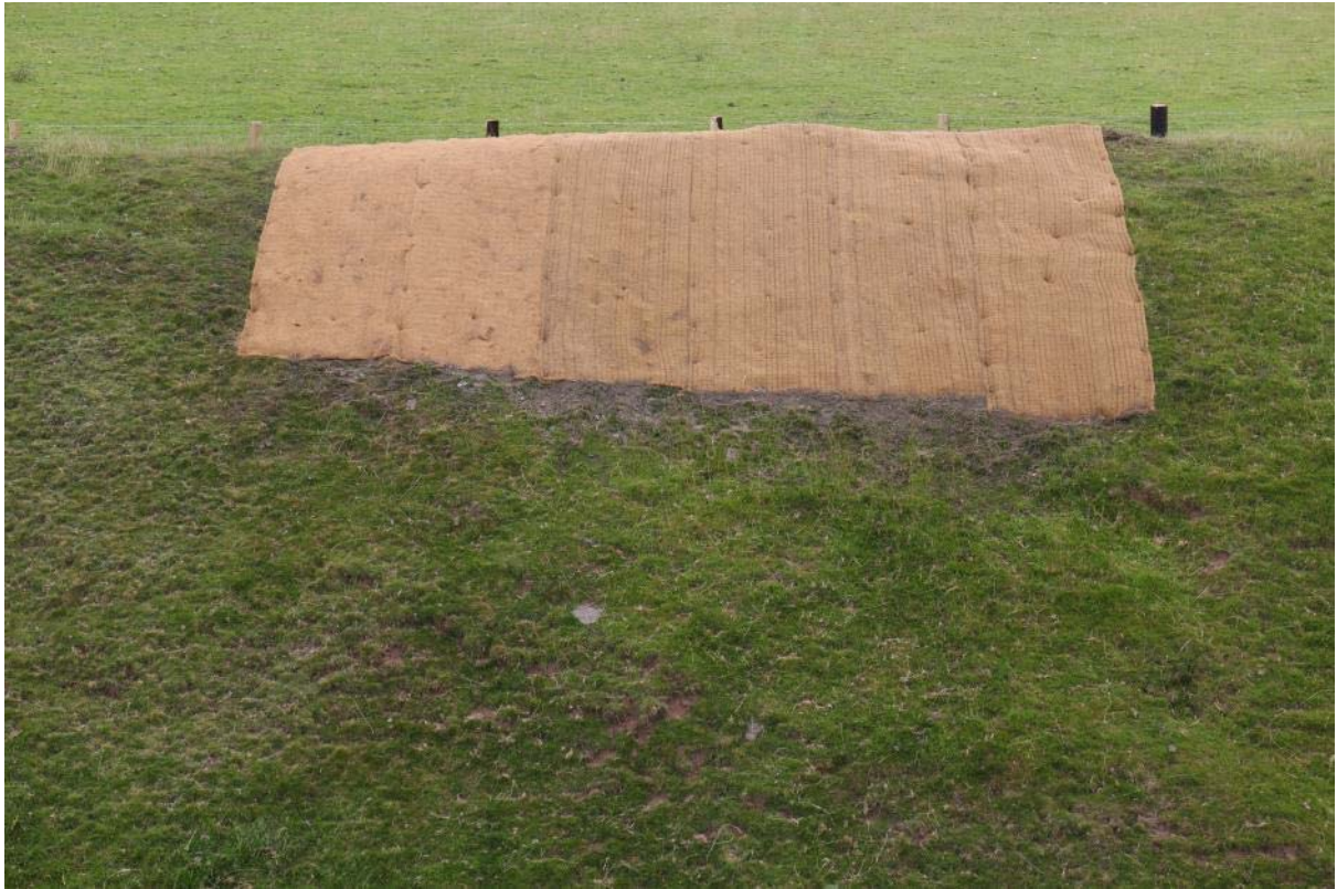
Location 10, completed repair, IMG_7635, 23.07.2015
