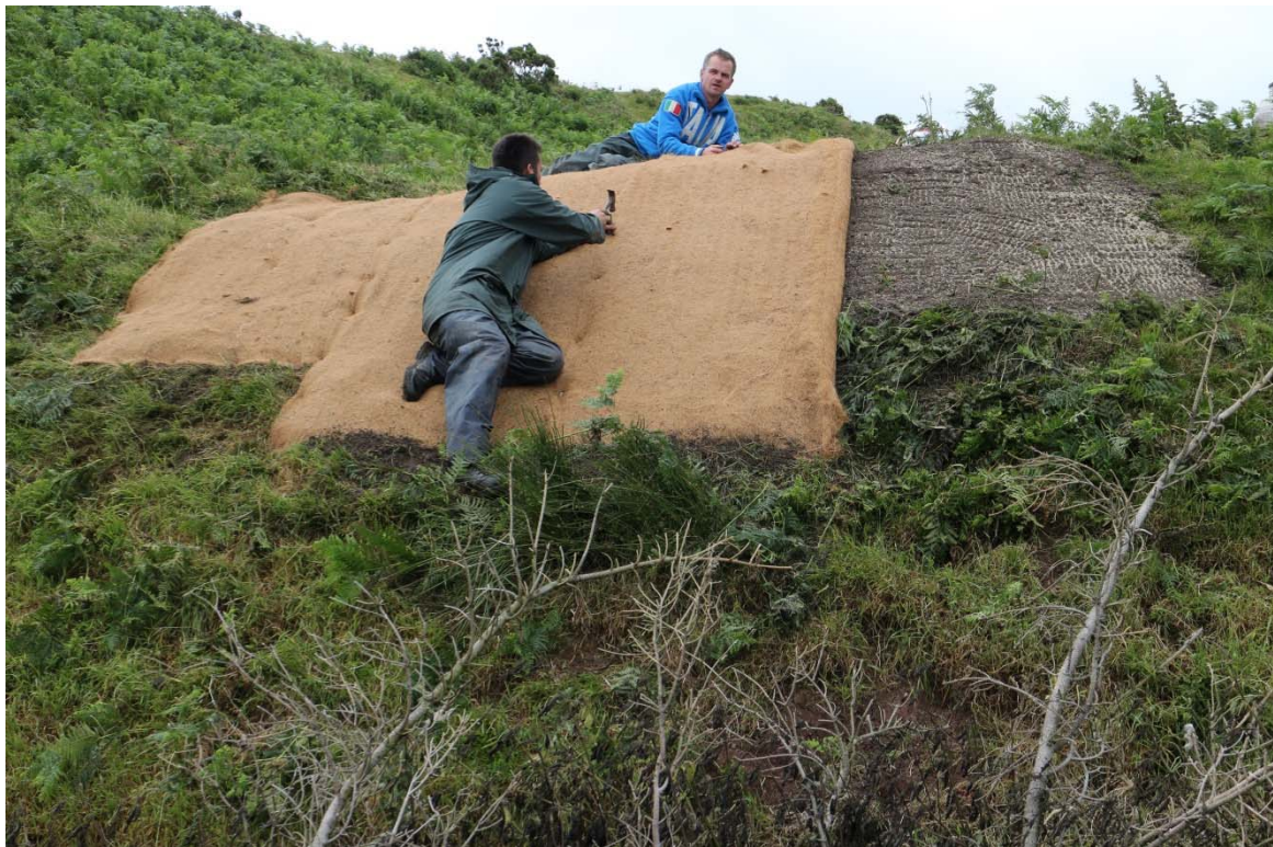
Location 7, infilled, reprofiled, installing Greenfix Eromat Type 6S, IMG_7486, 20.07.2015
