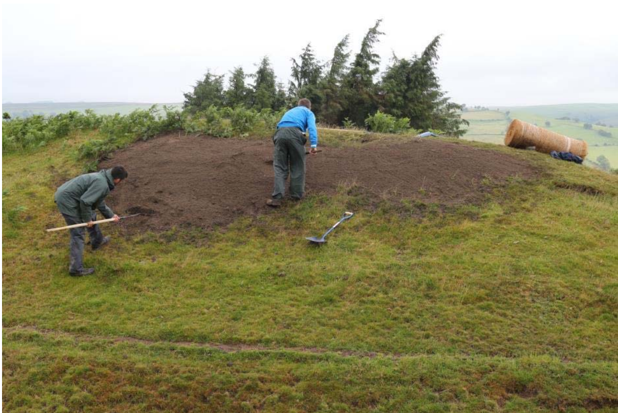
Locations 1 & 2, infilling and reprofiling, IMG_7471, 20.07.2015
