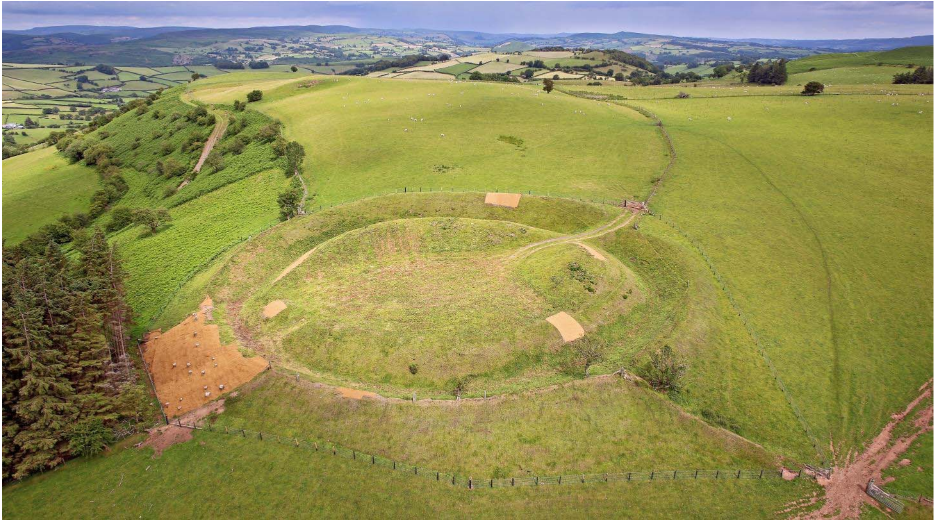
Completed conservation works, looking east, ©Richard Stanton Photographic, 23.07.2015
