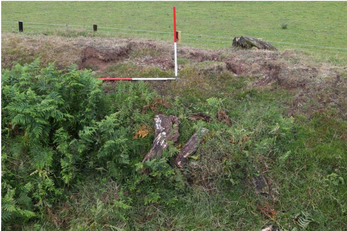
Location 12, before repair, IMG_7524, 21.07.2015
