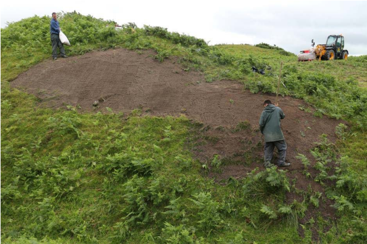
Location 8, infilling and reprofiling, IMG_7489, 20.07.2015
