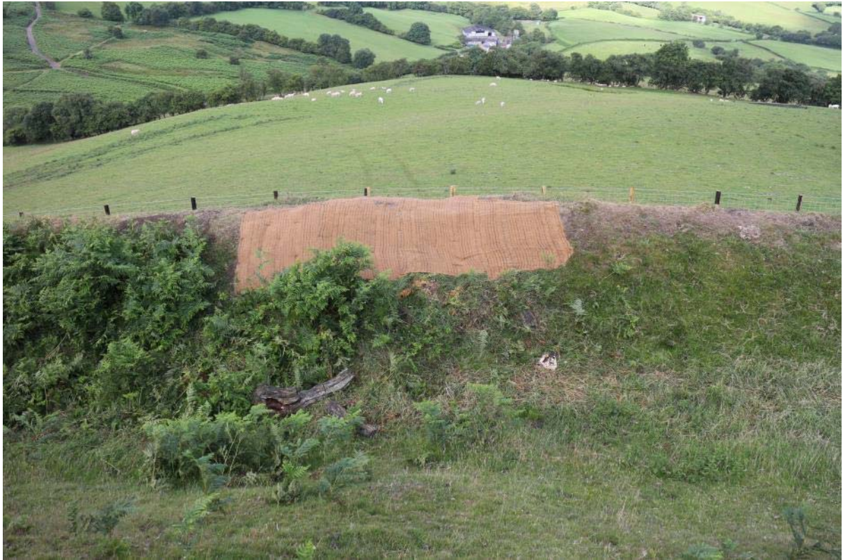
Location 12, completed repair, IMG_7530, 21.07.2015
