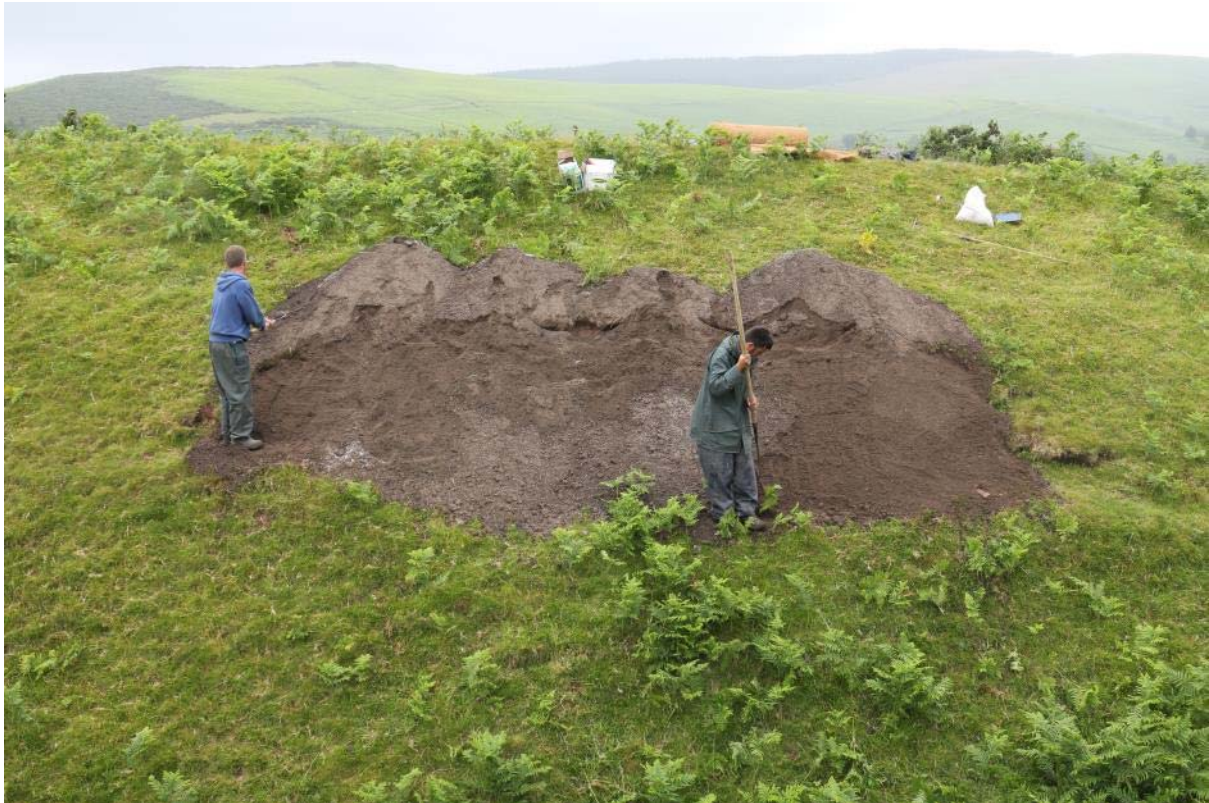
Location 9, infilling and reprofiling, IMG_7507, 20.07.2015
