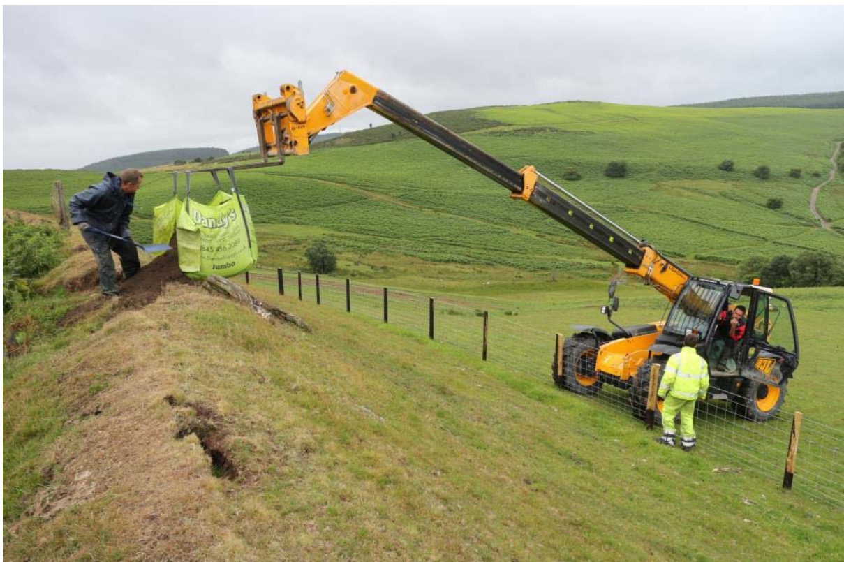
Location 12, commencing infilling and reprofiling, IMG_7529, 21.07.2015
