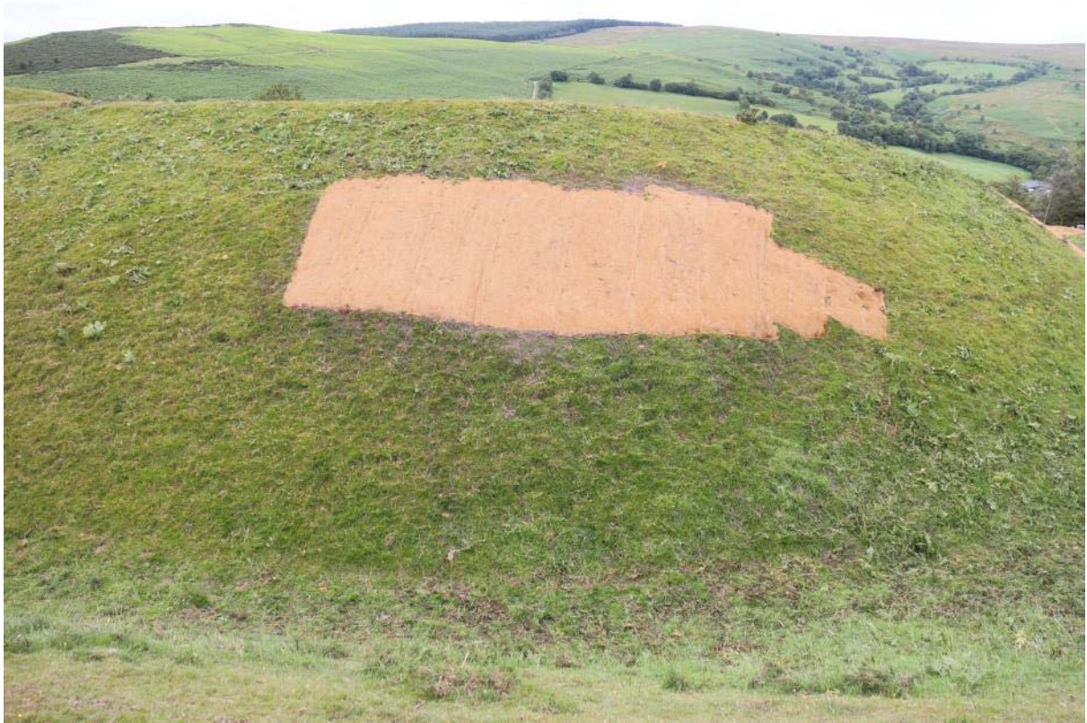
Location 9, completed repair, after bracken strimming/crushing, IMG_7631, 23.07.2015
