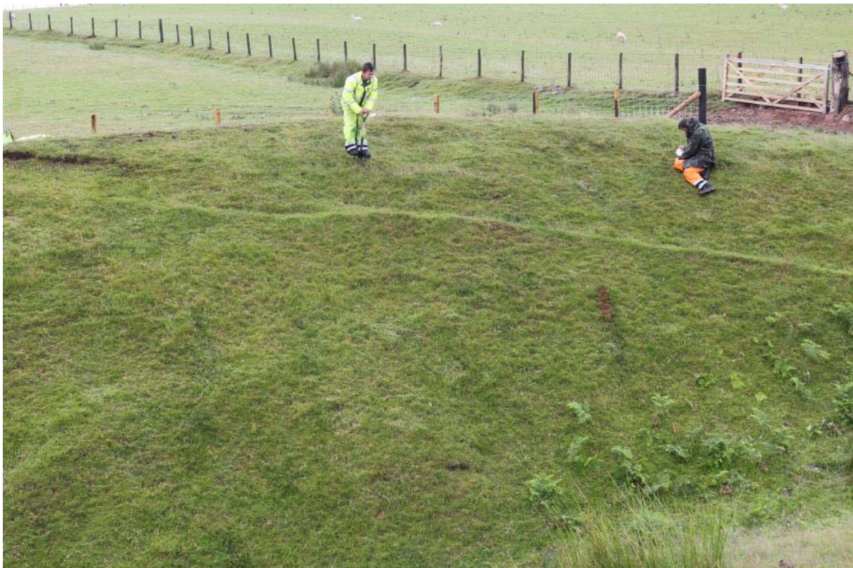
Location 11, during sward enhancement works, IMG_7518, 20.07.2015
