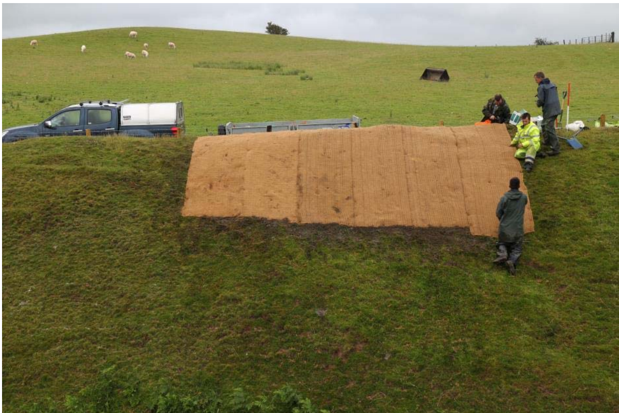
Location 10, installing Greenfix Eromat Type 6S, IMG_7519, 20.07.2015
