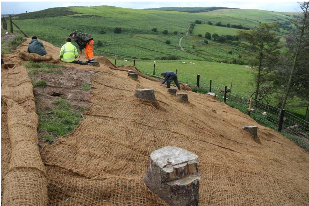
Installing Geocoir 900 matting, IMG_7542, 21.07.2015
