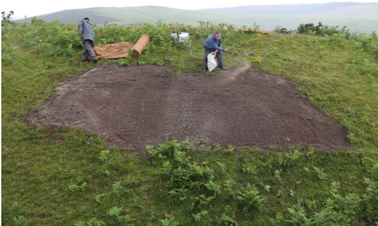
Location 9, hand broadcasting grass seed before installing matting, IMG_7508, 20.07.2015
