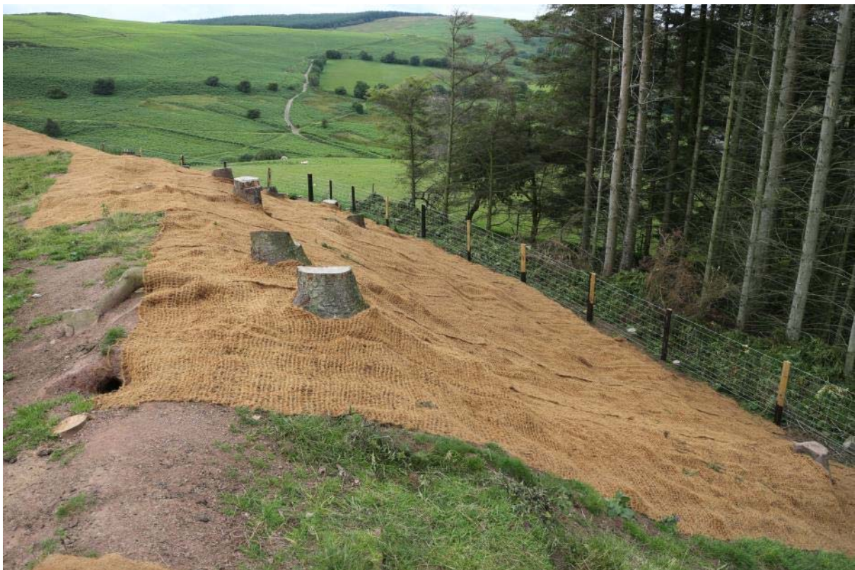
Completed repair, looking west, IMG_7622, 23.07.2015
