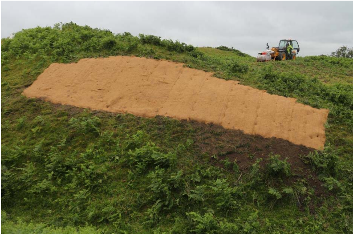
Location 8, completed repair, IMG_7504, 20.07.2015
