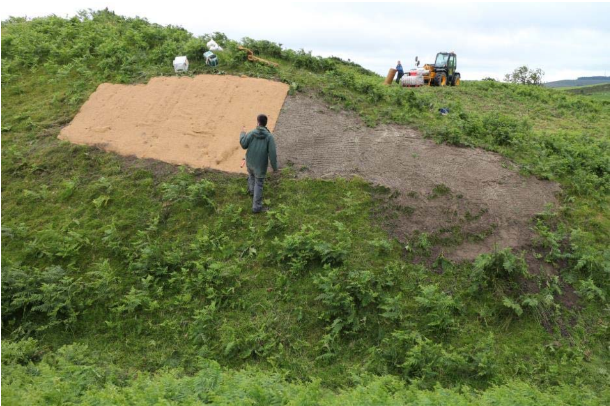
Location 8, installing Greenfix Eromat Type 6S, IMG_7493, 20.07.2015
