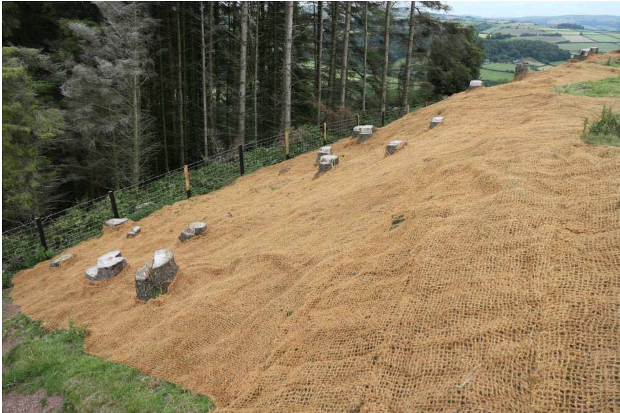
Completed repair, looking east, IMG_7620, 23.07.2015
