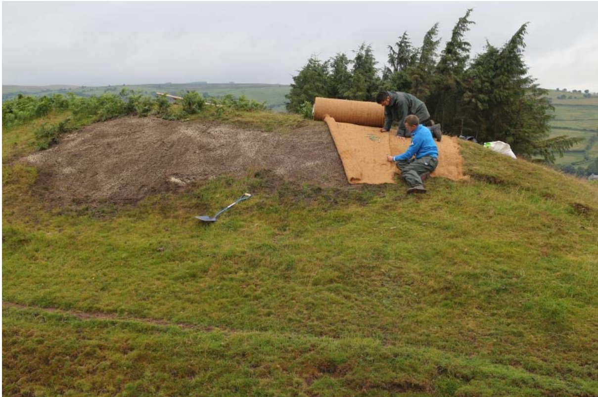
Locations 1 & 2, installing Greenfix Eromat Type 6S, IMG_7478, 20.07.2015
