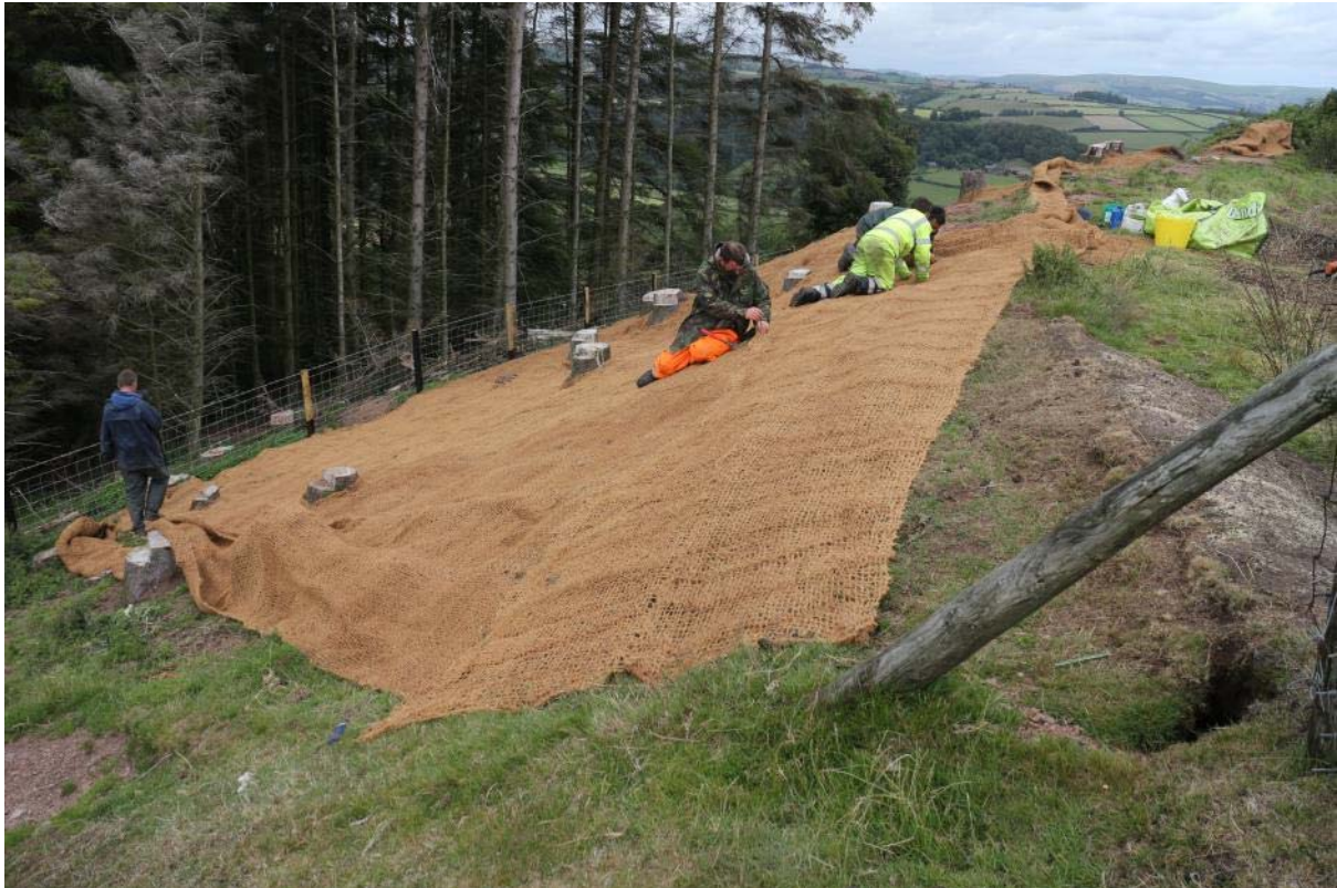
Installing Geocoir 900 matting, IMG_7537, 21.07.2015
