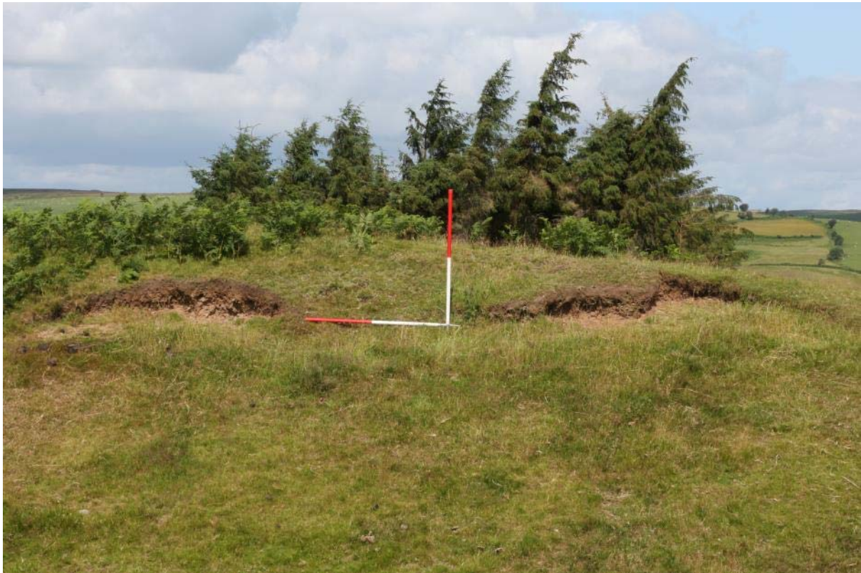
Locations 1 & 2, before repair, IMG_7456, 18.07.2015
