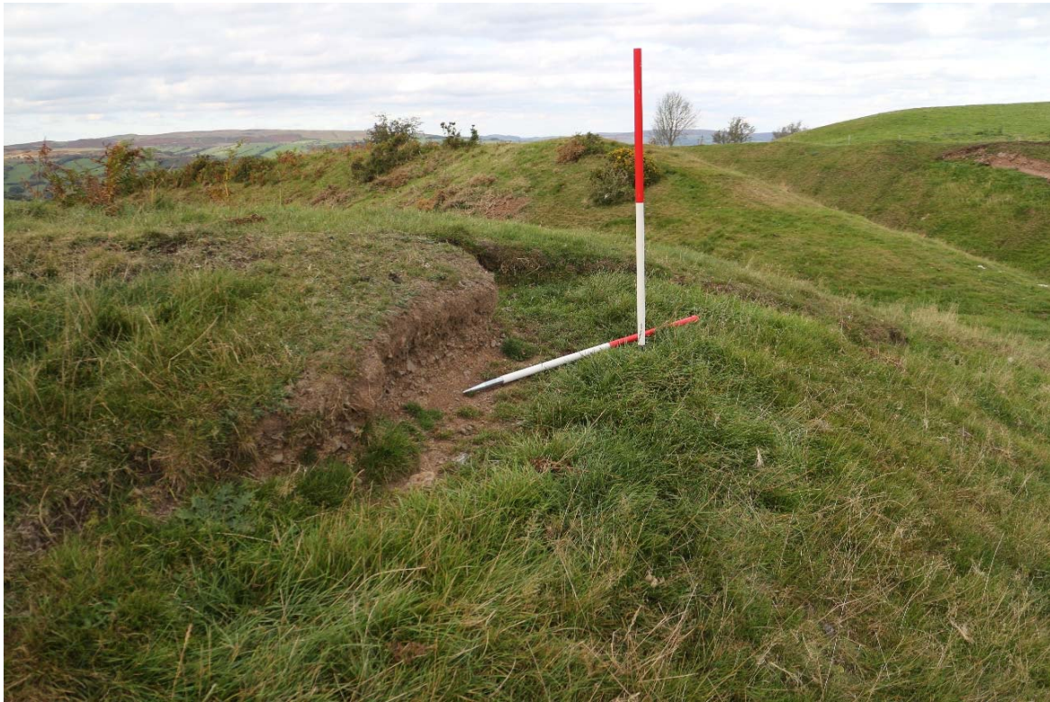
Location 1, before repair, IMG_2483, 02.10.2014
