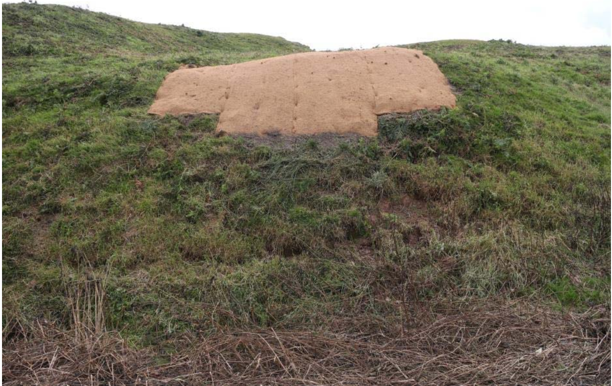
Location 7, completed repair, IMG_7628, 23.07.2015
