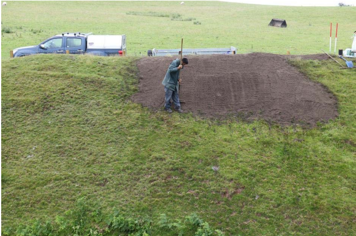
Location 10, infilling and reprofiling, IMG_7515 20.07.2015
