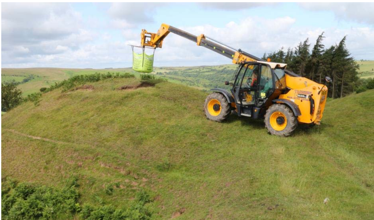
Delivery of topsoil to accessible erosion scars by JCB 535-95 Loadall, IMG_7450, 18.07.2015
