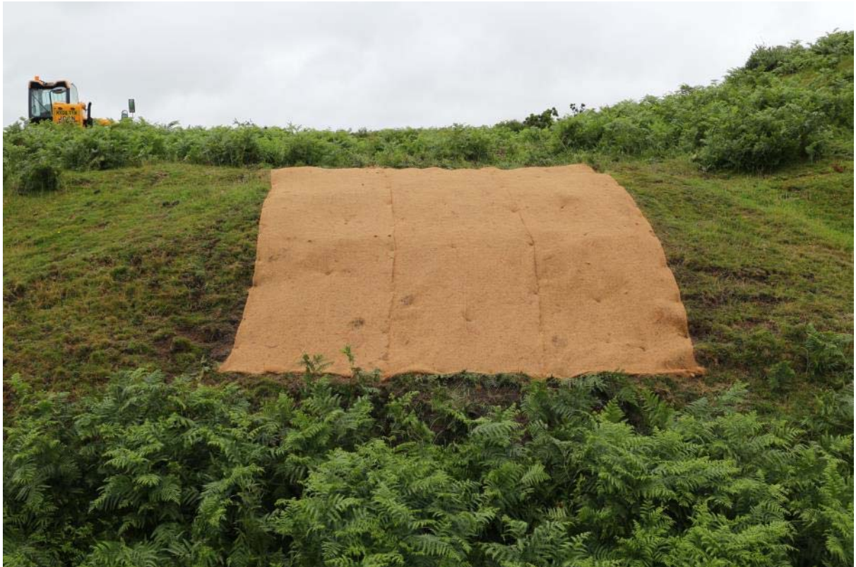
Locations 4, 5 & 6, completed repair, 20.07.2015
