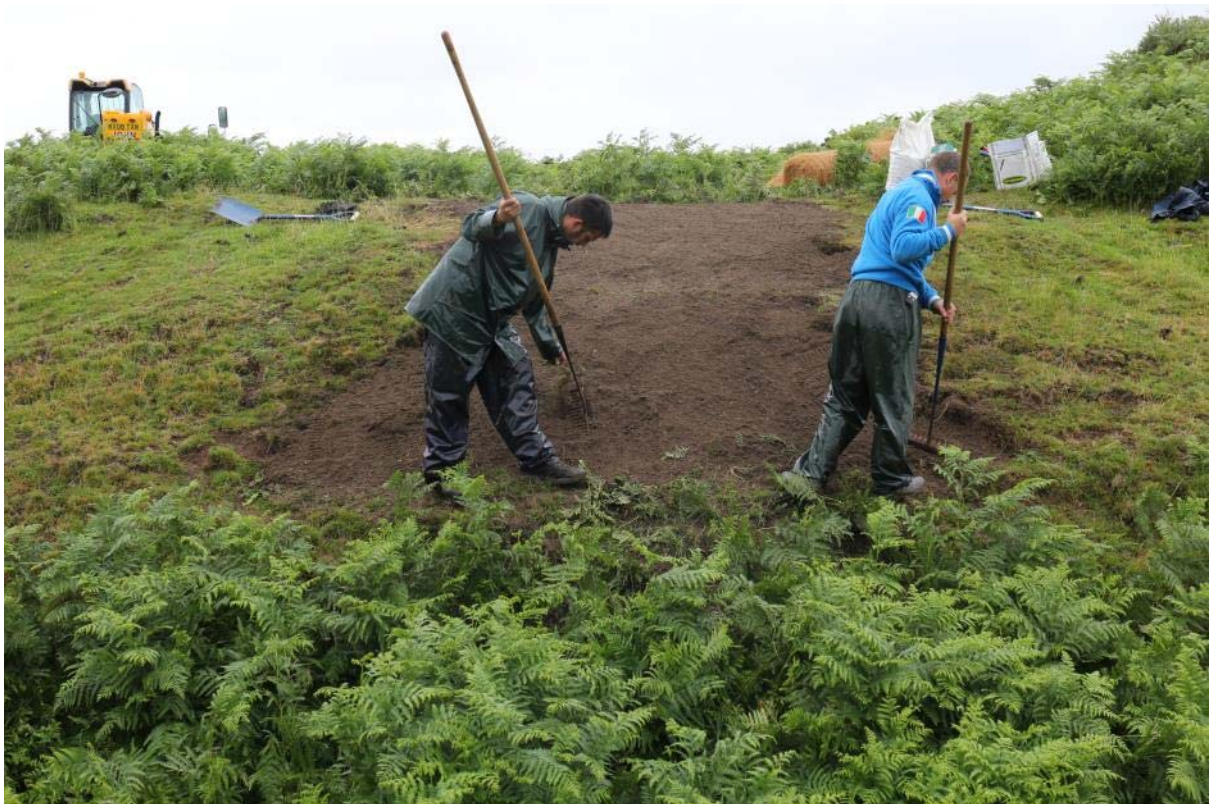
Locations 4,5 & 6, infilling and reprofiling, IMG_7483, 20.07.2015
