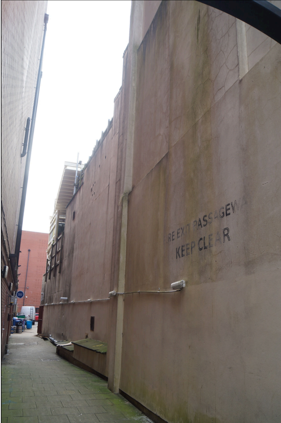
Plate 3: A view along the alleyway to the east of the former National Westminster Bank, showing the eastern side of the listed building. The structure of the mezzanine floor and canopy is visible at the far end of the building. Looking south-southwest.
