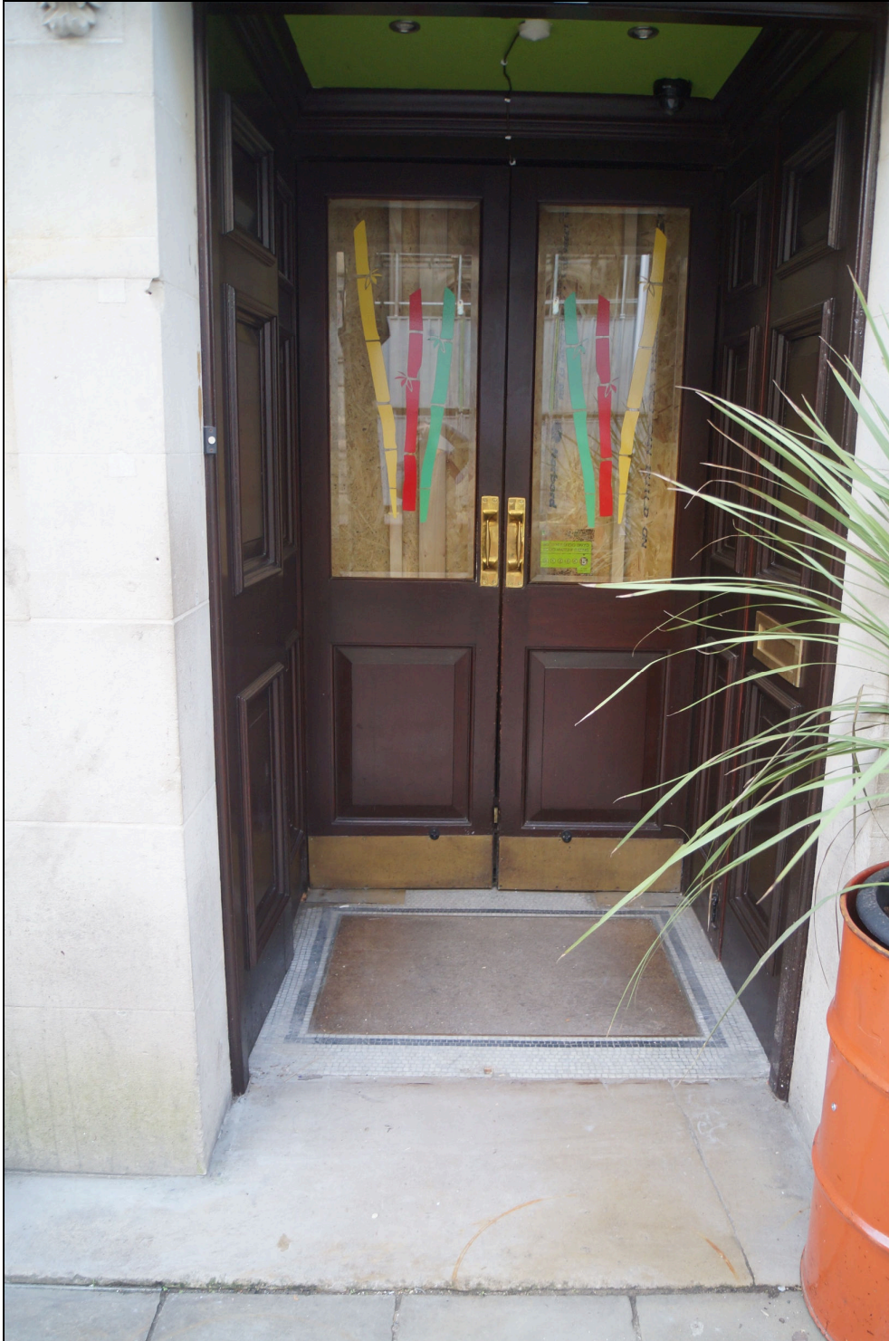
Plate 24: A view of the western doorway through the façade, the entrance to number 52, Wind Street originally, showing it fully open and revealing the entrance porch and inner doors. These doors and door furniture are also original, as are the mosaic tiled floor. Note how the outer doors either side have opened into a recess in order to ensure they do not impede access in any way. They are not affected by the development. Looking south-southwest.
