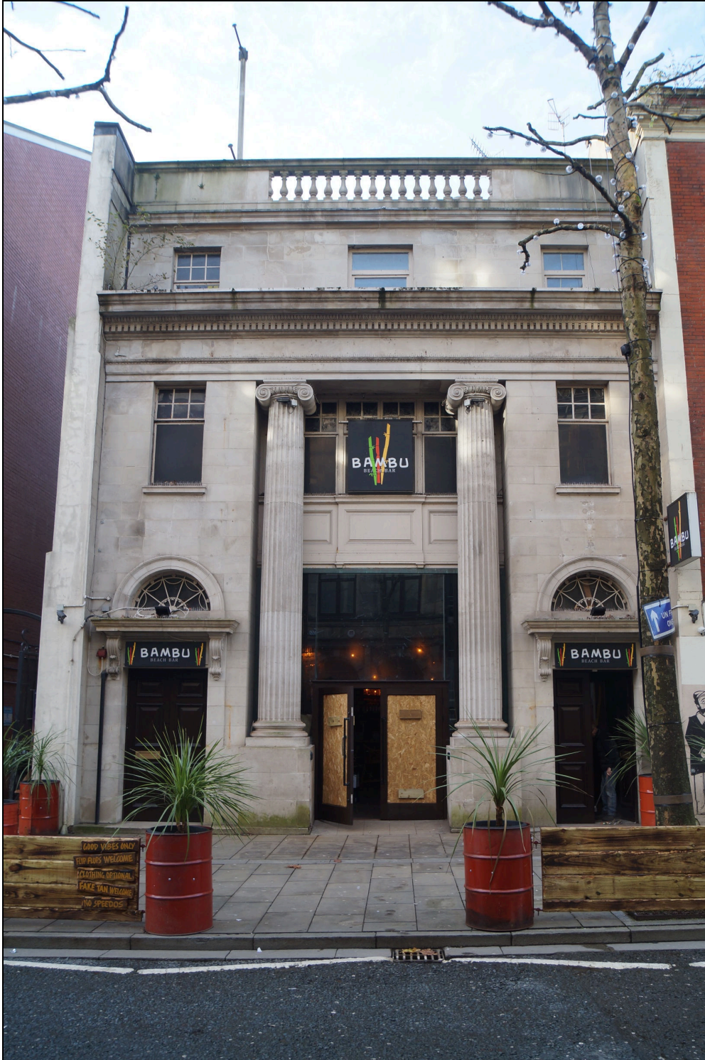
Plate 1: The façade of the former National Westminster Bank. The central door and windows were added c.2004 with planning permission. Apart from the Bambu signage, the rest of the façade is relatively unchanged. The doors to left and right are original features. Looking south-southwest.
