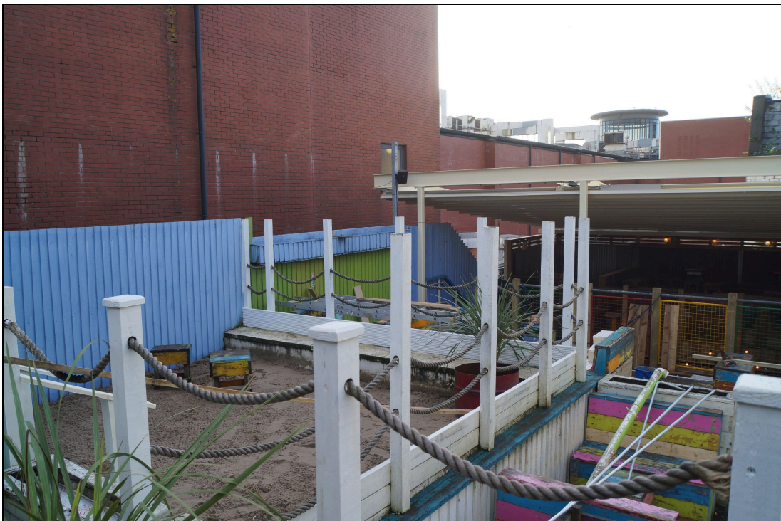
Figure 3: A partial view of the mezzanine floor and retractable canopy to the rear of the Bambu Beach Bar, showing modern development to the south of the property. The surrounding area has been transformed by new developments in the past two decades. Looking south.
