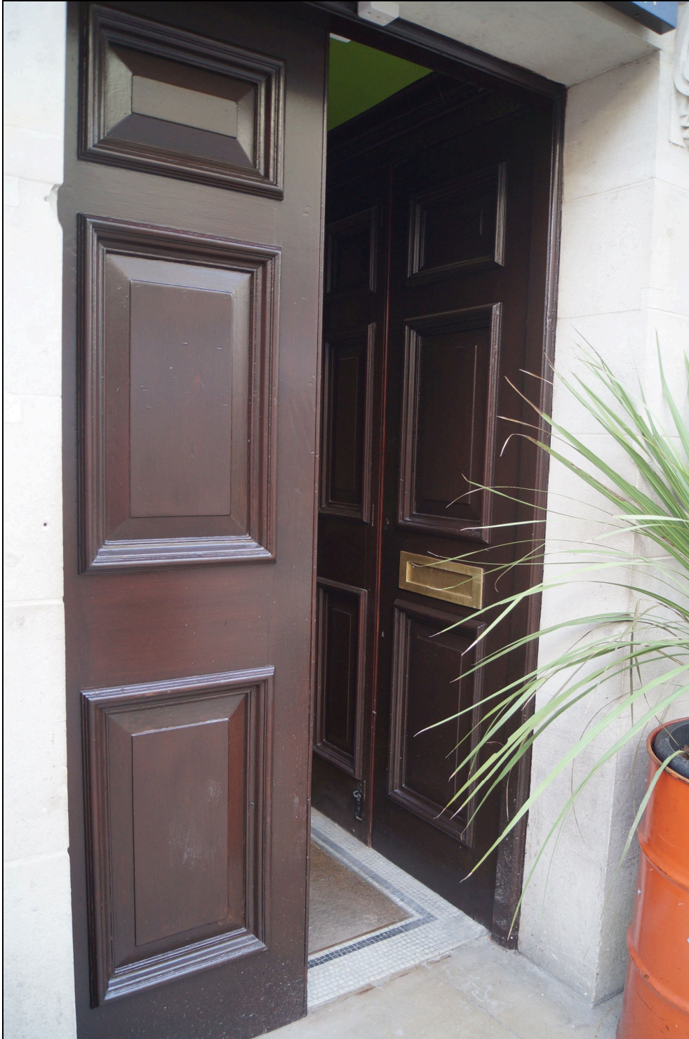
Plate 23: A view of the western doorway through the façade, the entrance to number 52, Wind Street originally. This shows how the doors were designed to open into a recess in order that they would be flush with the sides of the entrance porch when the bank was open. They are not affected by the development. Looking southwest.
