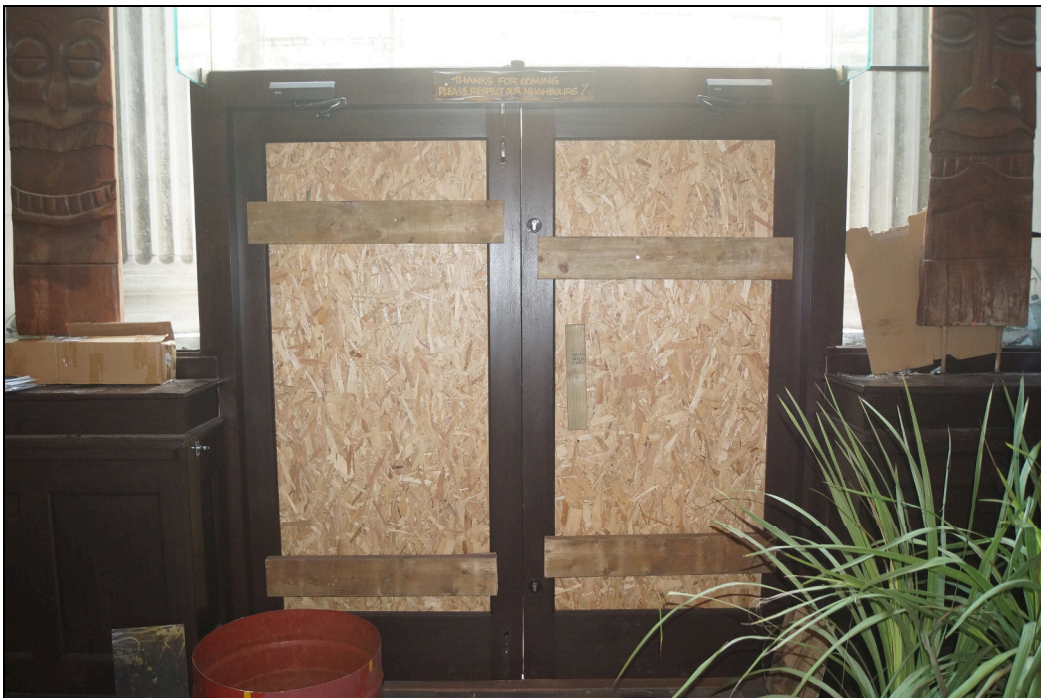
Plate 20: A view of the inside of the modern central doorway, which was added for Bar Riga after c.2004. This will be replaced by a more sympathetic hardwood, timber-framed door with glass panelling. Looking north-northeast.
