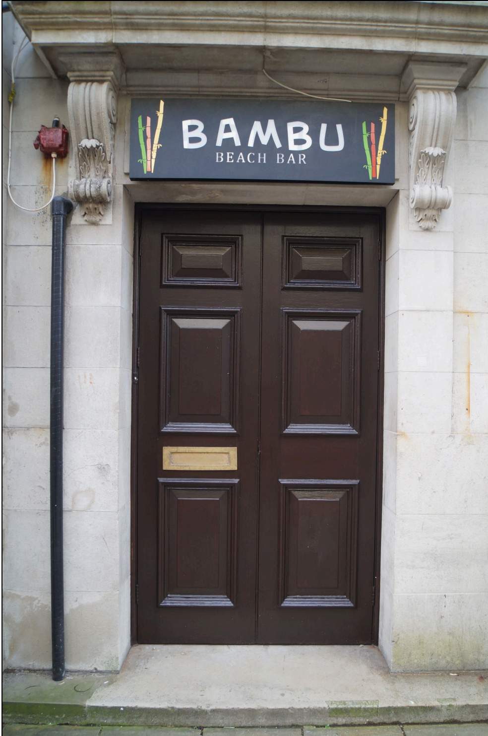
Plate 21: A view of the eastern doorway through the façade, the entrance to number 51, Wind Street originally. The door and door furniture are original. They are not affected by the development. Looking south-southwest.
