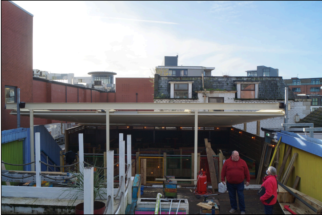
Plate 6: A view of the mezzanine floor and canopy. Looking south-southwest.
