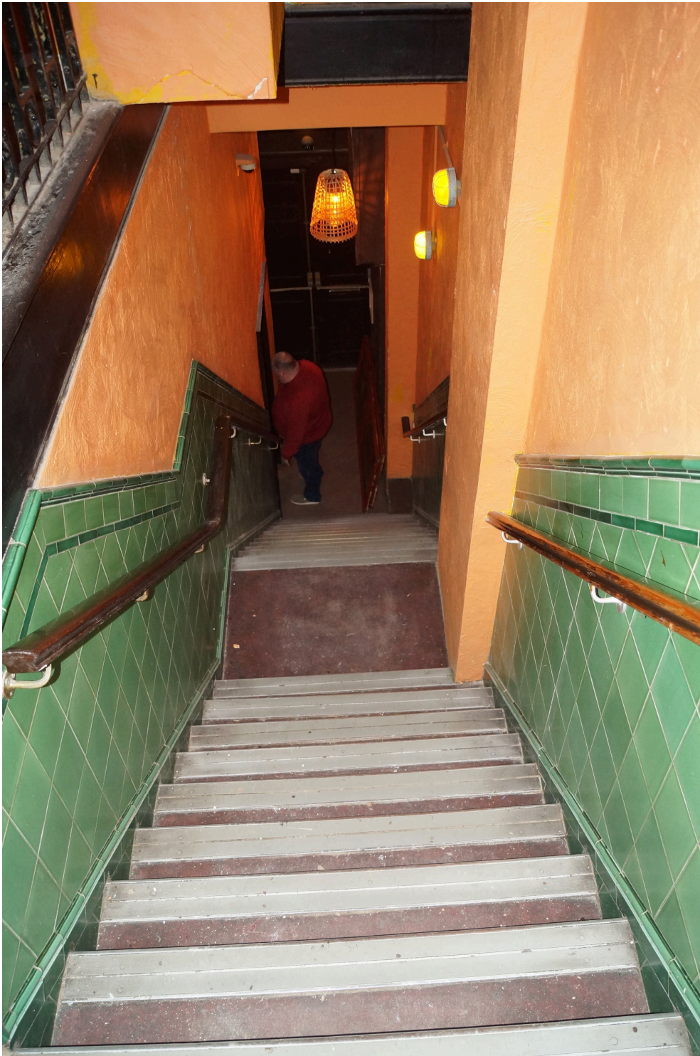
Plate 12: A view of down the stairs which lead from the ground floor entrance, No 51, on the eastern side of the building to the first floor offices. Looking north-northeast.
