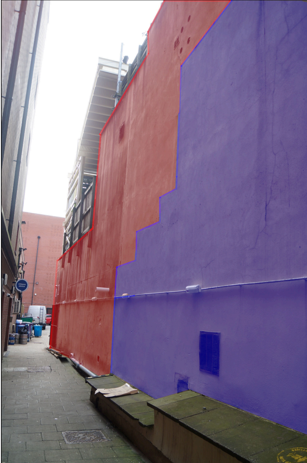
Plate 4: Another view of the eastern side of the former bank. The area shaded blue represents the approximate area of the original 1929 bank. The area shaded red shows the extension added c.1999 for conversion into a public house. The structure of the mezzanine floor and canopy is left unshaded and can be seen to be located on the later extension, not the original bank building. Looking southwest.
