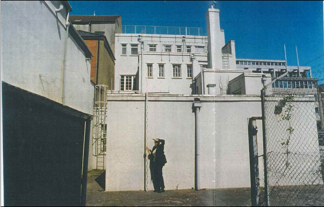
Figure 9: A view of the rear of the bank taken c.1997 by the RCAHMW showing the southern wall of the bank strong room at ground level, which was removed by the early 21 st century. Looking north-northeast. (Source National Monuments Record, RC20-0672 LM OAI). © Crown copyright: RCAHMW
