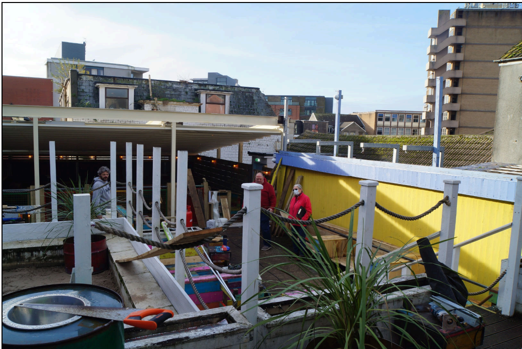
Plate 7: A view of the existing roof terrace with the mezzanine floor and canopy beyond. Note the modern development in the distance. Looking southwest.
