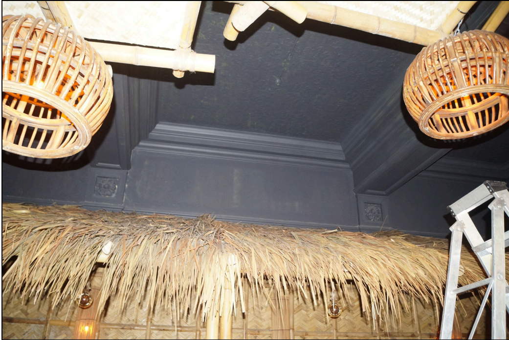
Plate 19: A view of the rosettes in the coffered ceiling in the former banking hall on the ground floor. These have been retained in the building and are not affected by the current development. Looking west-northwest.
