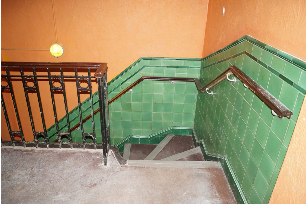
Plate 10: A view of the top of the stairs which lead from the ground floor entrance, No, 51, on the eastern side of the building to the first floor offices. The tiles and balustrade are original, the handrail is a later addition. Looking east-southeast. This is not the staircase to be converted to a fire escape.
