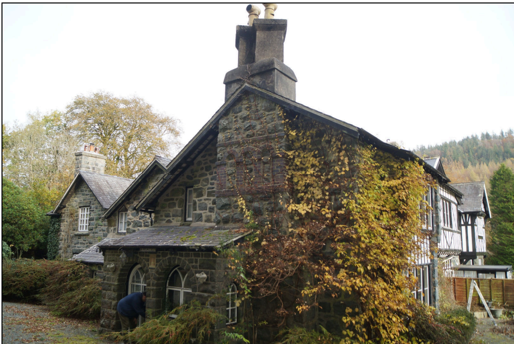
Plate 21: GGN2019_021 – A view of Gelligemlyn in 2019. The former mansion is now divided into four parts. The section to the left is the side
