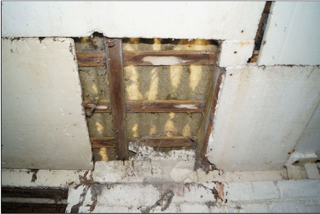
Plate 7: GGN2019_007 – A view through the ceiling showing the underside of the corrugated asbestos sheeting on the roof of the "stable" along the northern side of the building. Looking south.
