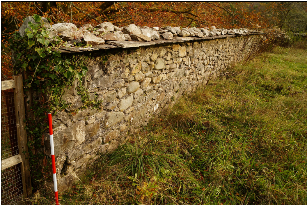
Plate 33: GGN2019_033 – a more detailed view of the eastern wall of the walled garden, showing the quality of its built and the slate copings still in situ. Looking southeast.
