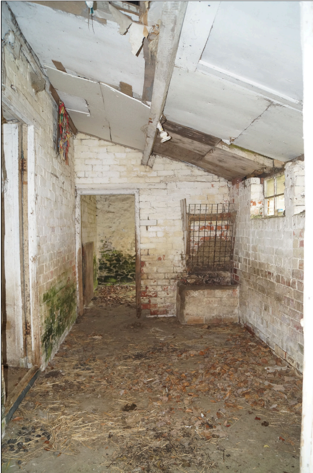
Plate 9: GGN2019_009 – A view of the inside of the "stable". The feeder to the right of centre has been added in after the building had ceased being used as a glasshouse and potting shed and the stable had been created inside its northern section. Looking west.
