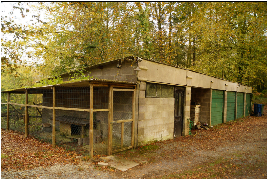
Plate 26: GGN2019_026 – A view of the later 20 th century garage range, which has no historical association with the former glasshouse. It does not appear on an aerial photograph of 1962 (Central Register of Aerial Photography for Wales, 6208 RAF58_5165/F22/0100) but is shown on an
