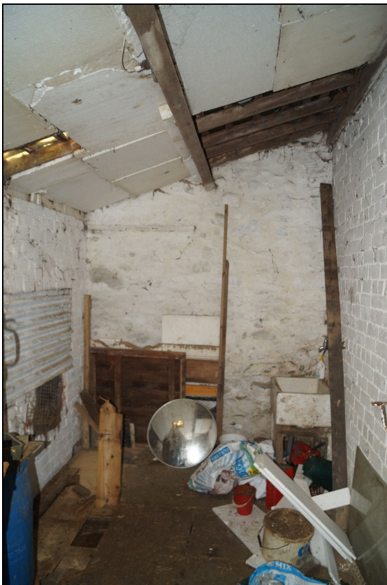
Plate 7: GGN2019_007 – A view through the ceiling showing the underside of the corrugated asbestos sheeting on the roof of the "stable" along the northern side of the building. Looking south.
