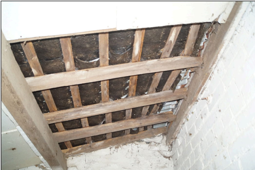
Plate 6: GGN2019_006 – A view through the ceiling showing part of the original slate roof inside the "stable" at the northern side of the building. This may originally been the potting shed. Looking east.
