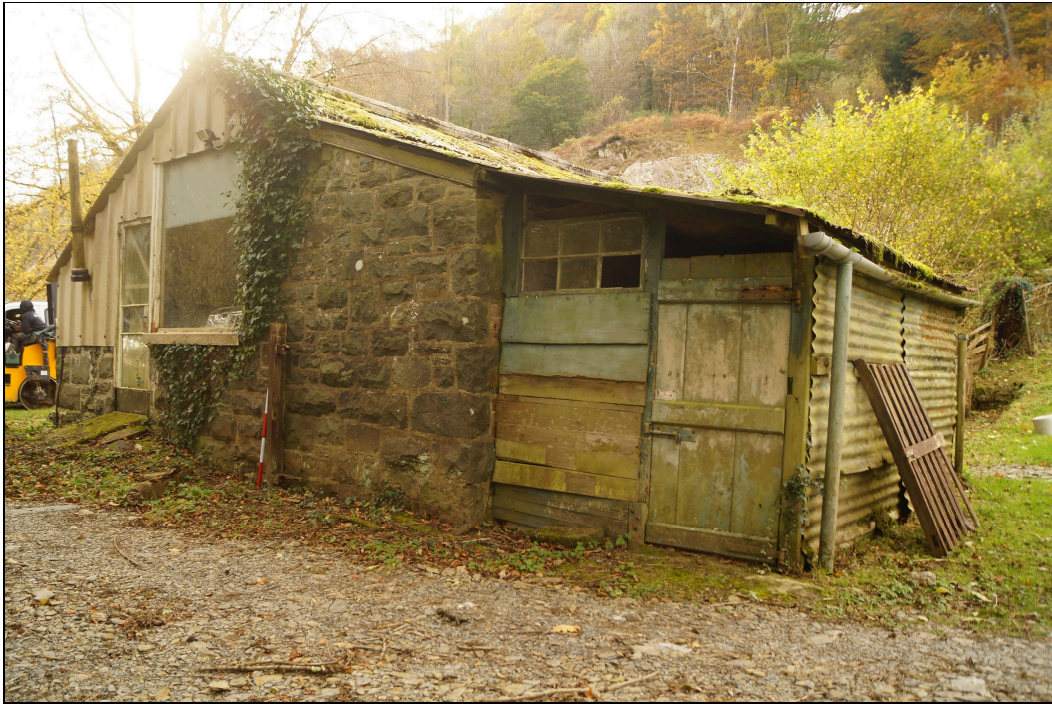
Plate 18: GGN2019_018 – An external view of the building. The crude extension seen right of centre does not appear to be part of the original glasshouse and potting shed. It first appears on an aerial photograph of 1962 (Central Register of Aerial Photography for Wales, 6208 RAF58_5165/F22/0100), being absent from aerial photographs dating to the 1940s. Looking southwest.
