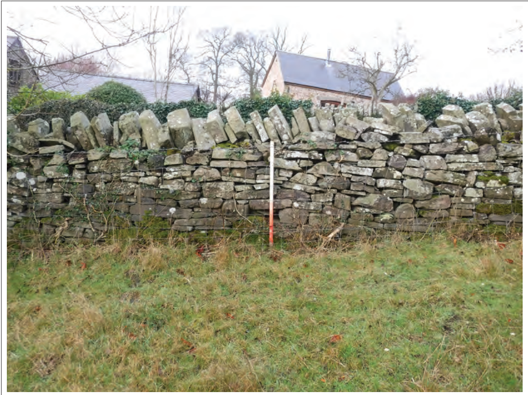
Plate 5. Western site boundary drystone wall, looking west.
