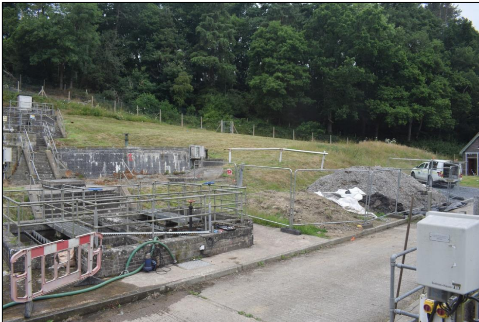
Fig. 7 Sewage treatment works viewed from the south-east, the grassed area to the rear of shot is the proposed site for additional treatment tanks (Fig. 2, 1) CPAT Photo 5001-002
